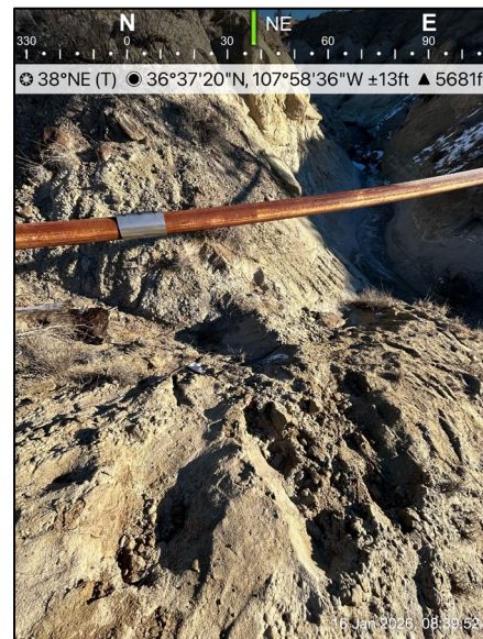
Photograph: 2 Date: 1/28/2026 Description: Repaired initial leak View: Northeast
