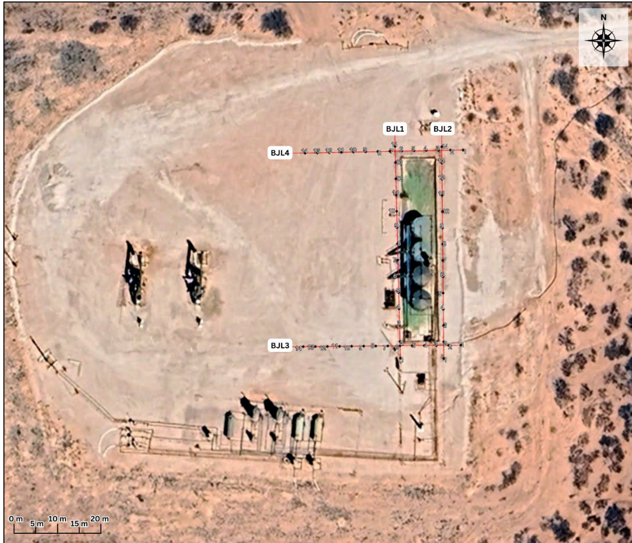
Figure 1. Aerial view of the Beetle Juice 19 Fed 3H site, illustrating the position of each electrode used during the electrical resistivity surveys.
