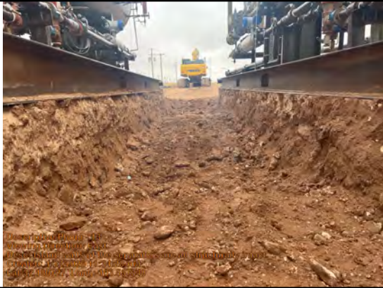
Island walls of the separators are all structurally intact.
