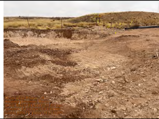
BS25- 24 and 25 at 2ft bgs.
