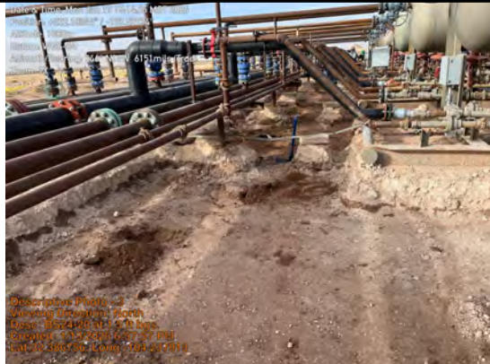
BS24-20 at 1.5 ft bgs.
