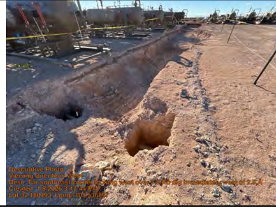
Far southeast corner looking west over 4' dig immediately west of 2.5' dig. Hydro vac'd underground flow lines seen.
