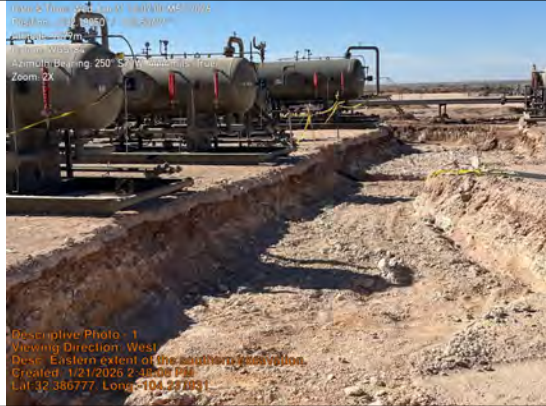
Eastern extent of the southern excavation.
