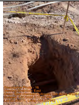
Spot checked hydrovac line along WS25-20.
