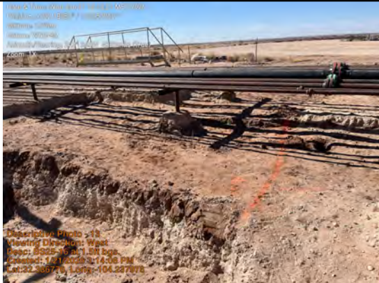
BS25-16 at 1.5ft bgs.
