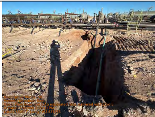
Flow lines and 3' excavated area, exposed via hydro vac
