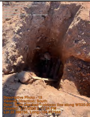
Spot checked hydrovac line along WS25-20.
