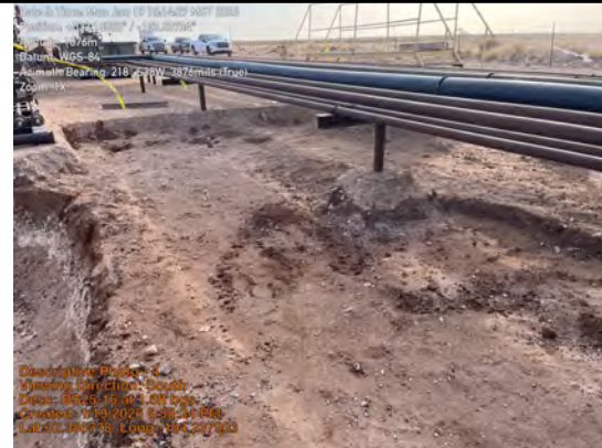
BS25-16 at 1.5ft bgs.
