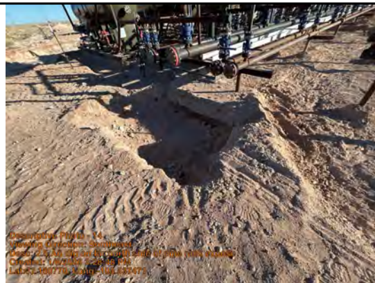
2.5' dig on far north side of pipe rack exposed
