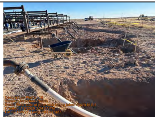
West side of pipe rack being taken down to 0.5'
