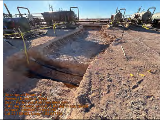
Hydro vac'd flow lines seen. 3' dig extends west to 4' dig in southwest corner.
