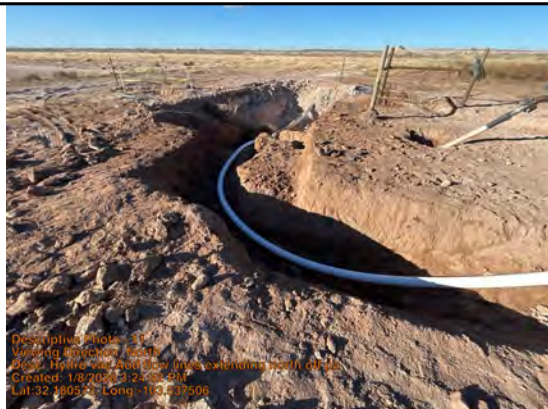
Hydro vac'd flow lines extending north off pad.
