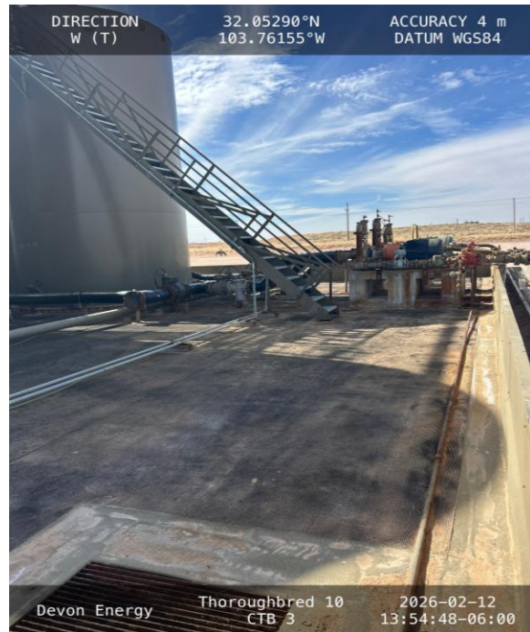
Photo 4 View of northside of secondary containment towards west.
