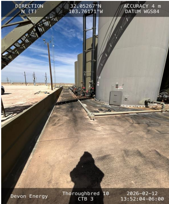
Photo 9 View of west side secondary containment towards north.
