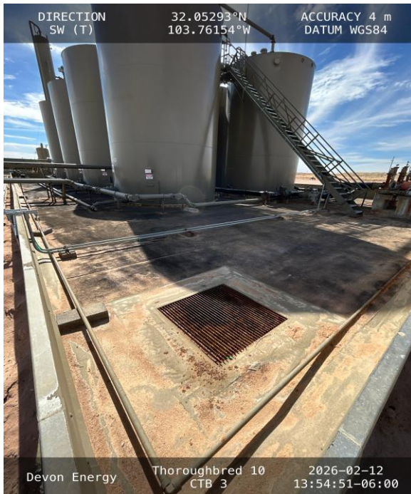
Photo 3 View of northeast corner of secondary containment.
