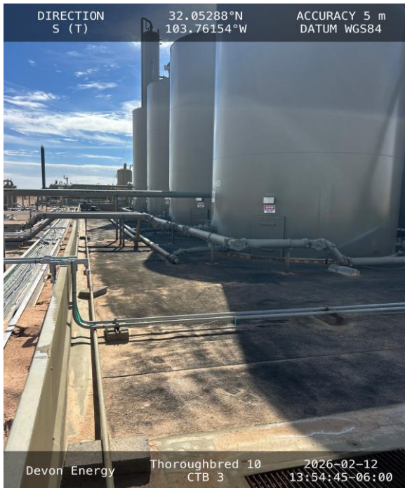
Photo 5 View of east side secondary containment towards south.
