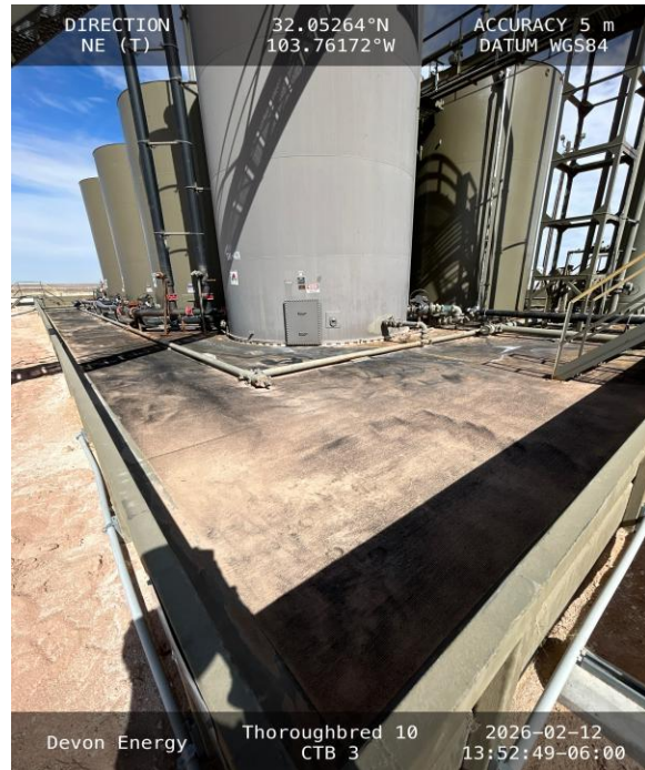
Photo 6 View of southwest corner of secondary containment.
