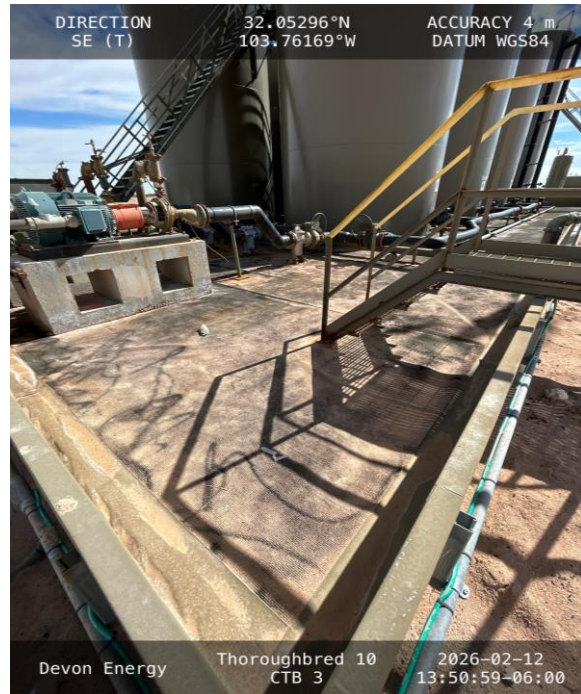
Photo 12 View of northwest corner of secondary containment.
