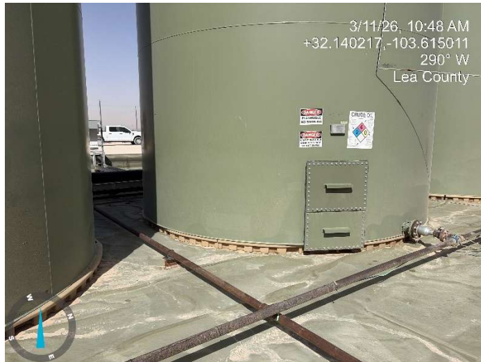
Photograph: 9 Date: 3/11/2026 Description: View of competent liner during inspection activities
