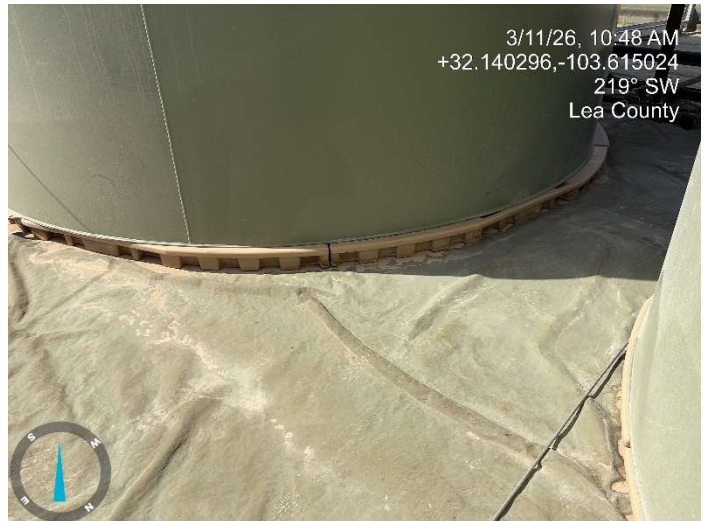
Photograph: 10 Date: 3/11/2026 Description: View of competent liner during inspection activities
