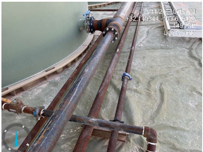
Photograph: 4 Date: 3/11/2026 Description: View of competent liner during inspection activities
