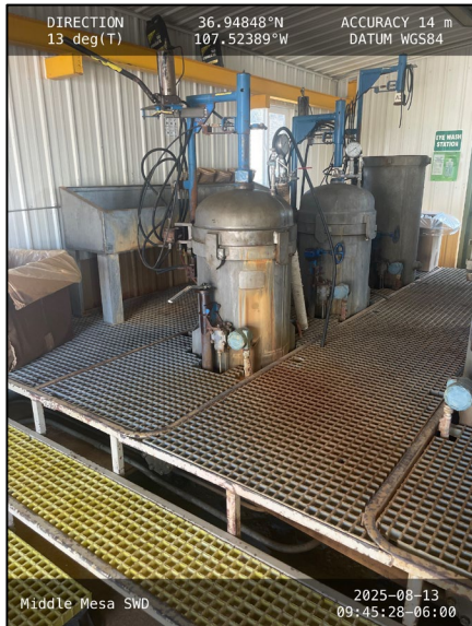
Photograph: 1 Date: 8/13/2025 Description: Release source from the A1 filter pot View: North
