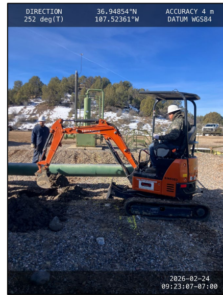
Photograph: 8 Date: 2/24/2026 Description: Additional sampling at pothole location PH01 View: West
