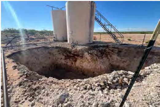
View to SE of W TB excavation (8/7/25).
