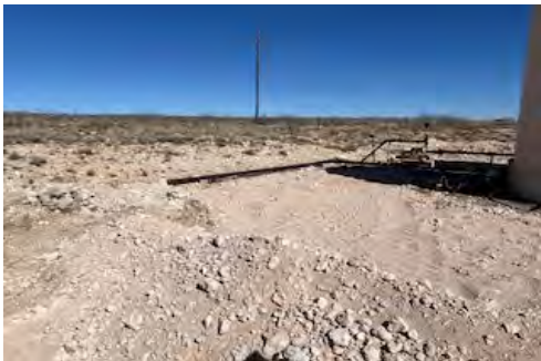
View to SE of backfilled excavations at battery (nSAP0225252743).
