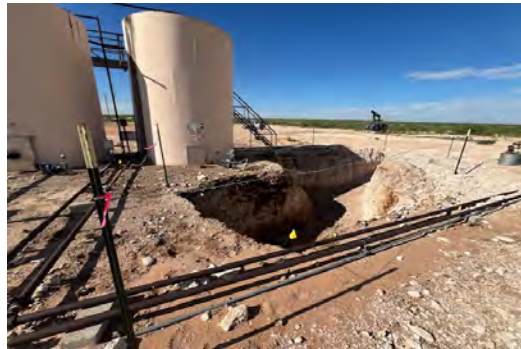
View to SW of E TB excavation (8/7/25).
