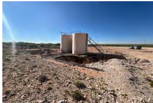
View to SE of TB excavations (8/7/25).
