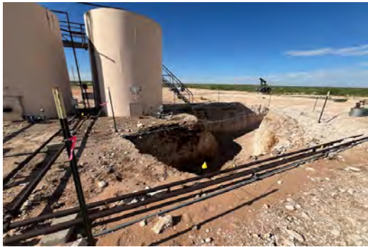
View to SW of E TB excavation (8/7/25).
