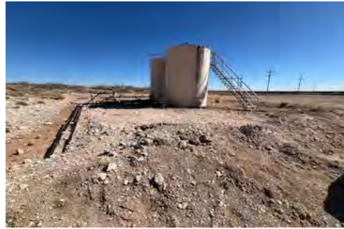
View to E of backfilled excavations at battery (nSAP0225252743).
