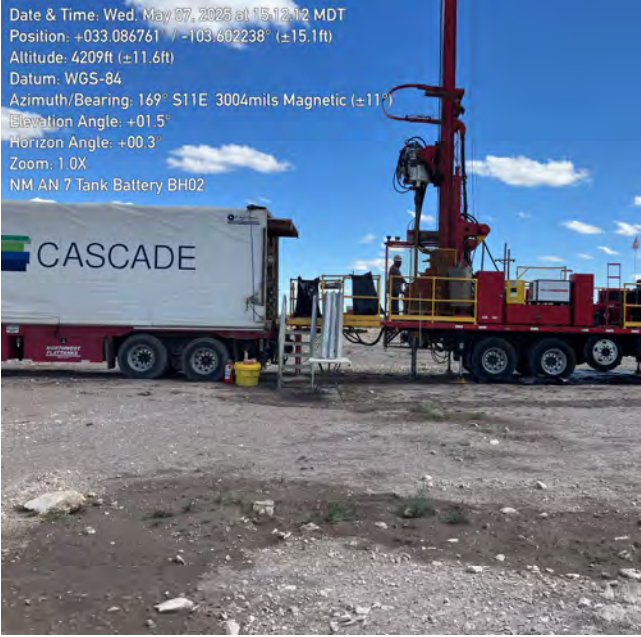
Photograph 1 Date: 05/07/2025 Description: Southeastern view of delineation activities.
