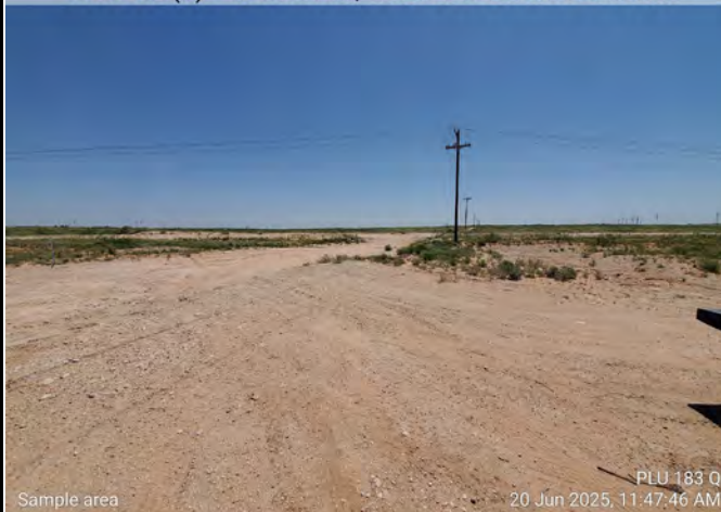
Photograph: 1 Date: 6/20/2025 Description: Backfill activities View: Northeast
