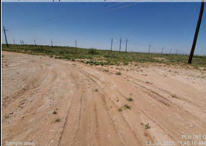
Photograph: 3 Date: 6/20/2025 Description: Backfill activities View: Southwest
