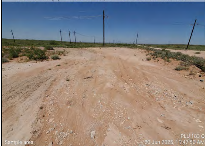
Photograph: 2 Date: 6/20/2025 Description: Backfill activities View: Southwest
