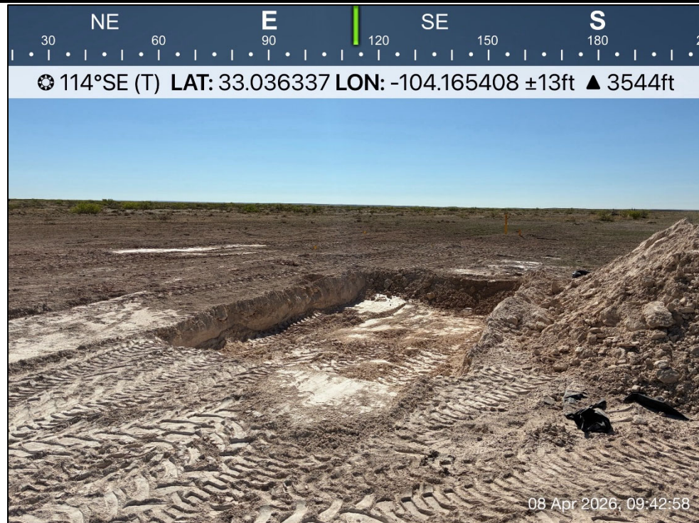
PHOTO 6: Southeastern view of excavation extent. 4/8/2026
