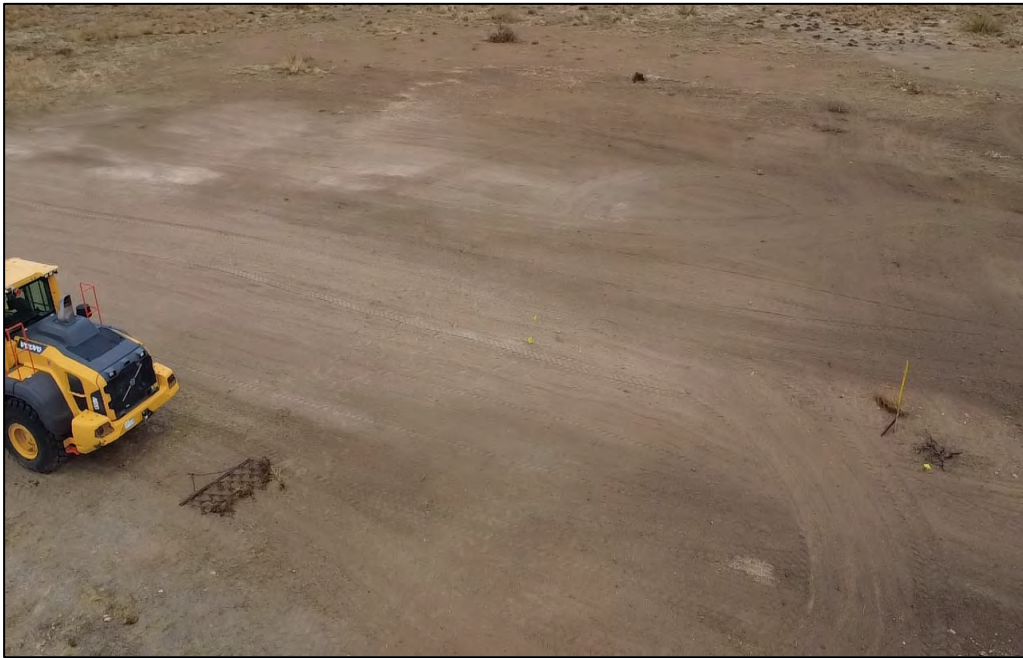
PHOTO 13: Northwestern view during restoration activities. 11/20/2025
