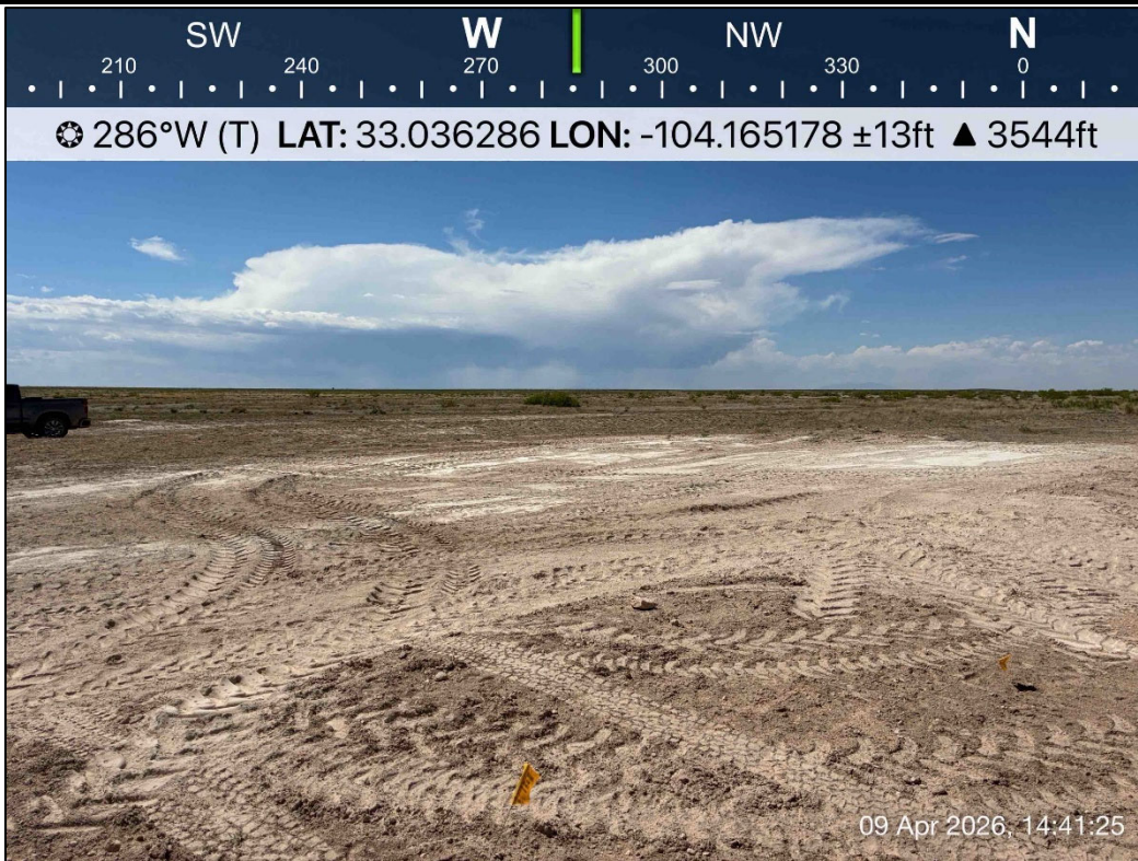
PHOTO 8: Northwestern view following restoration activities. 4/9/2026
