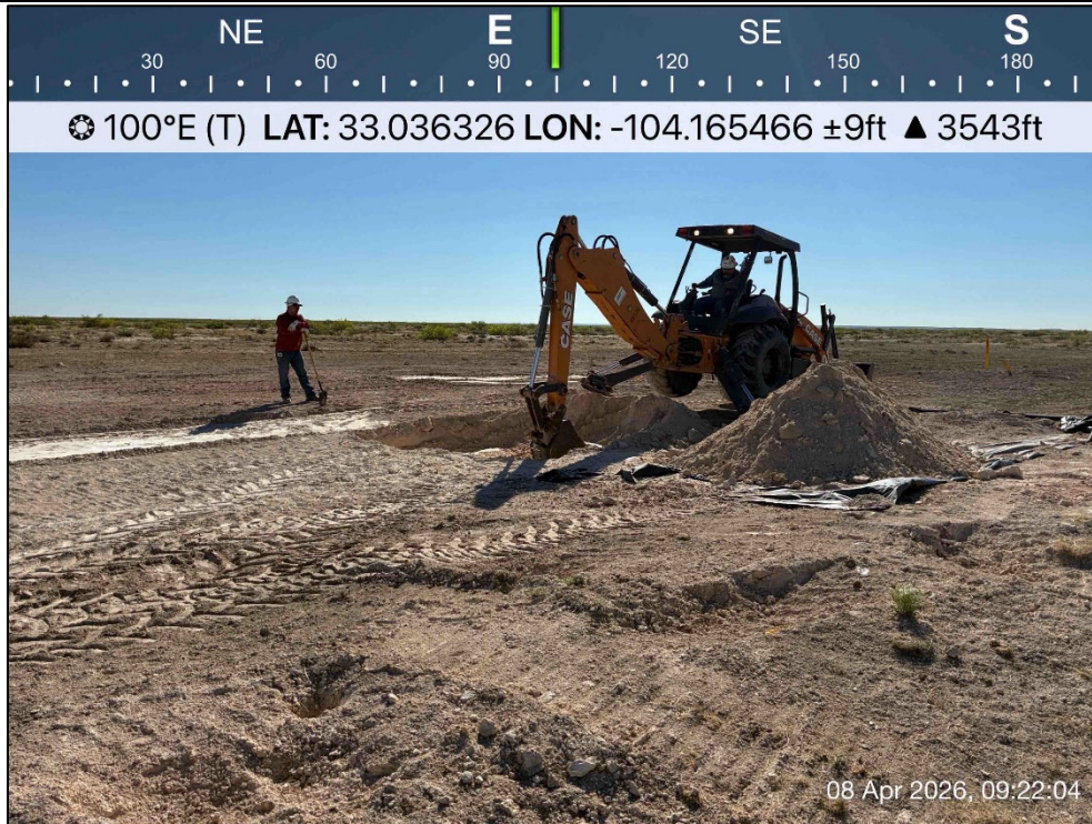
PHOTO 5: Southeastern view during excavation activities. 4/8/2026
