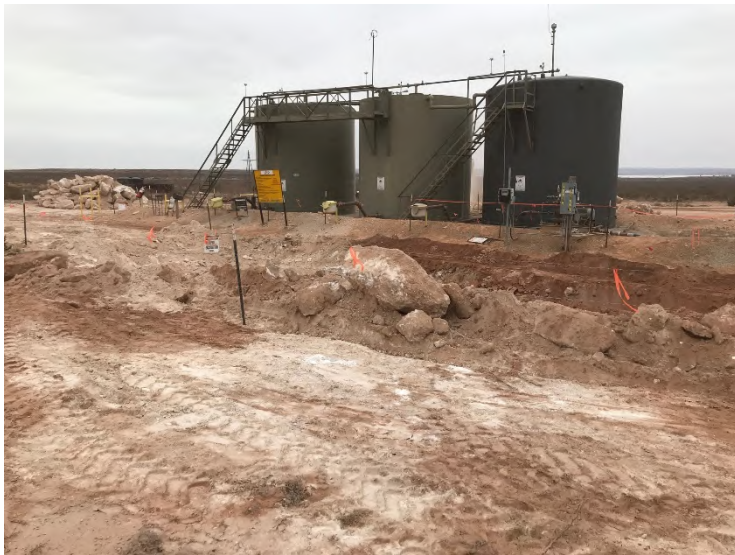
Photograph 3: View of tank battery and excavation - looking north west.
