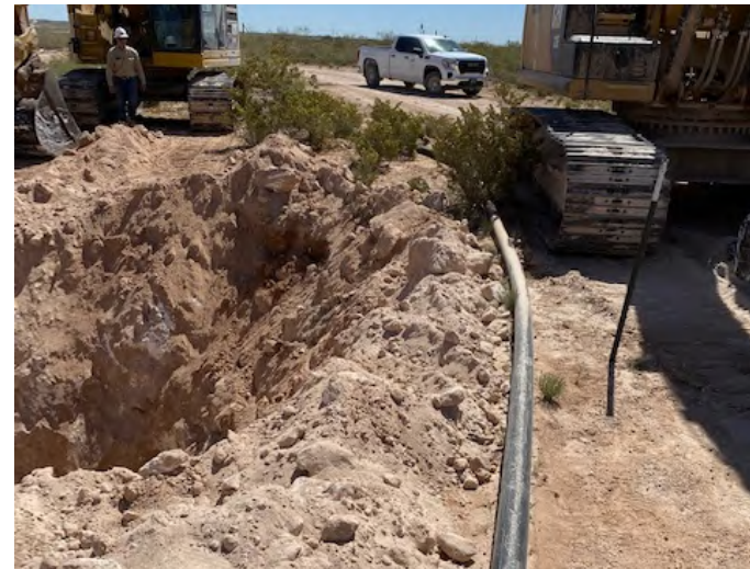
Photograph 4: View of open excavation – looking east.
