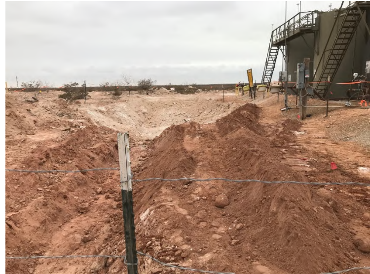
Photograph 2: View of pad and excavation – looking west
