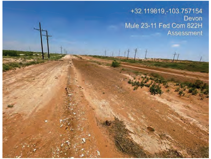
South side looking north
