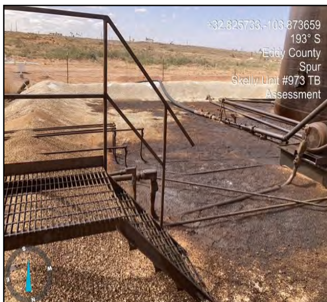
Photograph taken during initial assessment facing south.
