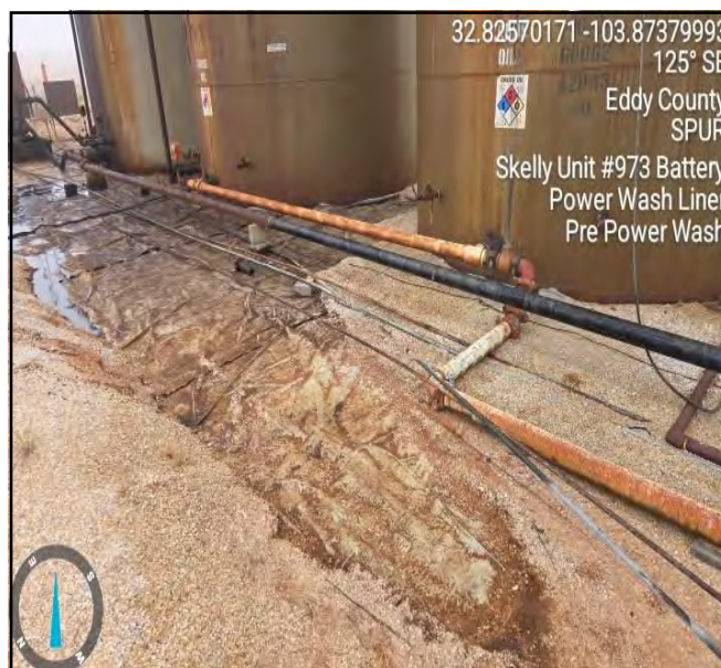
Photograph taken pre powerwash process facing southeast.
