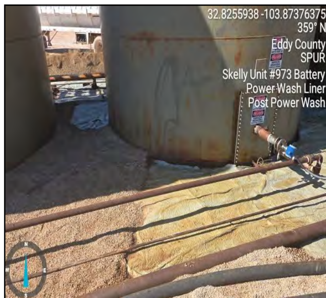
Photograph taken post powerwash facing north.
