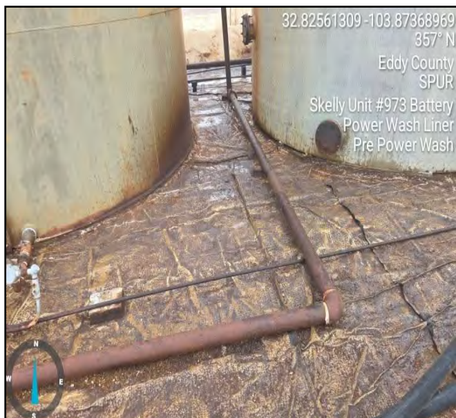
Photograph taken pre powerwash process facing north.
