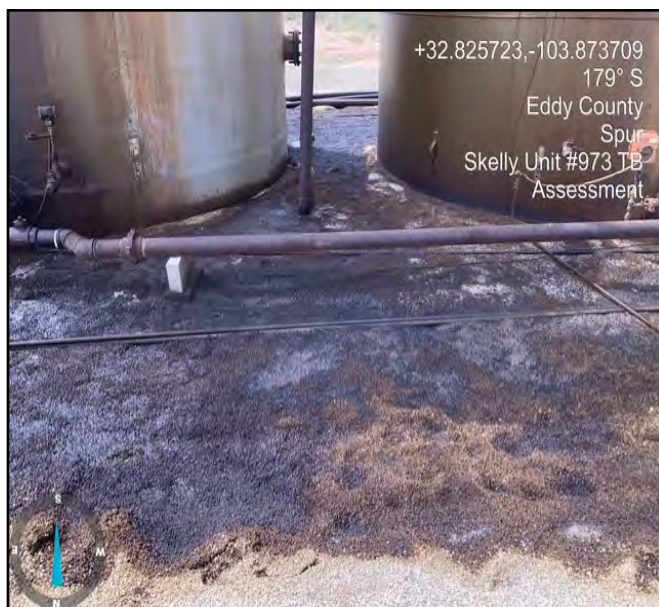
Photograph taken during initial assessment facing south.
