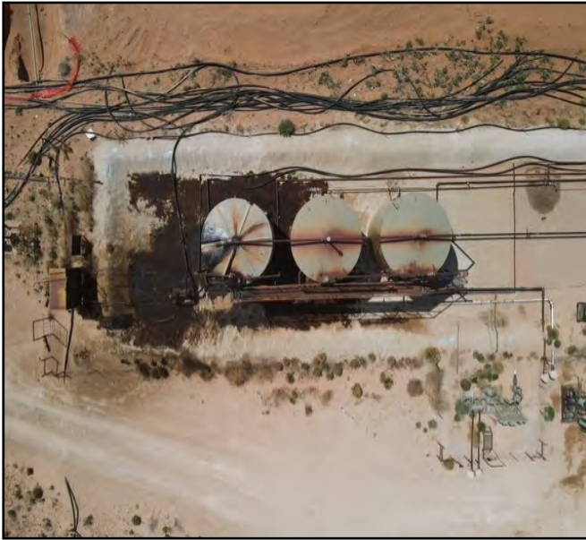
Pre aerial photos taken of location.
