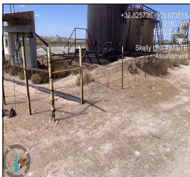
Photograph taken during initial assessment facing southwest.
