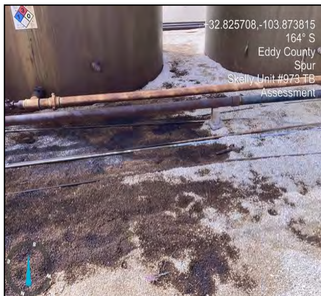
Photograph taken during initial assessment facing south.
