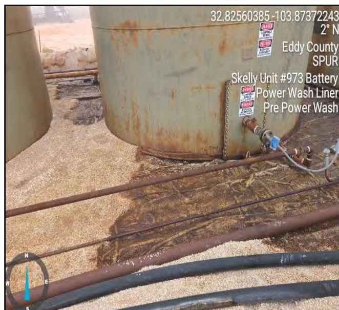
Photograph taken pre powerwash process facing north.
