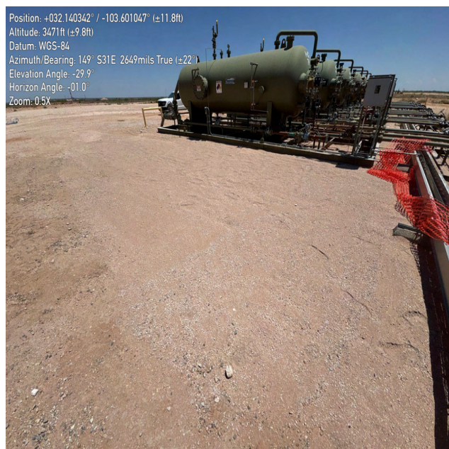
Photograph 16 Date: 05/27/2026 Description: Southeastern view of backfill activities.
