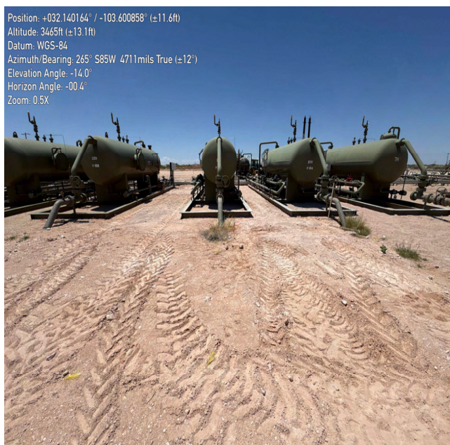
Photograph 15 Date: 05/27/2026 Description: Southwestern view of backfill activities.
