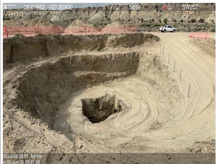
Photograph: 12 Description: Final excavation extent View: Southwest Date: 6/2/2026
