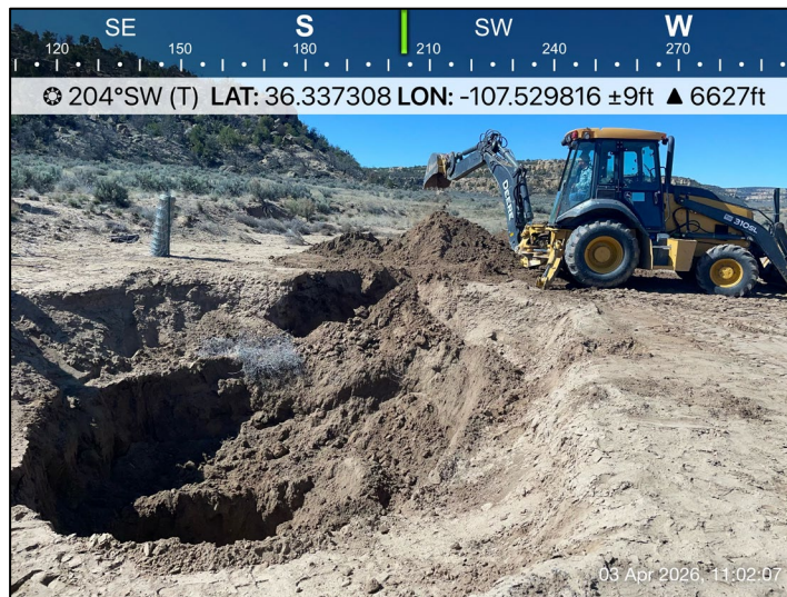
Photograph: 2 Description: Excavation activities.
