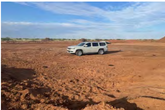
View to SW of excavation.
