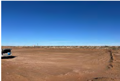
View to N of E end of Section 1 excavation.
