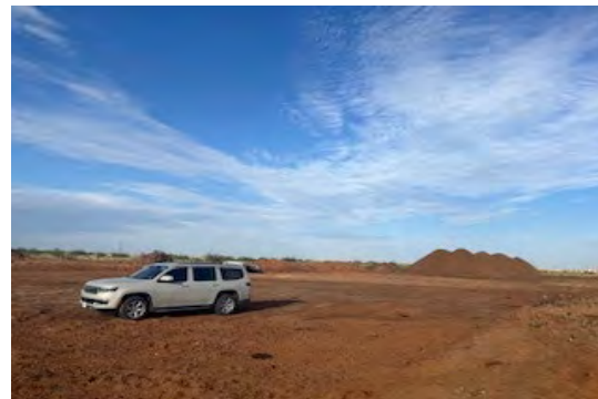
View to SW of excavation and treated soil.
