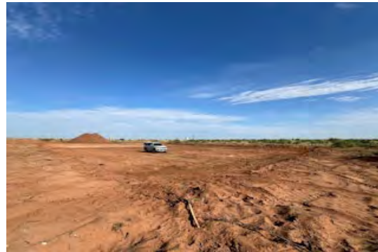
View to NW from SE corner of excavation.
