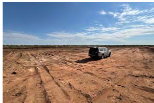
View to E from SW side of excavation.
