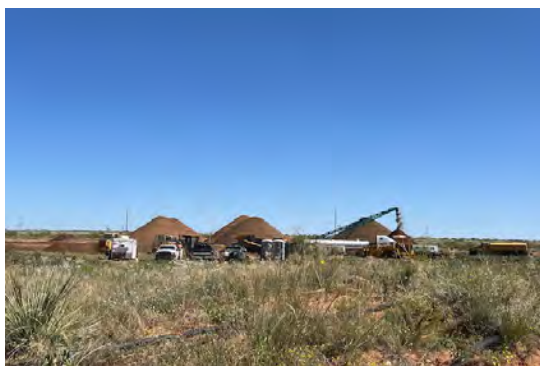
View to S of treated soil piles (7/30/25).
