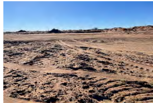
View to N of W part of Section 1 excavation.
