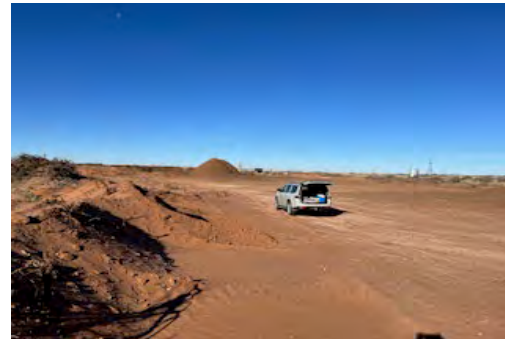
View to W of S side of Section 1 excavation.
