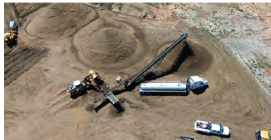
Aerial view of treated soil piles (7/25/25).
