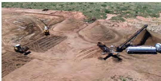
Aerial view of treated soil piles (7/25/25).
