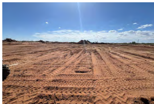
View to W of excavation and treated soil piles (7/30/25).
