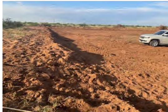
View to E of N side of excavation.
