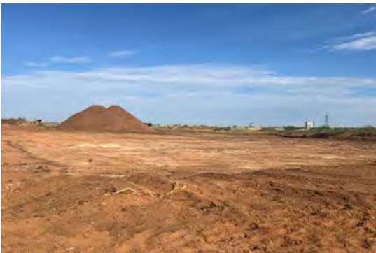
View to NW from SE corner of excavation at 3' depth.
