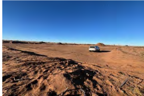
View to SW of Section 1 excavation.
