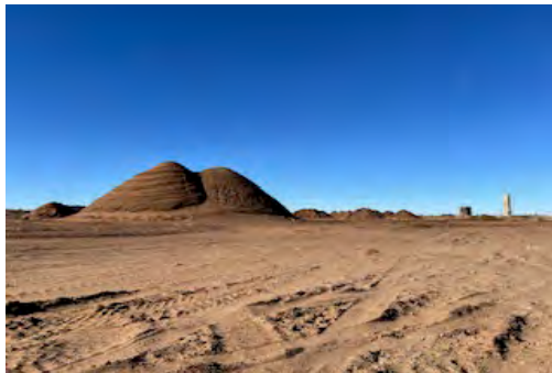
View to W of W end of Section 1 excavation.
