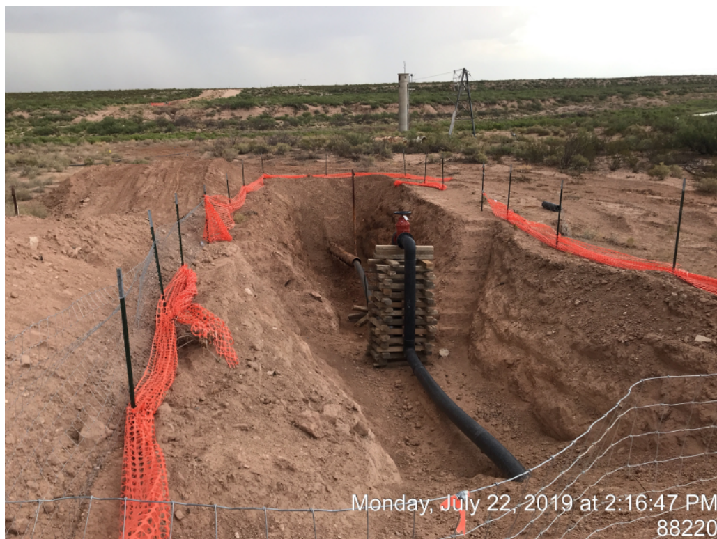
West side of river vent pipe repair
