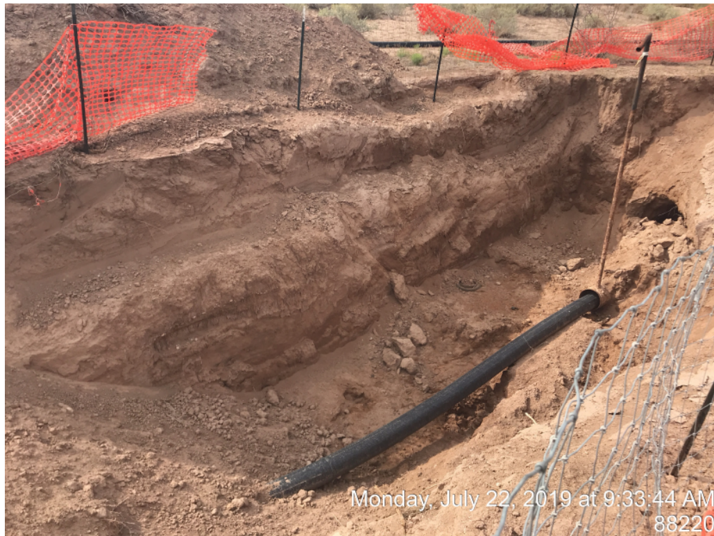
East side of the river vent pipe
