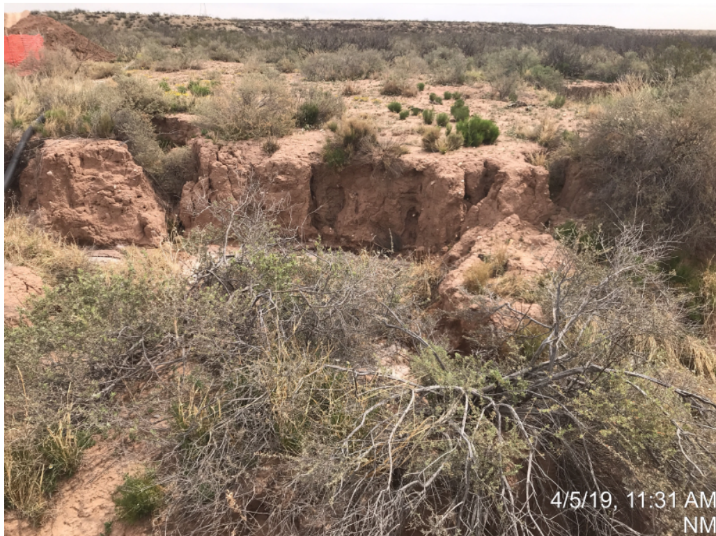
East side of the river looking east over wash out
