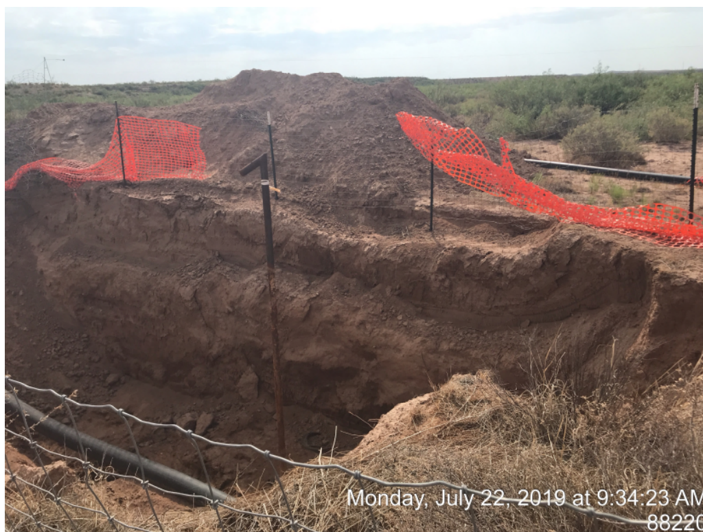
East side of the river vent pipe
