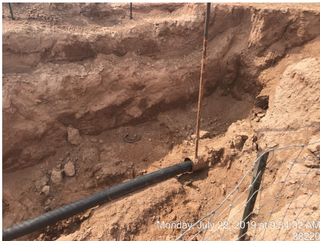
East side of the river vent pipe
