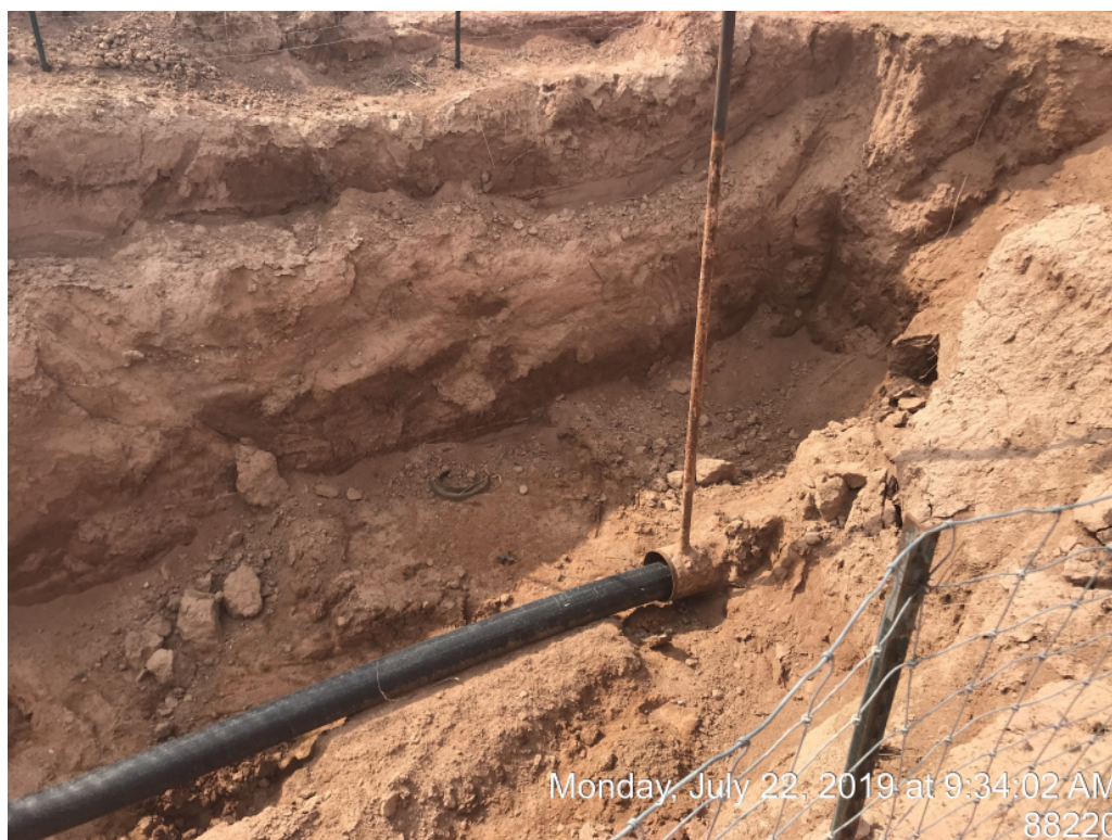
East side of the river vent pipe
