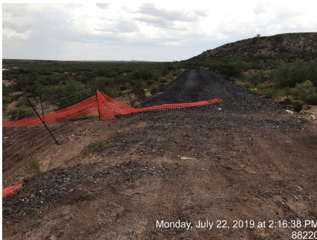
West side of the river looking south, Railroad tracks
