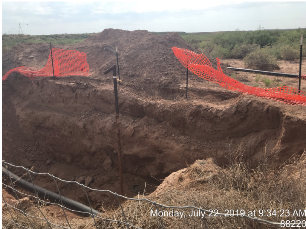
East side of the river vent pipe
