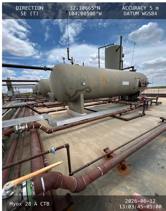
Photo 5 View of containment facing southeast.
