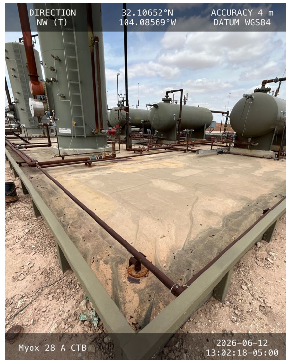
Photo 2 View of southeast corner of east side of containment area facing northwest.
