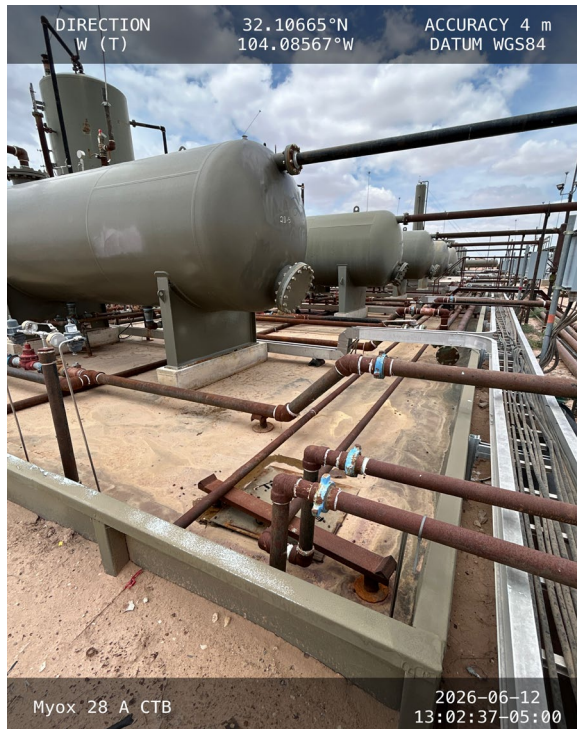
Photo 3 View of east side of containment area facing west.
