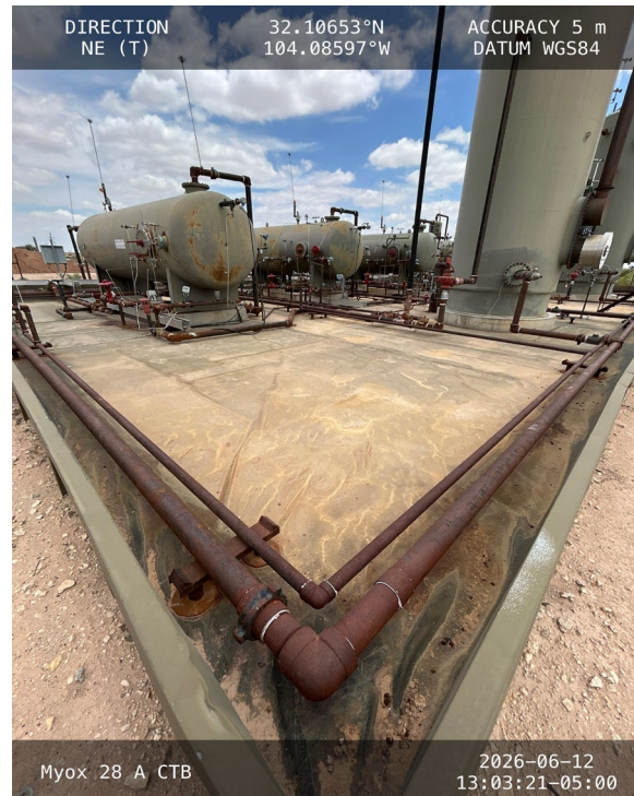
Photo 4 View of southwest corner of east side of containment area facing northeast.
