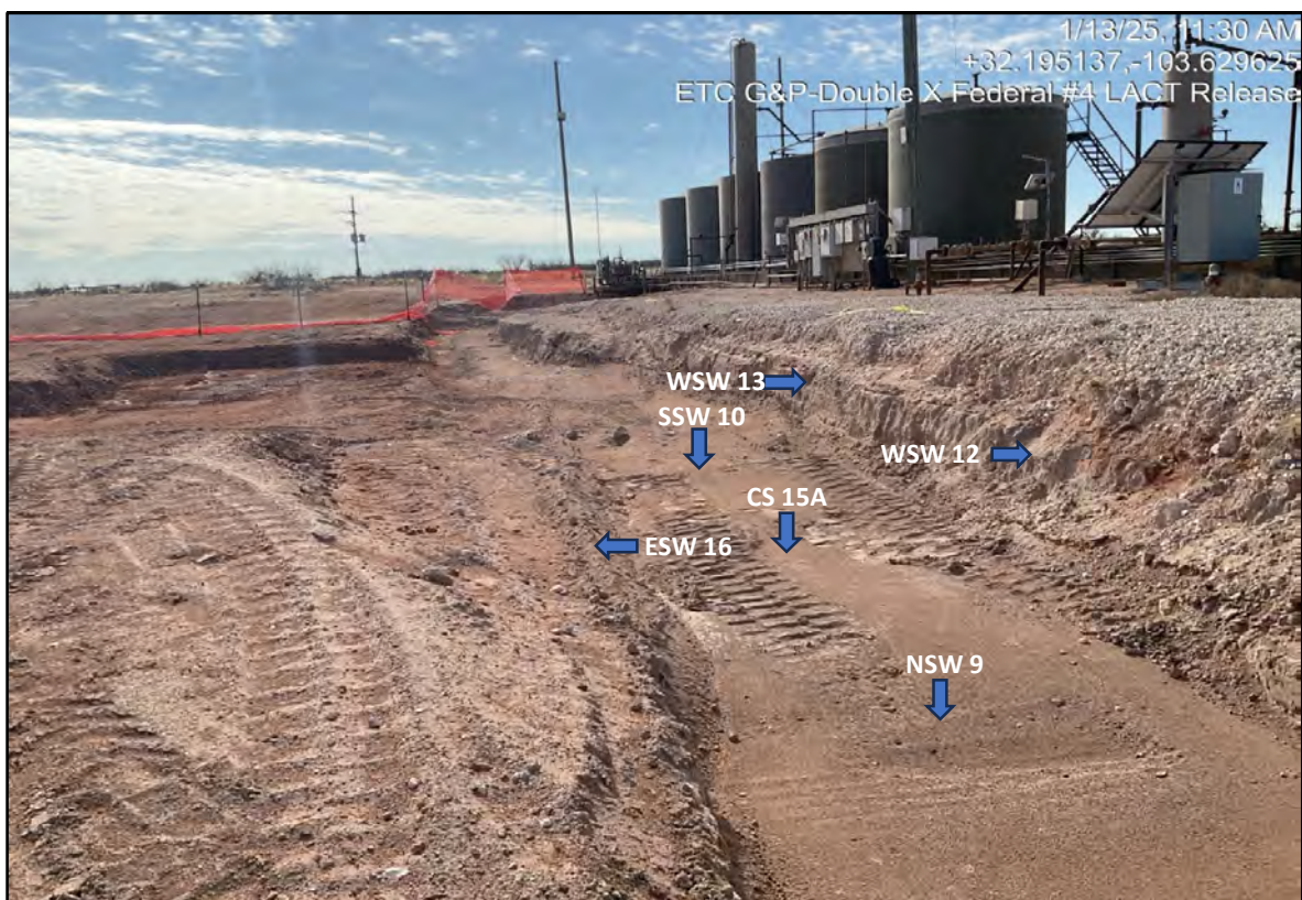
View South - Remediation activities (i.e., excavation and stockpiling) in progress. Sample locations CS 15A, NSW 9, WSW 12, WSW 13, ESW 16, and SSW 10.
