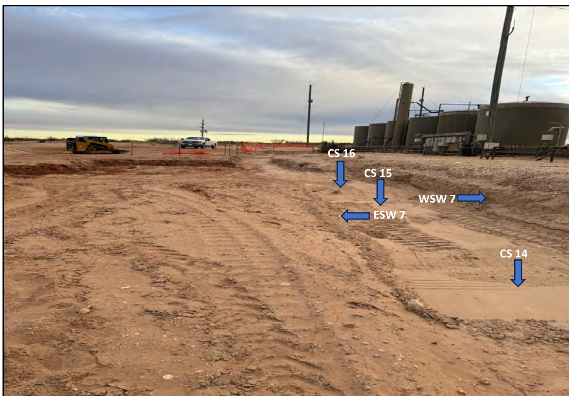
View South - Remediation activities (i.e., excavation and stockpiling) in progress. Sample locations CS 14 thru CS 16, WSW 7, and ESW 7.
