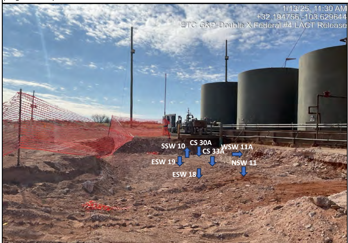
View South - Remediation activities (i.e., excavation and stockpiling) in progress. Sample locations CS 30A, CS 33A, NSW 11, WSW 11A, ESW 18, ESW 19, and SSW 10.
