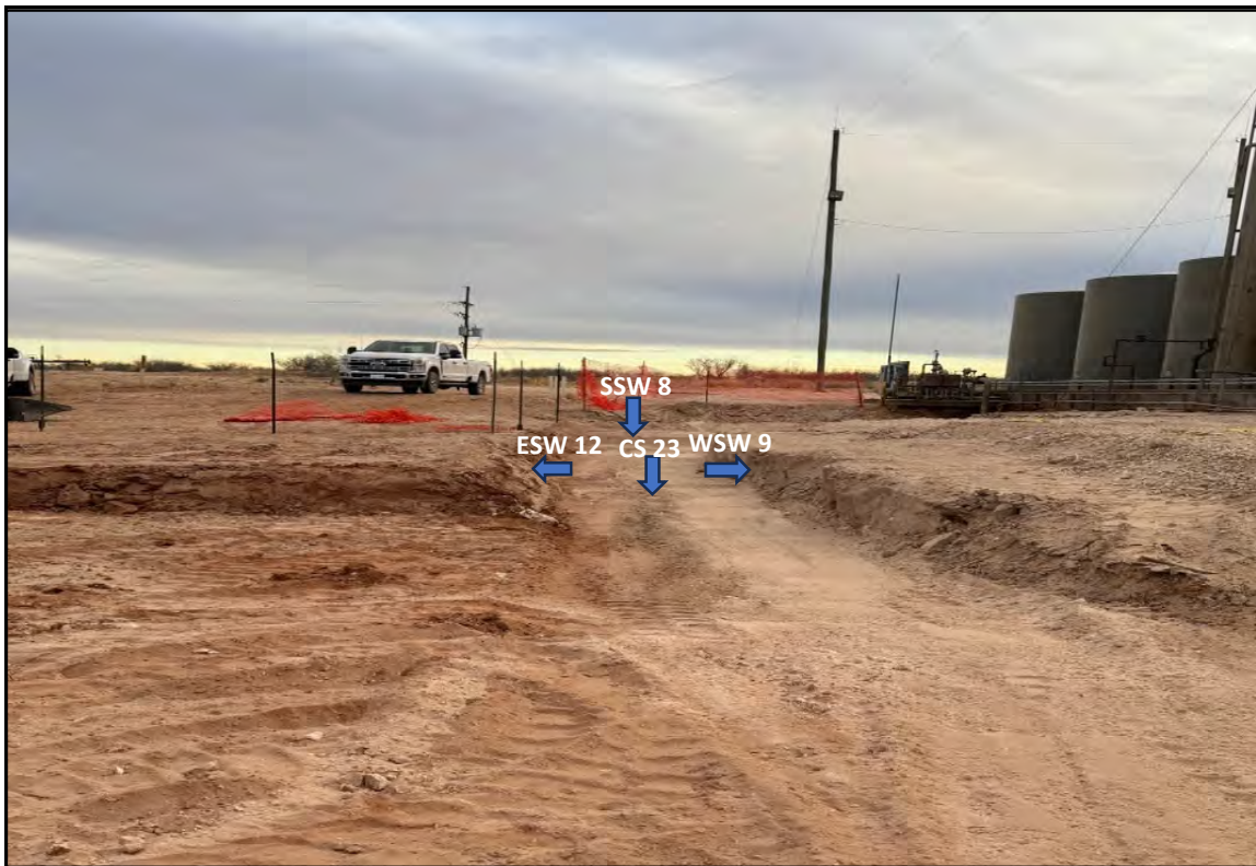
View South - Remediation activities (i.e., excavation and stockpiling) in progress. Sample locations CS 23, WSW 9, ESW 12, and SSW 8.
