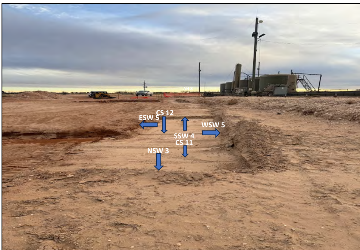
View South - Remediation activities (i.e., excavation and stockpiling) in progress. Sample locations CS 11, CS 12, NSW 3, WSW 5, ESW 5, and SSW 4.
