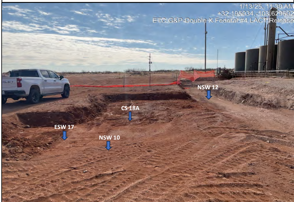
View South - Remediation activities (i.e., excavation and stockpiling) in progress. Sample locations CS 18A, NSW 10, NSW 12, and ESW 17.
