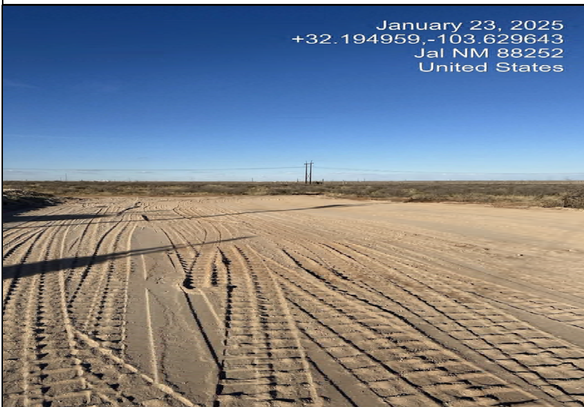
View North - Remediation activities (i.e., backfilling) complete.
