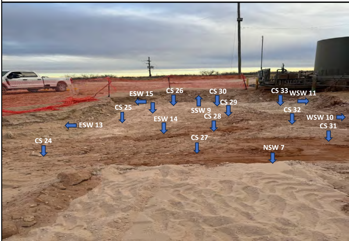
View South - Remediation activities (i.e., excavation and stockpiling) in progress. Sample locations CS 24 thru CS 33, NSW 7, WSW 10, WSW 11, ESW 13 thru ESW 15, and SSW 9.
