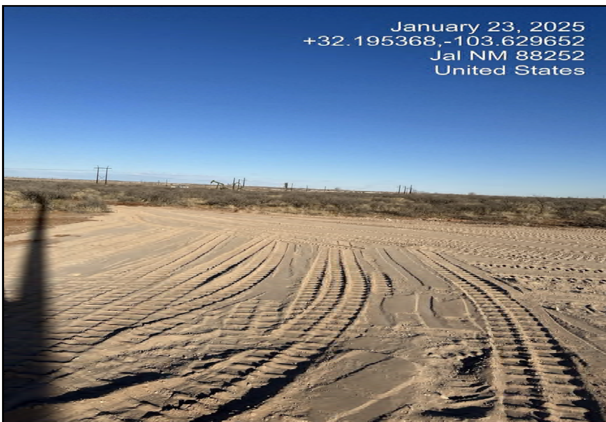
View East - Remediation activities (i.e., backfilling) complete.
