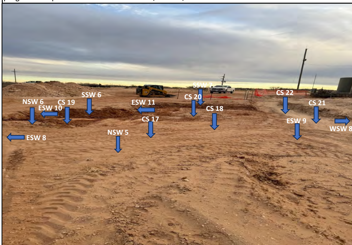
View South - Remediation activities (i.e., excavation and stockpiling) in progress. Sample locations CS 17 thru CS 22, NSW 5, NSW 6, WSW 8, ESW 8 thru ESW11, SSW 6, and SSW 7.
