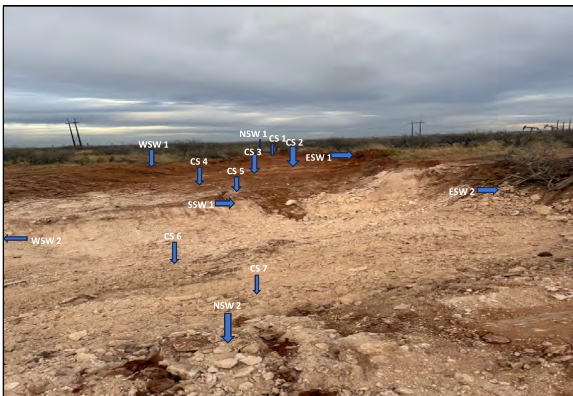
View East - Remediation activities (i.e., excavation and stockpiling) in progress. Sample locations CS 1 thru CS 7, NSW 1, NSW 2, ESW 1, ESW 2, SSW 1, WSW 1, and WSW 2.
