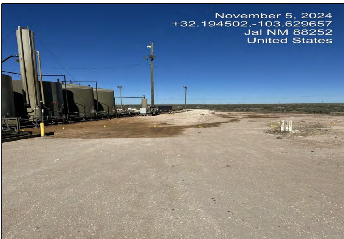
View North - A portion of the release footprint. Note the surface staining (i.e., dark brown color). Release caused by a corroded valve on a LACT unit.
