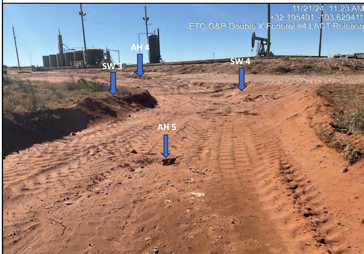
View North - Remediation activities (i.e., excavation and stockpiling) in progress. Sample locations AH 4, AH 5, SW 3, and SW 4.
