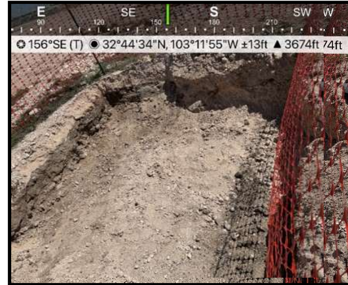
View of Excavation (5/13/26)
