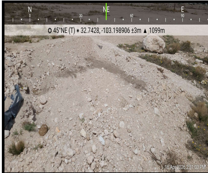
View of Excavation (4/16/26)
