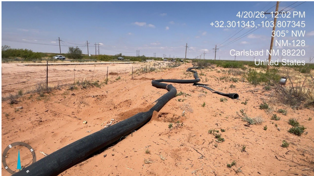
Photograph showing a completed boring of a delineation sample location, viewing northwest.
