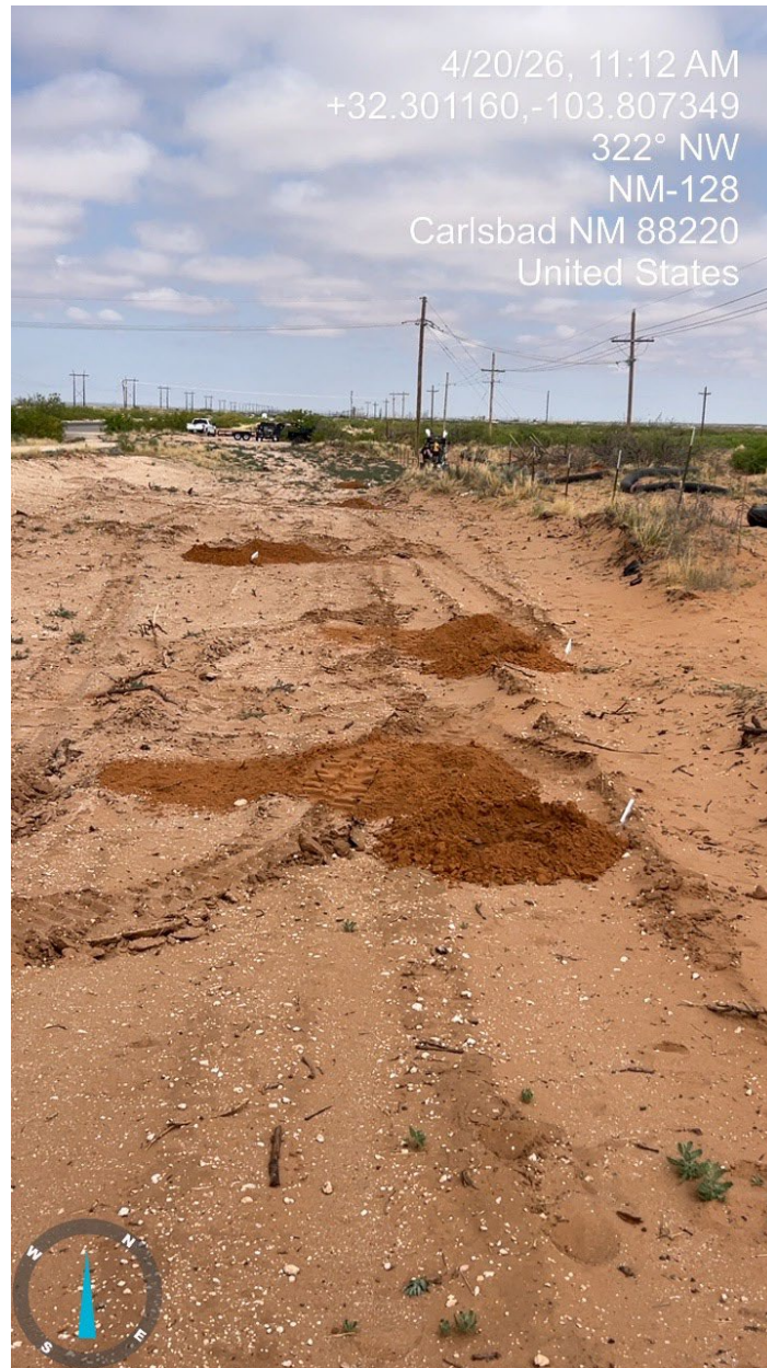
Photograph showing a completed boring of a delineation sample location, viewing northwest.
