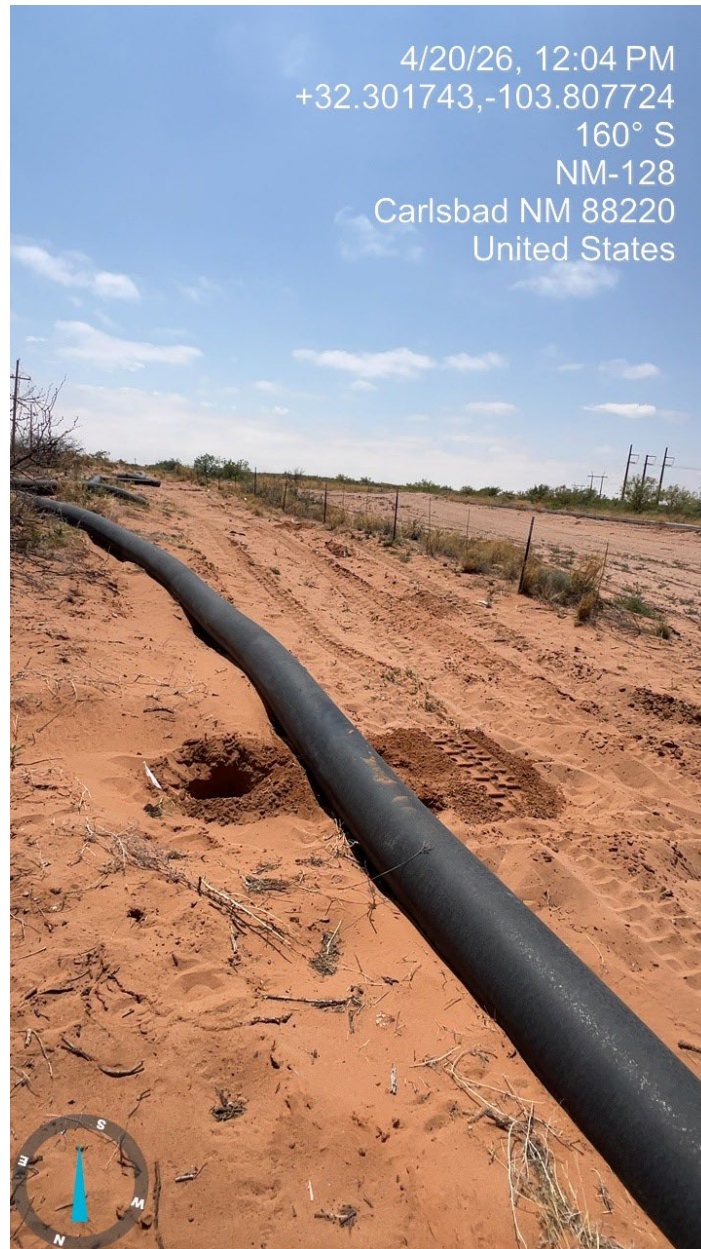
Photograph showing a completed boring of delineation sample location, viewing south.
