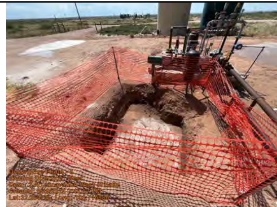
2' excavation West of battery
