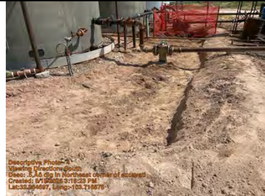
.5' dig in Northeast corner of excavation
