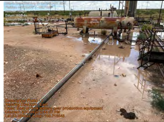
East of tank battery near production equipment
