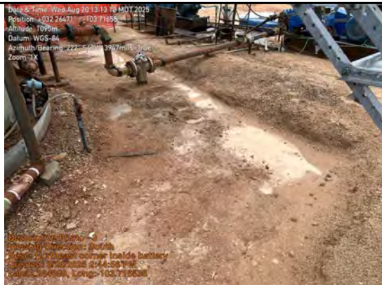
Northeast corner inside battery
