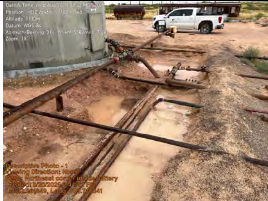
Northeast corner inside battery
