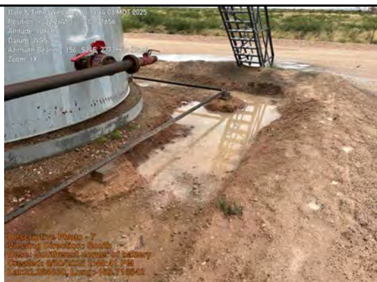
Southwest corner of battery
