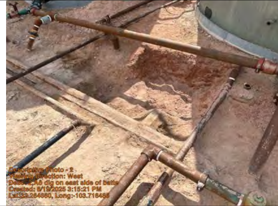
2' dig on east side of battery
