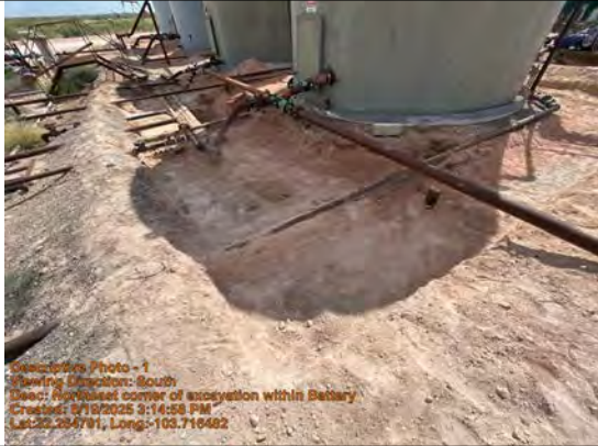
Northeast corner of excavation within Battery
