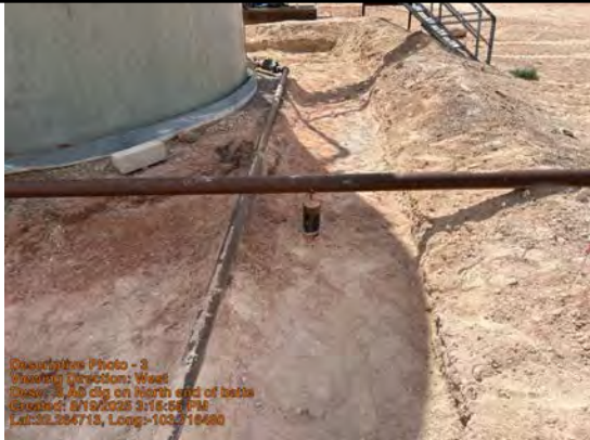
.5' dig on North end of battery
