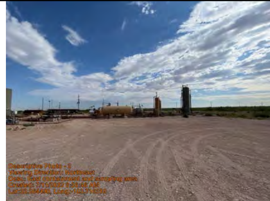
East containment and sampling area
