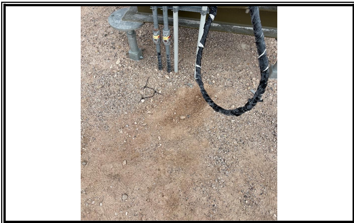
View of the site following discovery of the release. (Photo Provided by WES)
