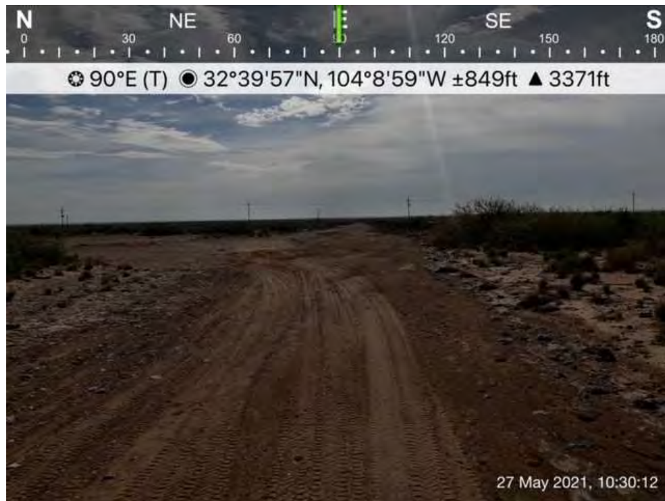
Saturated soil on lease road, Spill Area D, viewing to the east.
