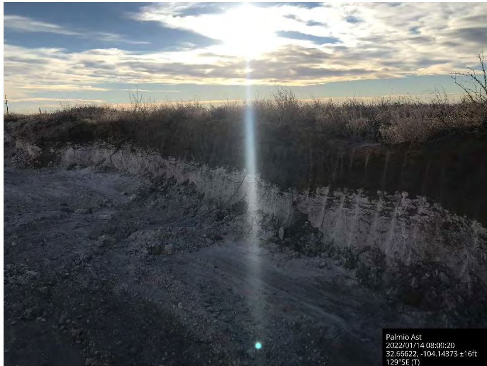
Further excavation of sidewall in pasture, Spill Area B, viewing to the southeast.
