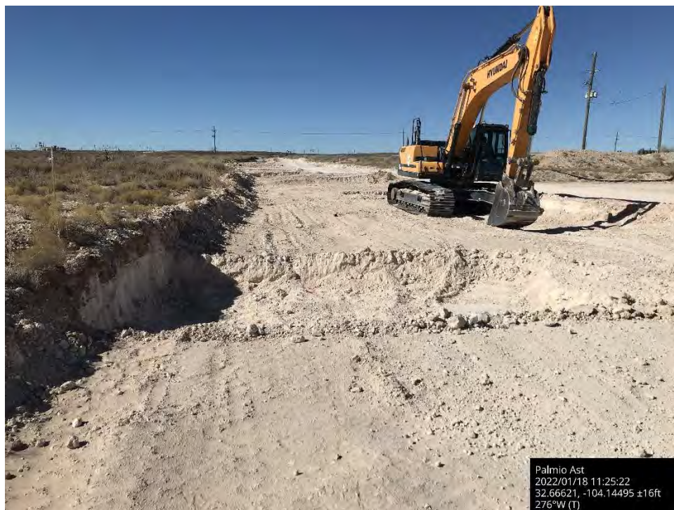
Further excavation on lease road, Spill Area C, viewing to the west.
