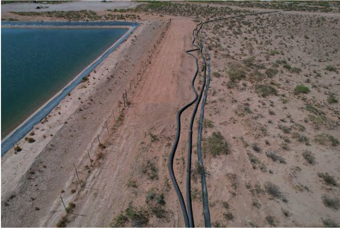
Drone imagery of seeded and contoured area in pasture on June 15, 2022, Spill Area E, viewing to the north. Coordinates: 32°40'08.3"N, 104°09'20.8"W
