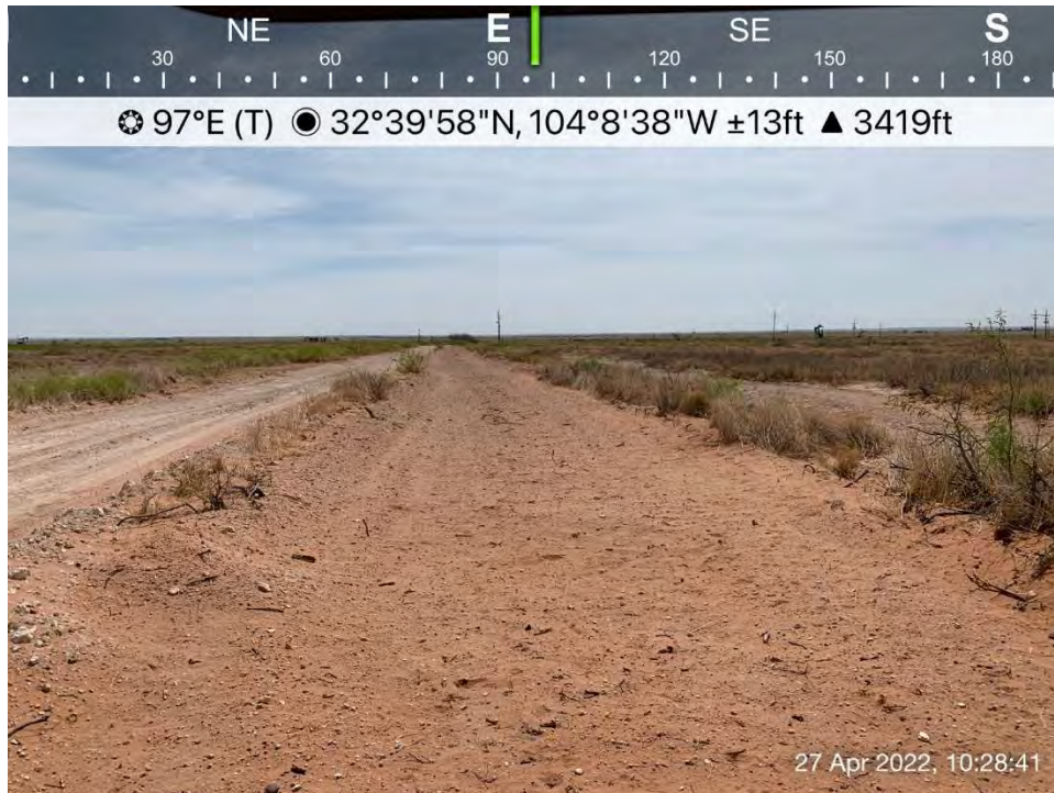
Backfilled excavation on lease road, Spill Area B, viewing to the east.
