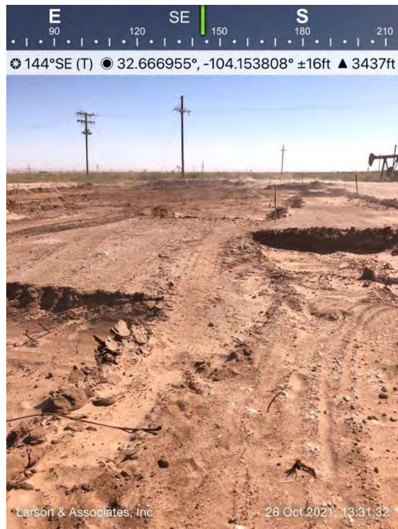
Further excavation on pad south of frac pond, Spill Area D, viewing southeast.
