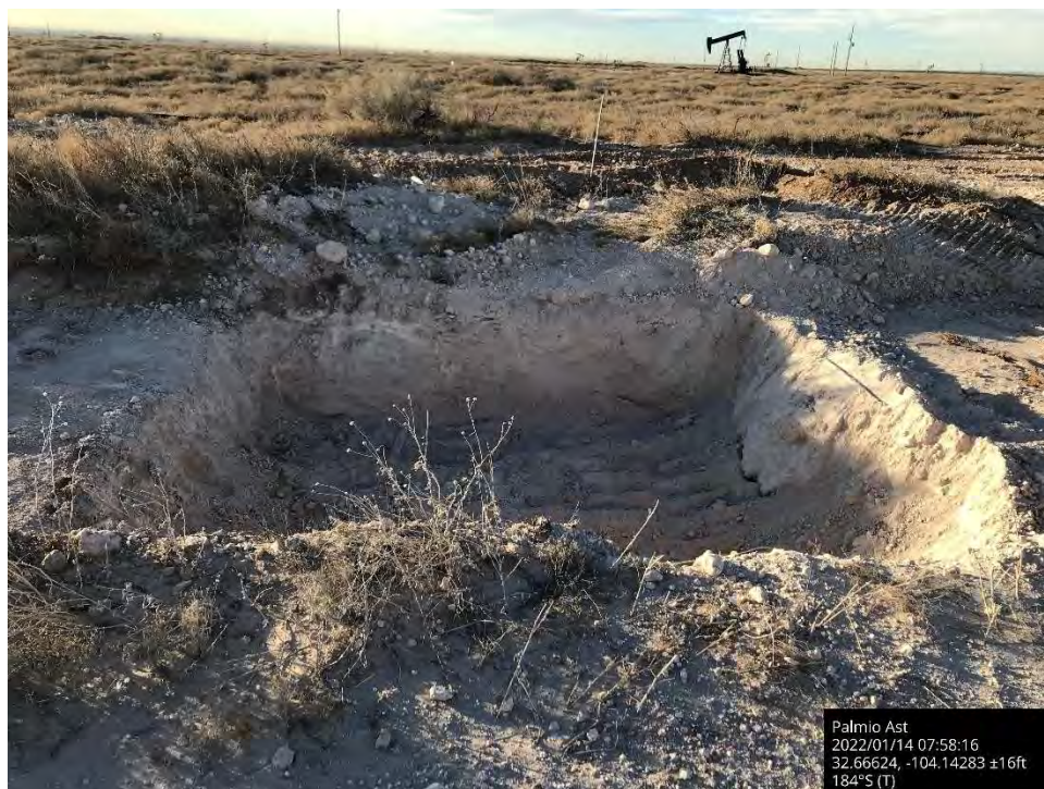
Further excavation in pasture, Spill Area B, viewing to the south.
