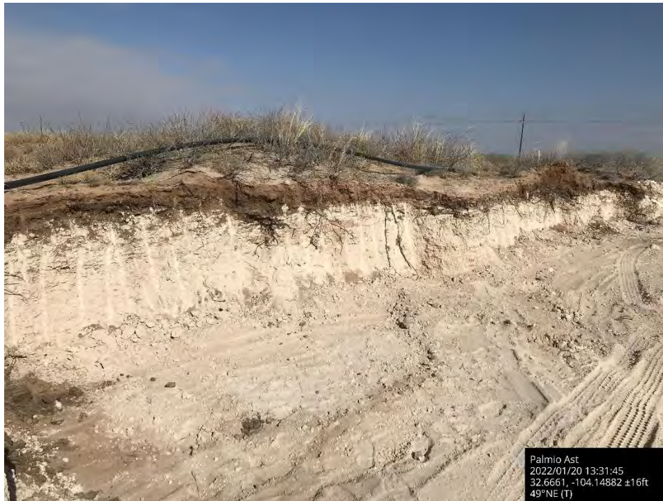
Further excavation of sidewall on lease road, Spill Area C, viewing to the northeast.
