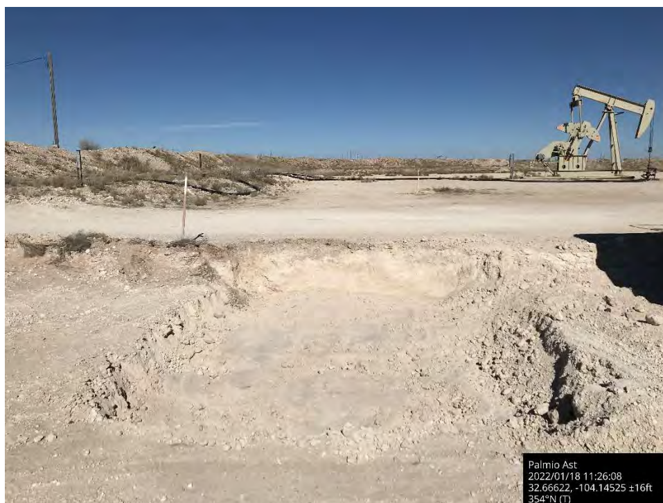
Further excavation on lease road, Spill Area C, viewing to the north.
