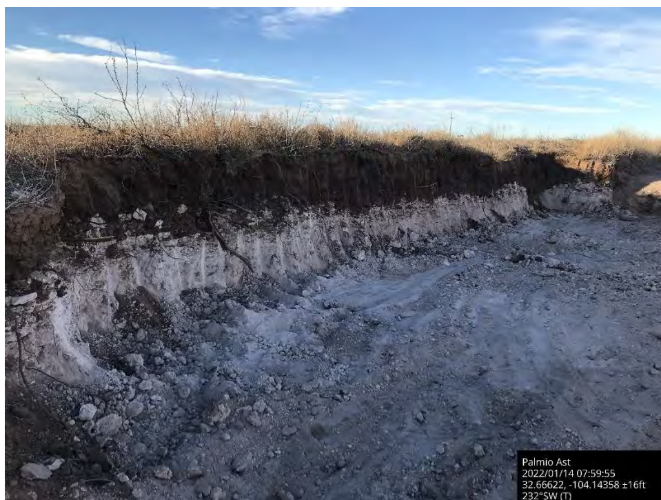
Further excavation of sidewall in pasture, Spill Area B, viewing to the southwest.
