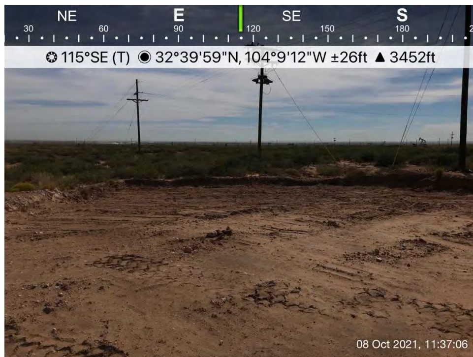
Excavated area on the pad and in the pasture, Spill Area D, viewing to the southeast.
