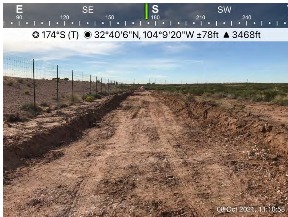
Excavated area west of the frac pond, Spill Area E, viewing to the south.
