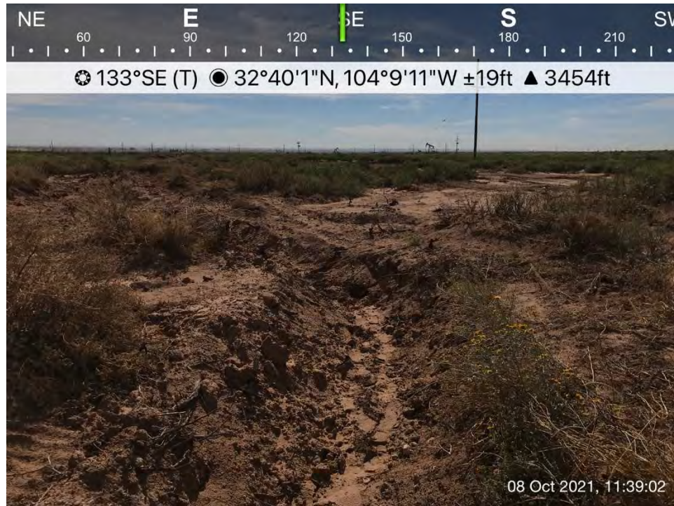
Excavated area in pasture east of the pad, Spill Area D, viewing to the southeast.
