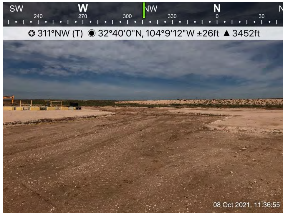
Excavated area on pad, Spill Area D, viewing to the northwest.
