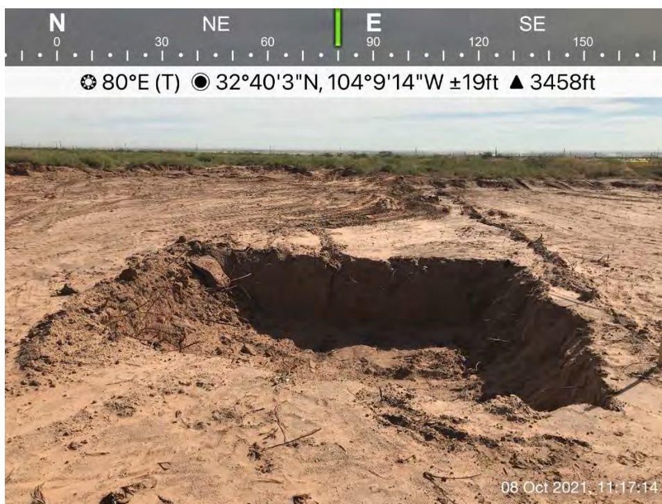
Further excavated area south of the frac pond, Spill Area E, viewing to the east.
