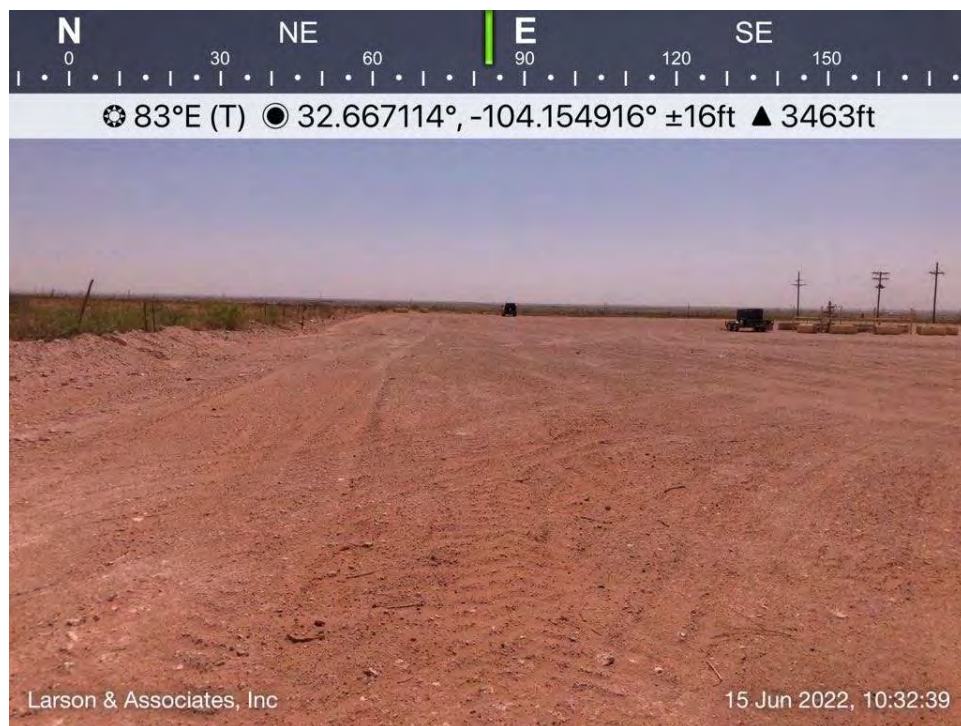
Backfilled area on pad, Spill Area D, viewing to the east.
