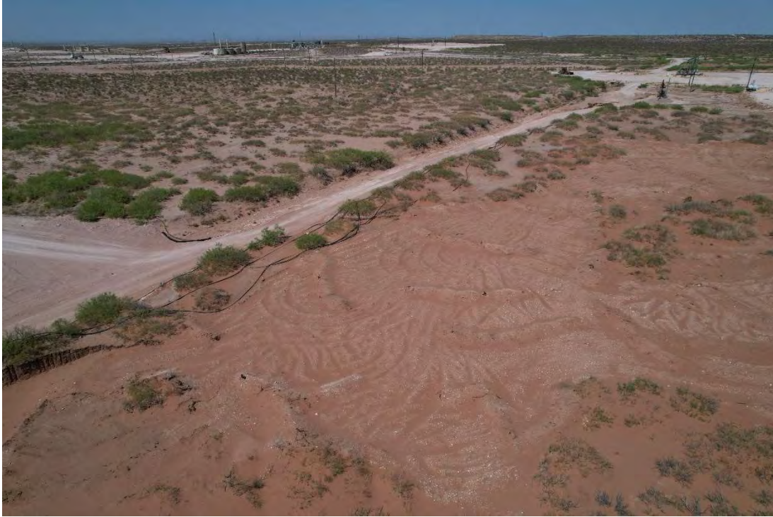
Drone imagery of seeded and contoured area in pasture and backfilled lease road on June 15, 2022, Spill Area D, viewing to the southwest. Coordinates: 32°39'59.3"N, 104°09'05.9"W
