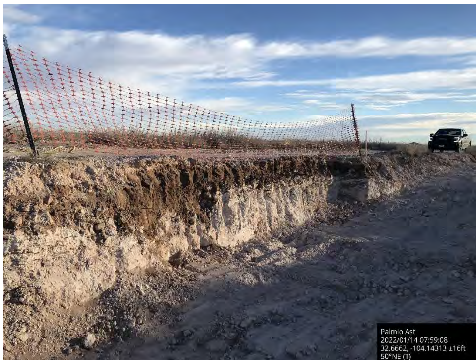
Further excavation of sidewall in pasture, Spill Area B, viewing to the northeast.
