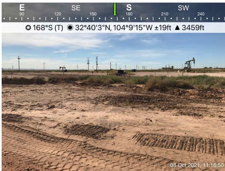
Excavated area south of the frac pond, Spill Area E, viewing to the south.
