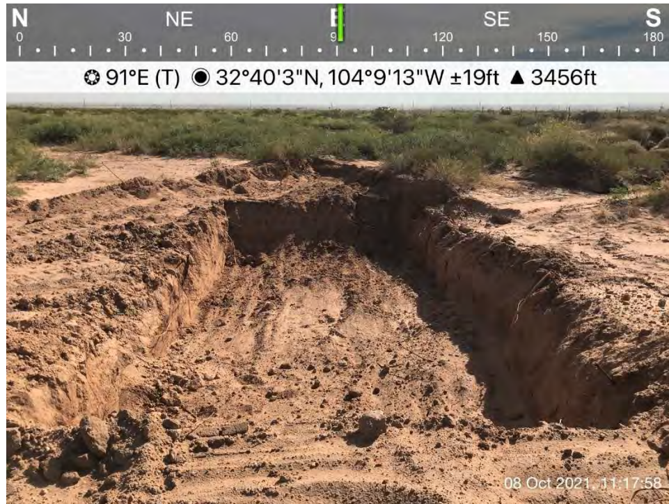
Further excavated area south of the frac pond, Spill Area E, viewing east.
