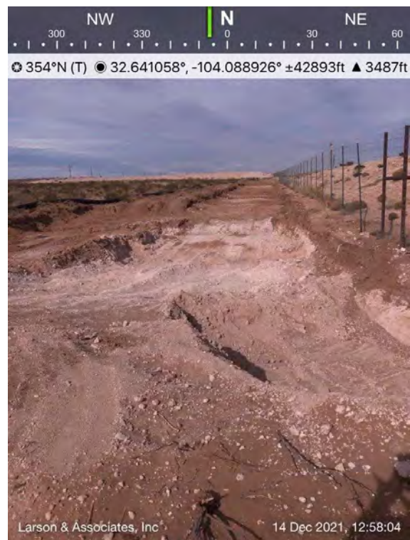
Further excavation south of the frac pond, Spill Area E, viewing to the north.
