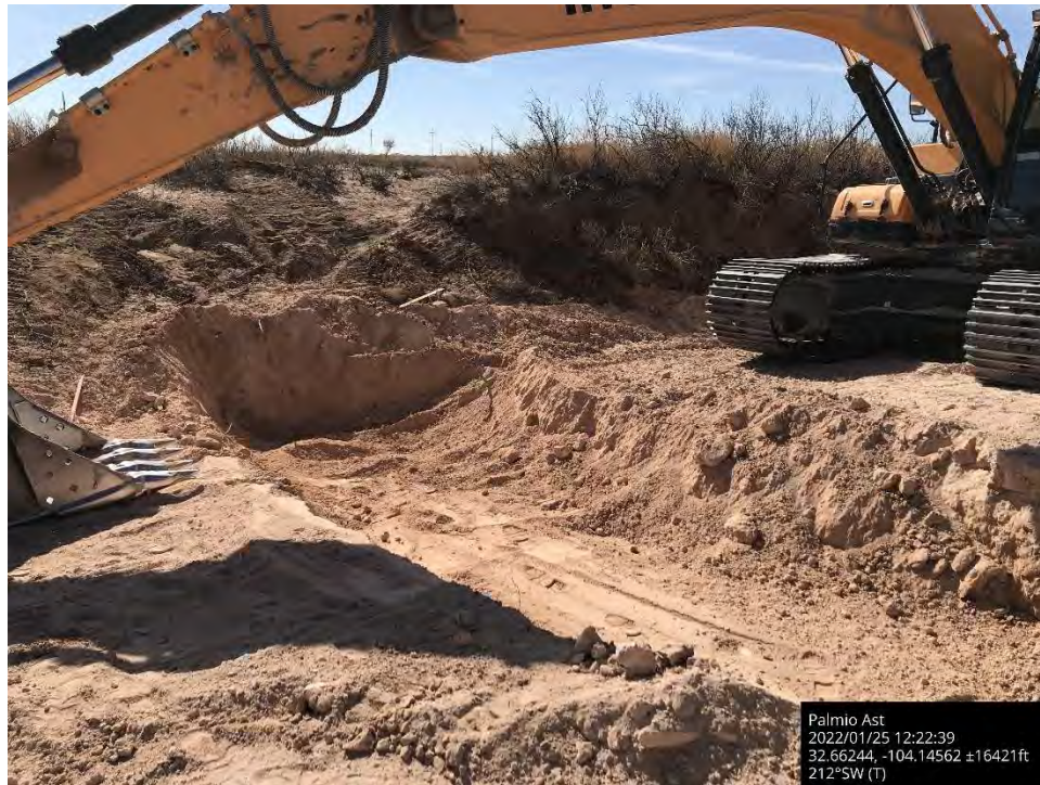
Further excavation on lease road, Spill Area D, viewing to the southwest.
