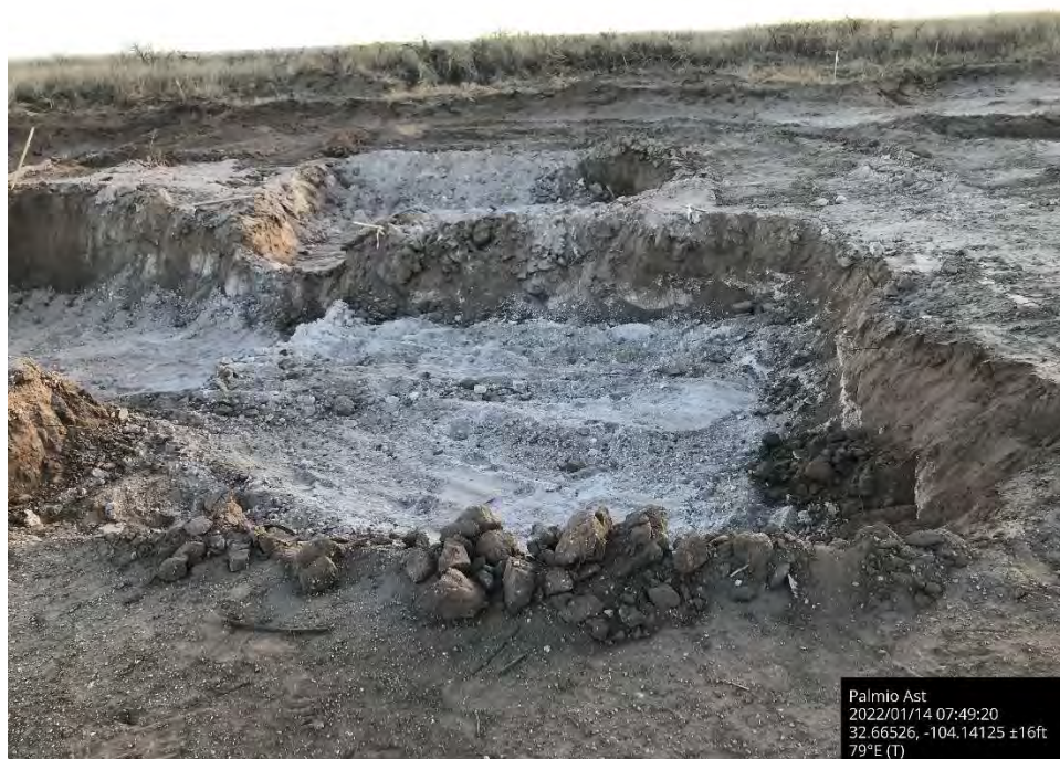
Further excavation in pasture, Spill Area A, viewing to the east.
