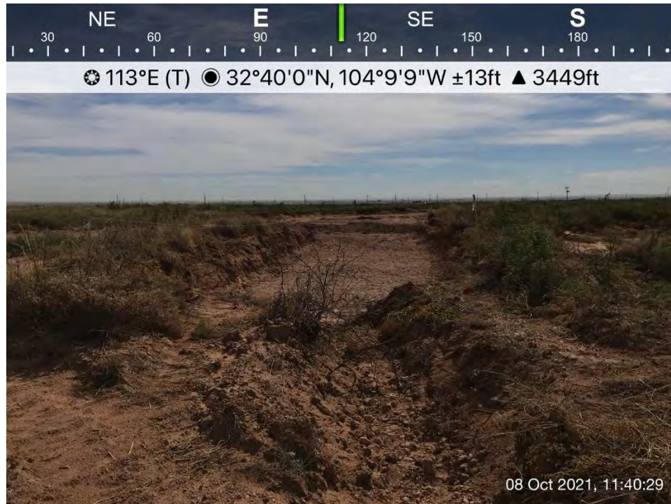
Excavated area in pasture east of the pad, Spill Area D, viewing to the east.
