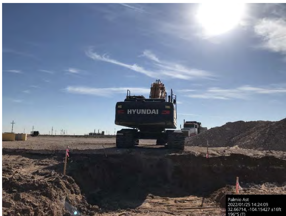
Further excavation on pad, Spill Area D, viewing to the south.
