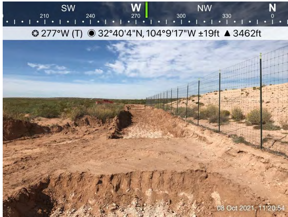
Further excavated areas south of the frac pond, Spill Area E, viewing to the west.
