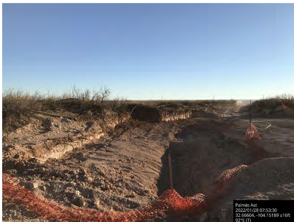
Further excavation on lease road, Spill Area D, viewing to the east.
