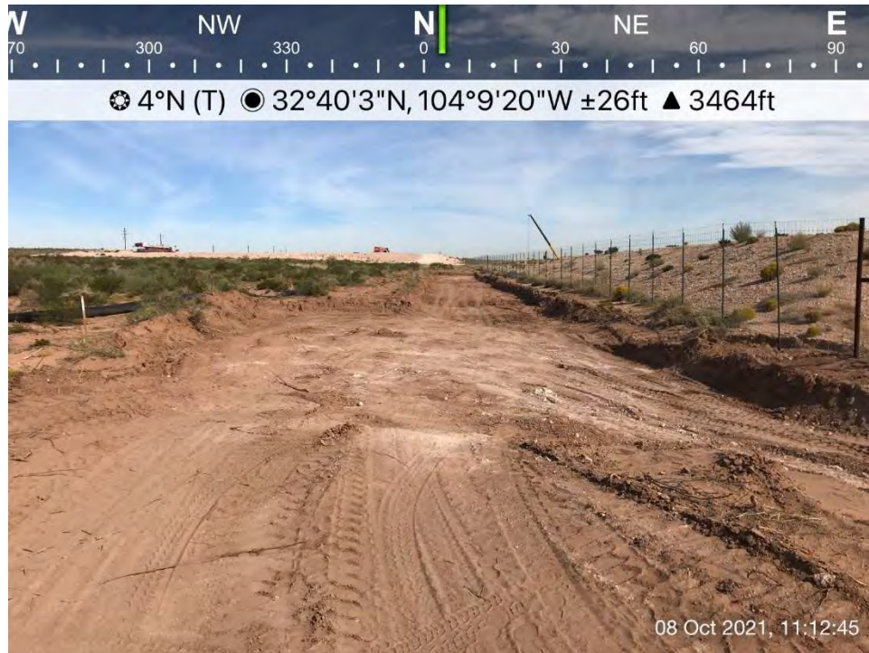
Excavated area west of the frac pond, Spill Area E, viewing to the north.
