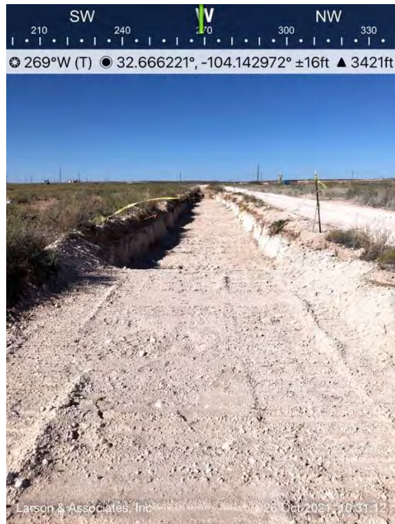
Excavated area in pasture, Spill Area B, viewing to the west.
