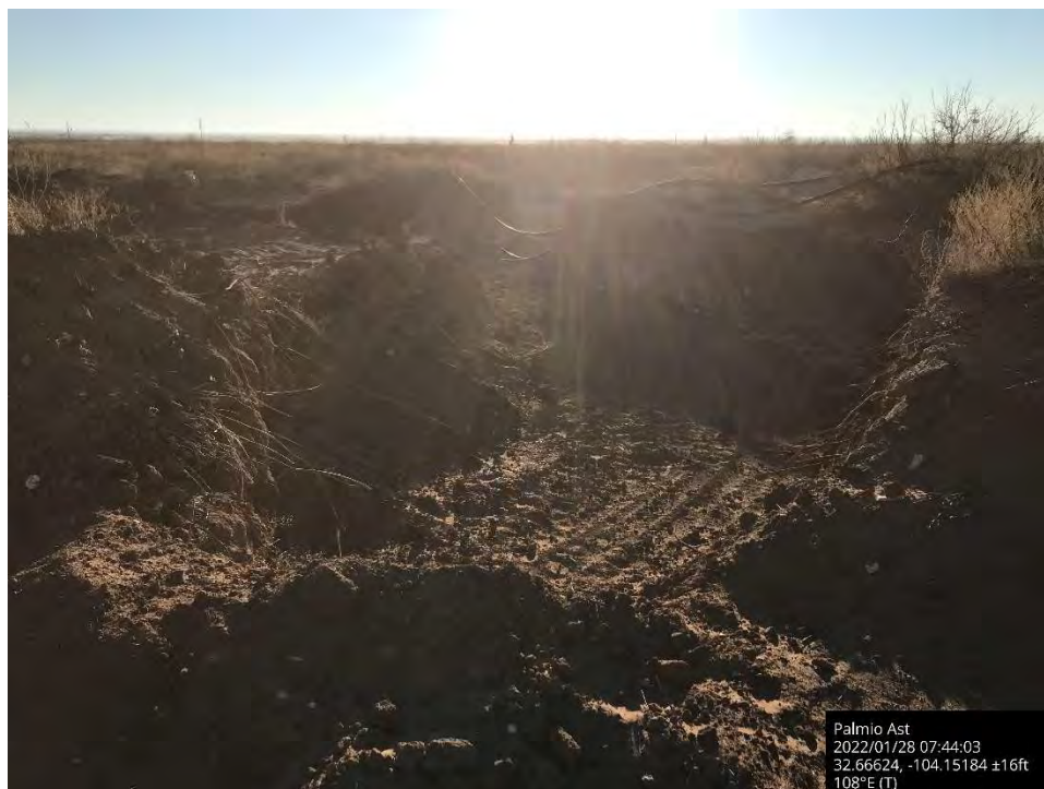
Further excavation in pasture, Spill Area D, viewing to the east.
