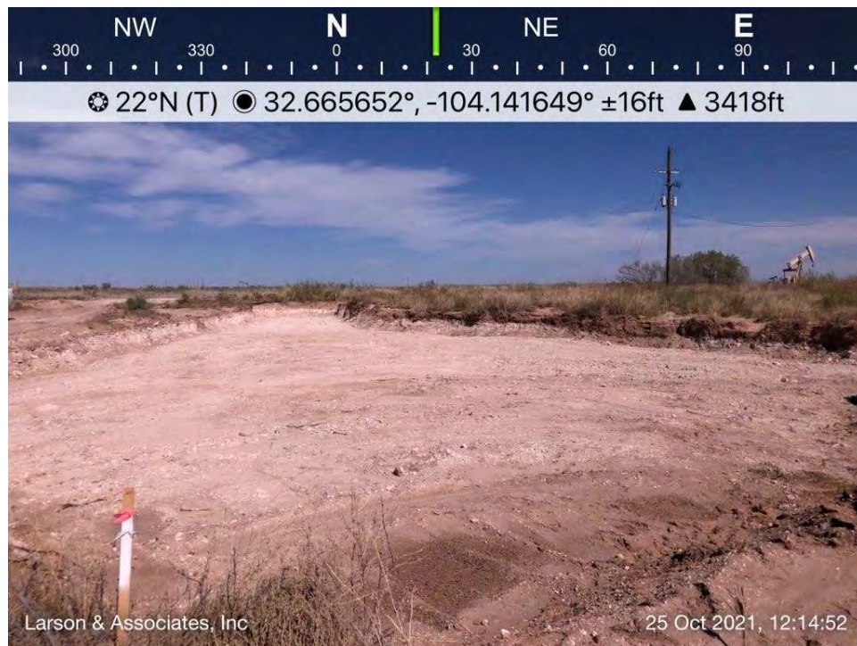
Excavated area in pasture, Spill Area A, viewing to the north.
