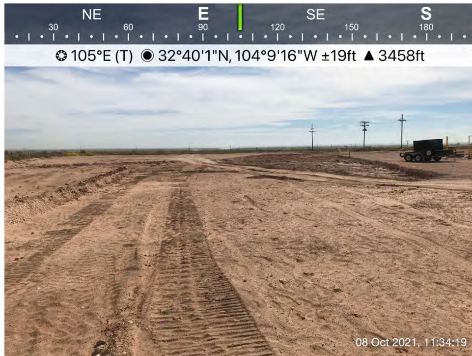
Excavated area on pad, Spill Area D, viewing to the east.
