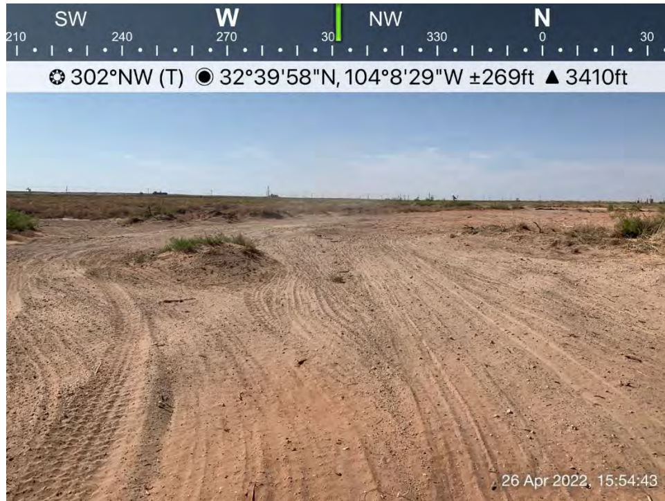
Backfilled and seeded excavation in pasture, Spill Area A, viewing to the northwest.
