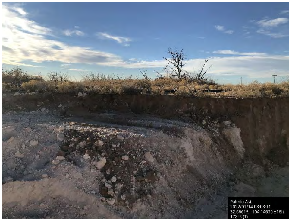
Further exaction of sidewall on lease road, Spill Area C, viewing to the south.
