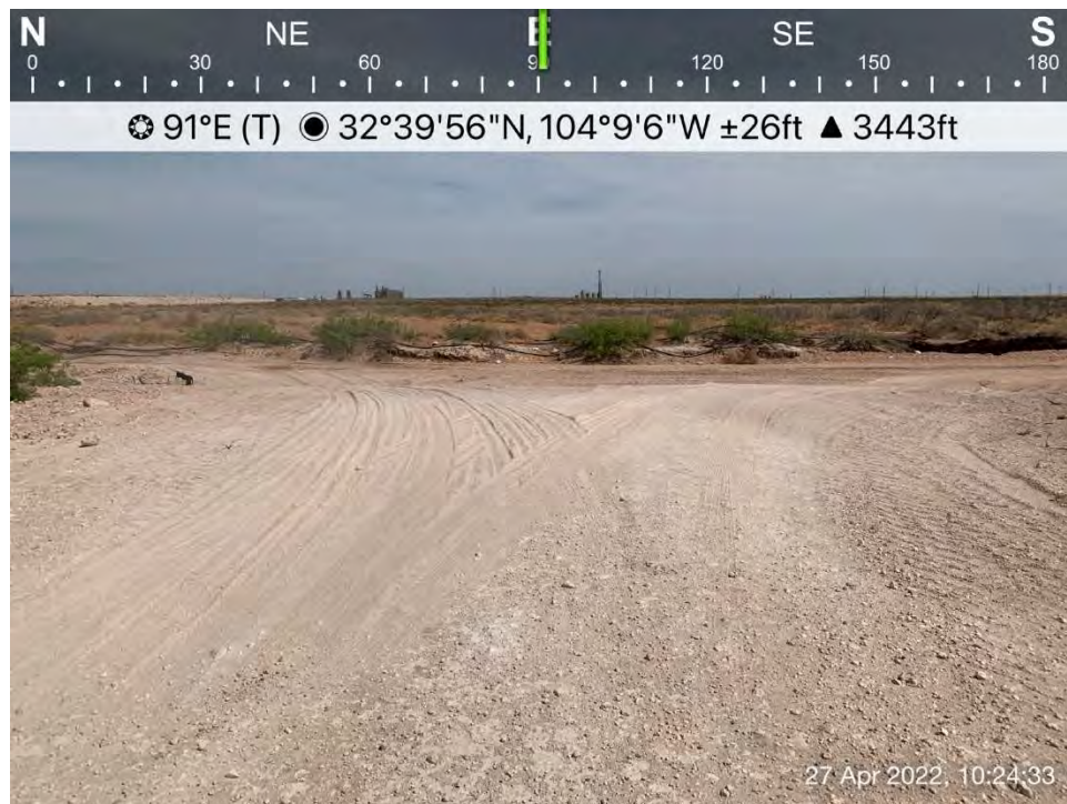
Backfilled excavation on lease road, Spill Area D, viewing to the east.
