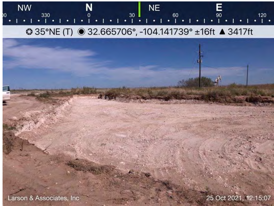
Excavated area in pasture, Spill Area A, viewing to the northeast.
