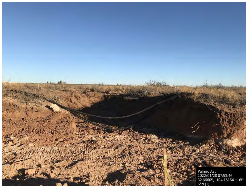
Further excavation on lease road, Spill Area D, viewing to the north.
