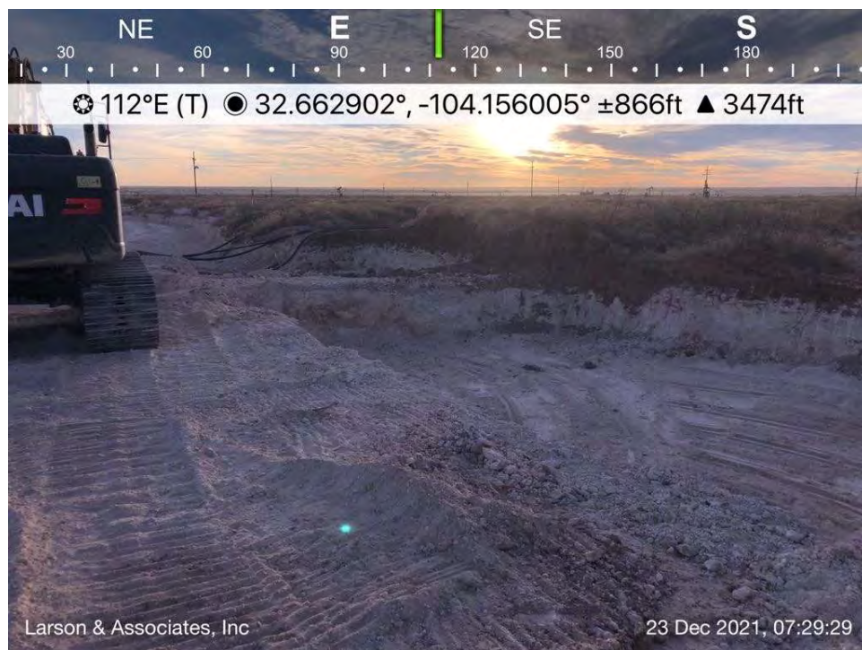
Further exaction on lease road, Spill Area C, viewing to the east.
