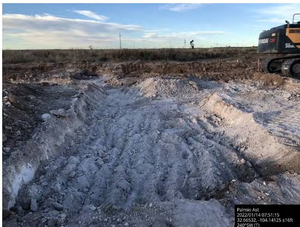
Further excavation in pasture, Spill Area A, viewing to the southwest.
