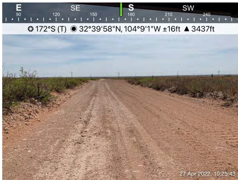
Backfilled excavation on lease road, Spill Area D, viewing to the south.
