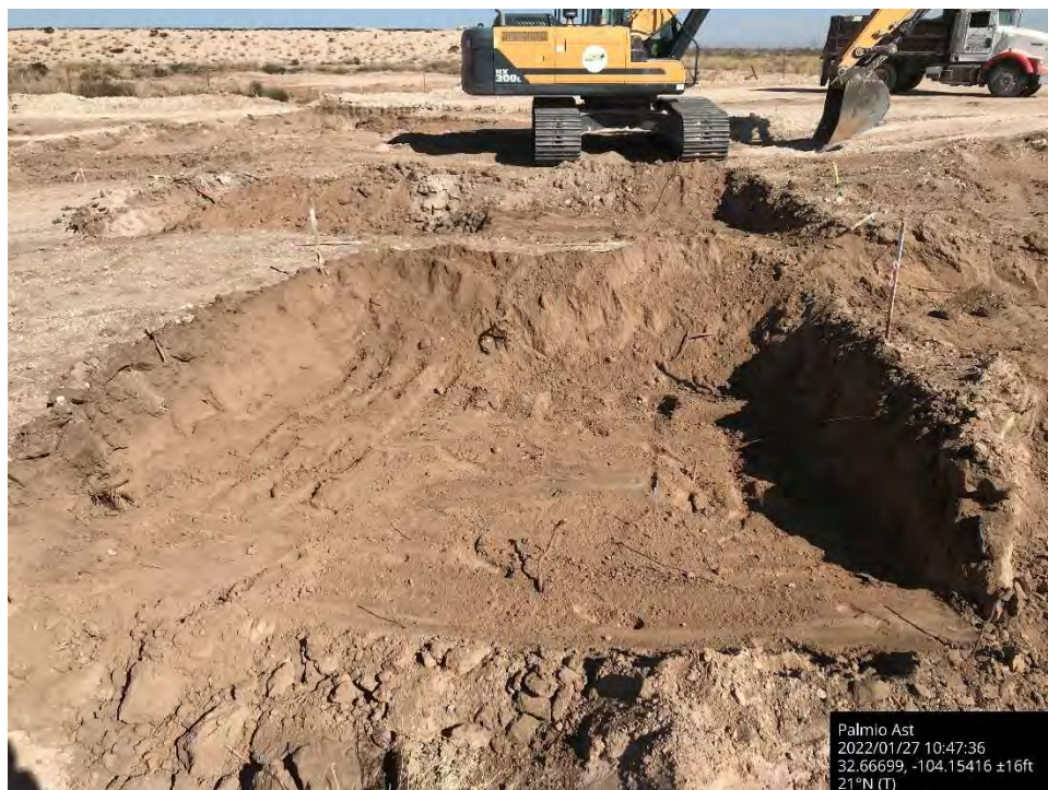
Further excavation on pad, Spill Area D, viewing to the north.
