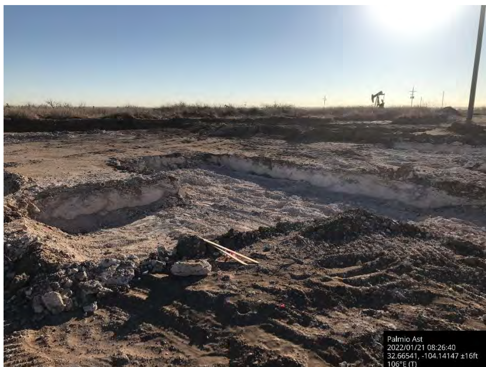
Further excavation in pasture, Spill Area A, viewing to the east.
