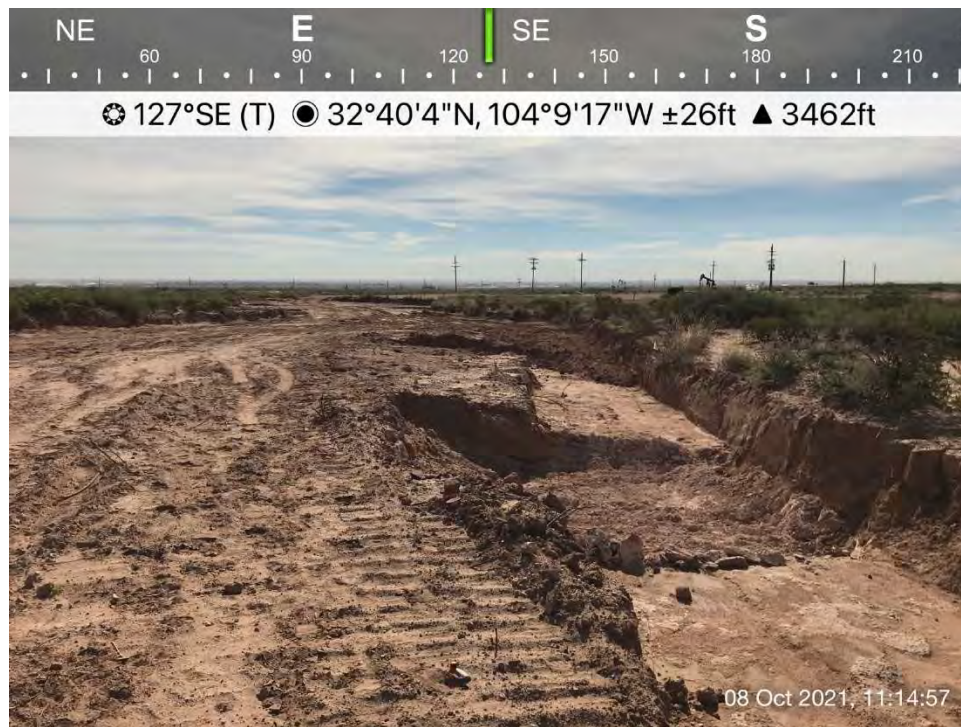
Further excavated areas south of frac pond, Spill Area E, viewing to the southeast.
