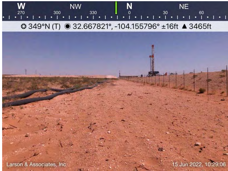
Backfilled area west of the frac pond, Spill Area E, viewing to the north.
