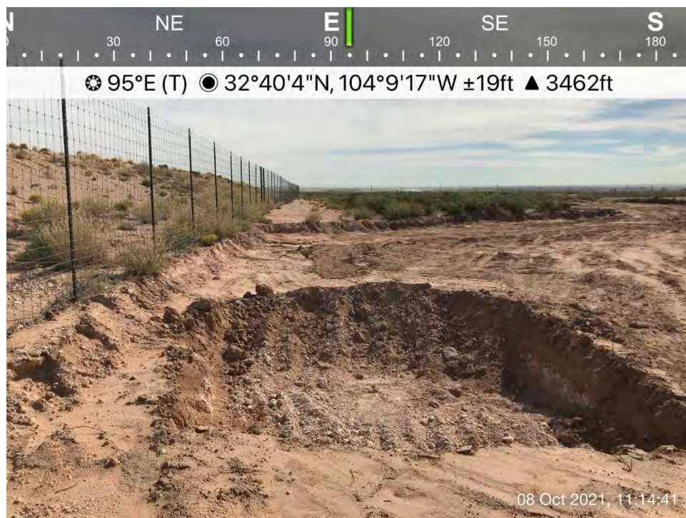
Further excavated area south of the frac pond, Spill Area E, viewing to the east.
