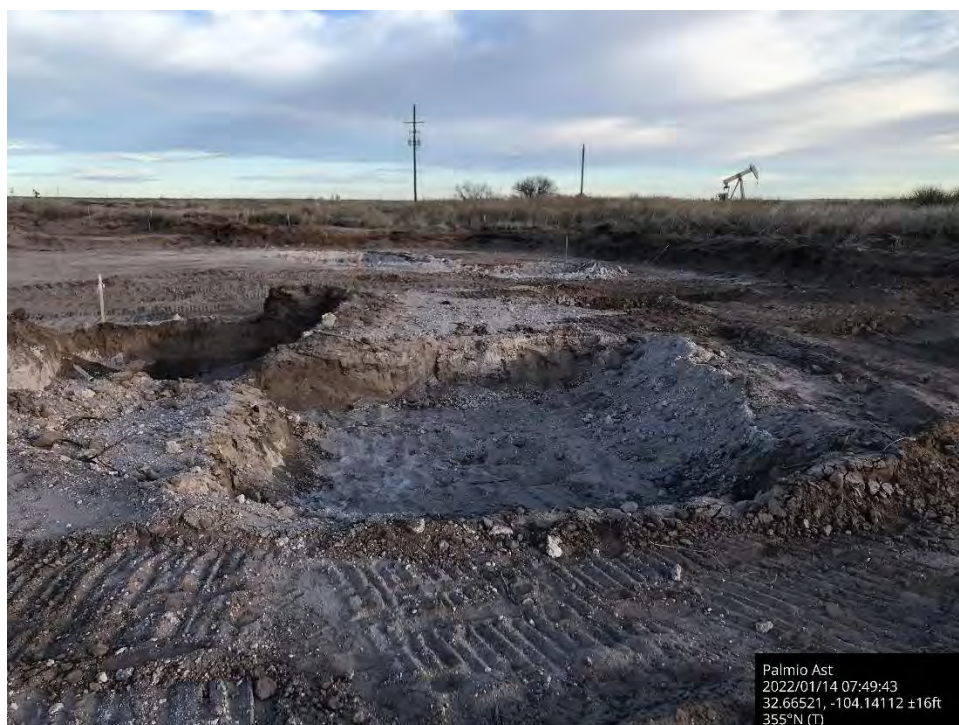
Further excavation in pasture, Spill Area A, viewing to the north.
