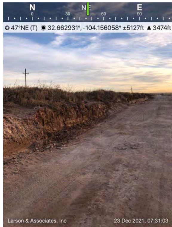
Further excavation of sidewall on lease road, Spill Area C, viewing to the northeast.
