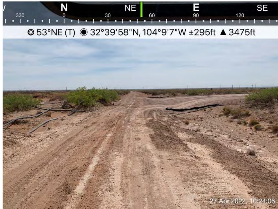
Backfilled excavation on lease road, Spill Area D, viewing to the northeast.
