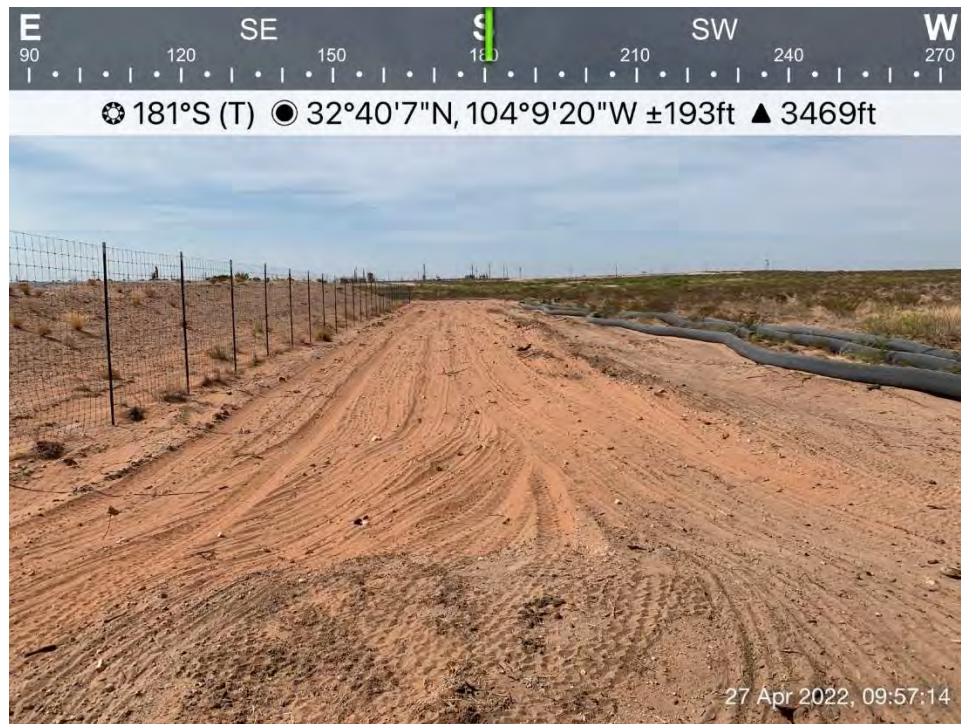
Backfilled and seeded excavation in pasture, Spill Area E, viewing to the south.
