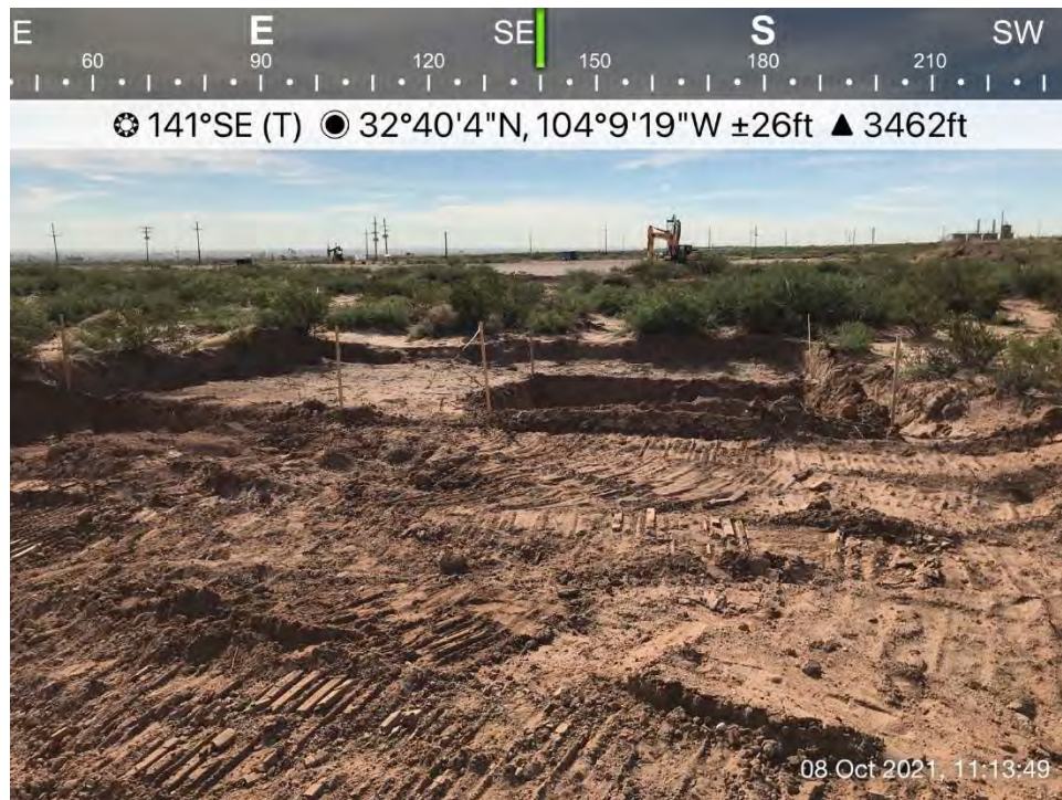
Further excavated area south of frac pond, Spill Area E, viewing to the southeast.
