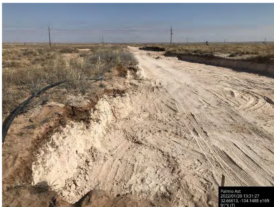
Further excavation of sidewall on lease road, Spill Area C, viewing to the east.
