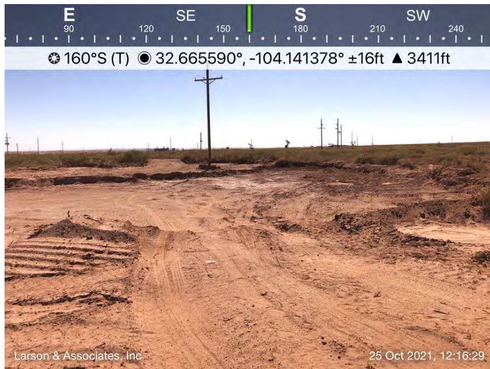
Excavated area in pasture, Spill Area A, viewing to the south.
