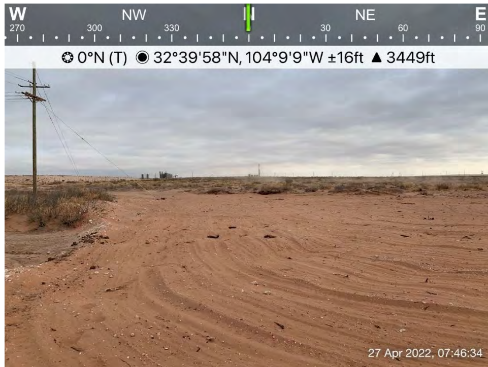
Backfilled and seeded excavation in pasture, Spill Area D, viewing to the north.
