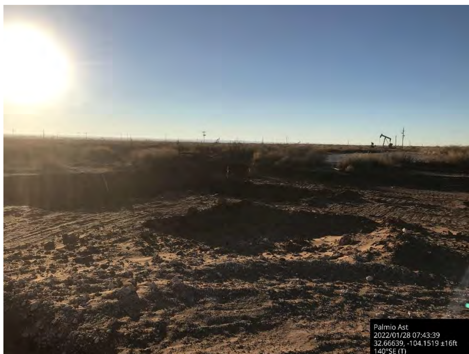
Further excavation in pasture, Spill Area D, viewing to the southeast.
