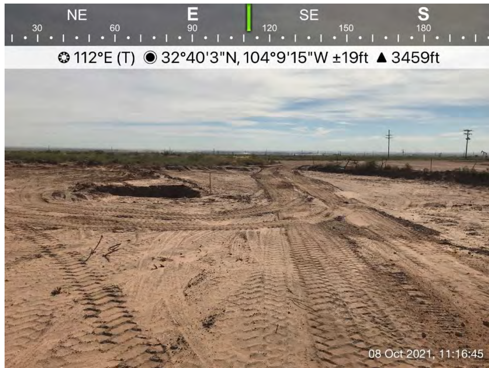
Excavated area in south of the frac pond, Spill Area E, viewing to the east.
