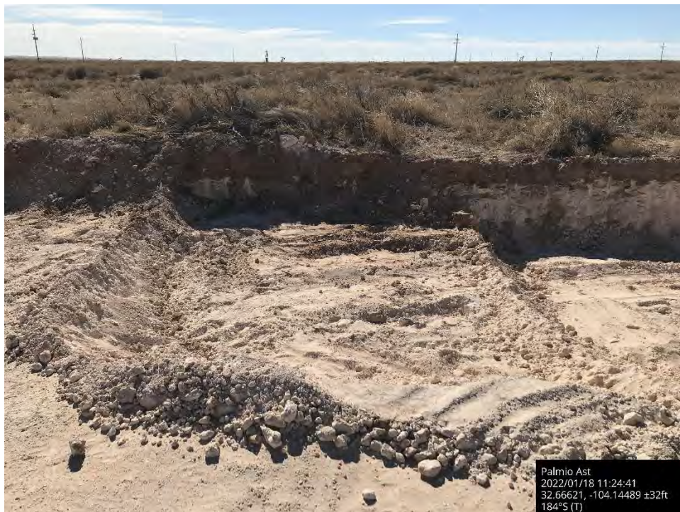
Further excavation on lease road, Spill Area C, viewing to the south.
