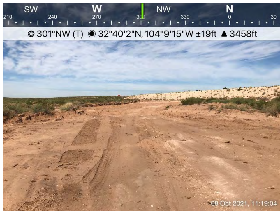
Excavated area south of the frac pond, Spill Area E, viewing to the north.
