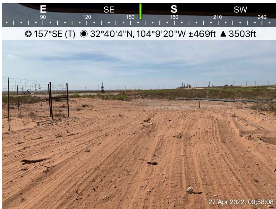
Backfilled and seeded excavation in pasture, Spill Area E, viewing to the southwest.
