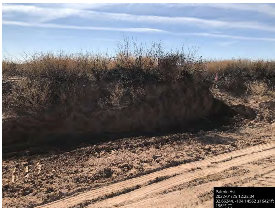
Further excavation of sidewall on lease road, Spill Area D, viewing to the south.
