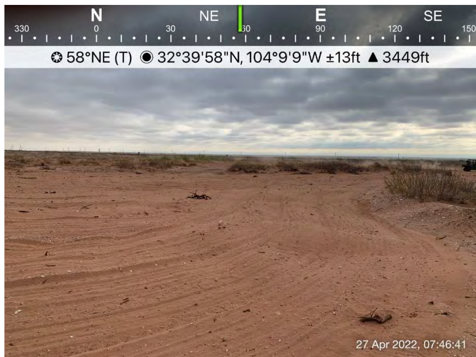
Backfilled and seeded excavation in pasture, Spill Area D, viewing to the northeast.
