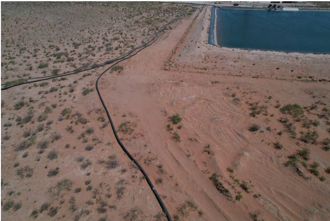
Drone imagery of seeded and contoured area in pasture on June 15, 2022, Spill Area E, viewing to the north. Coordinates: 32°40'02.2"N, 104°09'19.9"W
