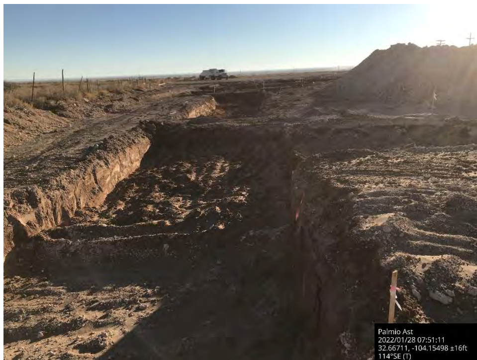
Further excavation on pad, Spill Area D, viewing to the southeast.
