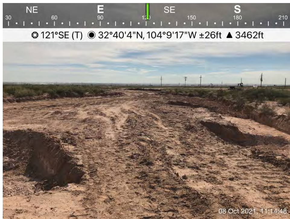
Excavated area south of the frac pond, Spill Area E, viewing to the southeast.
