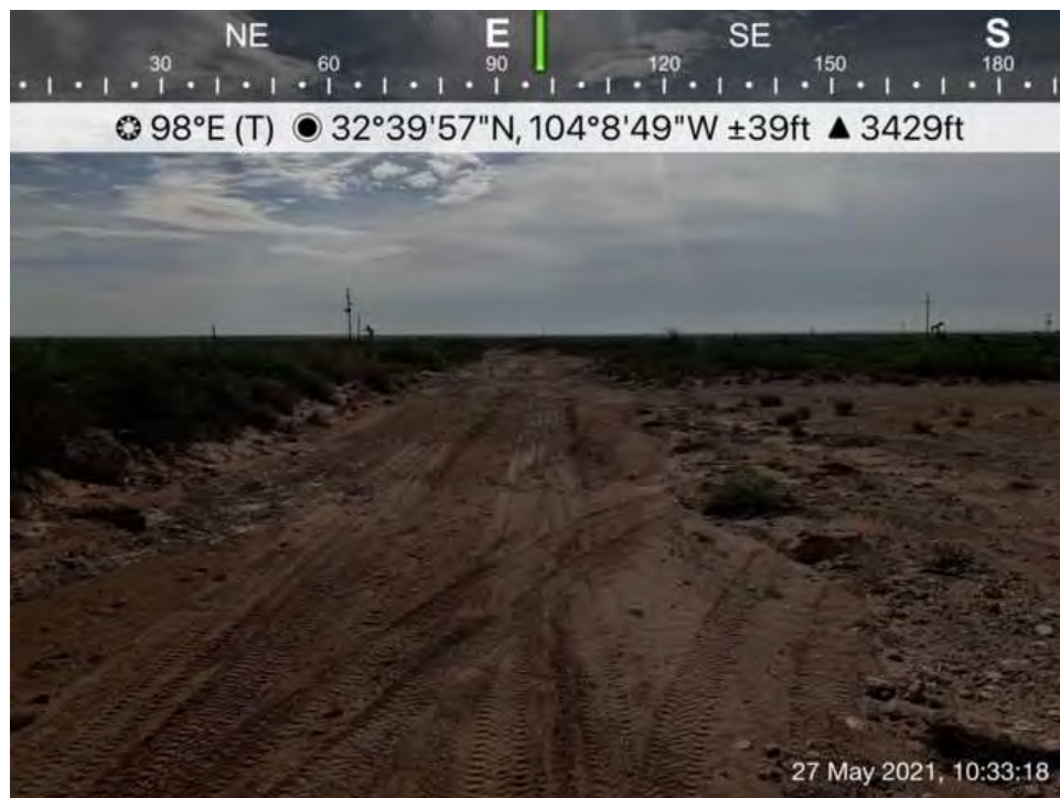
Saturated soil on lease road, Spill Area C, viewing to the east.
