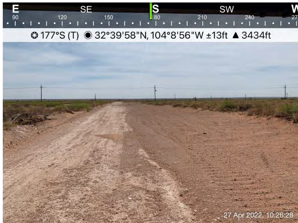
Backfilled excavation on lease road, Spill Area C, viewing to the south.
