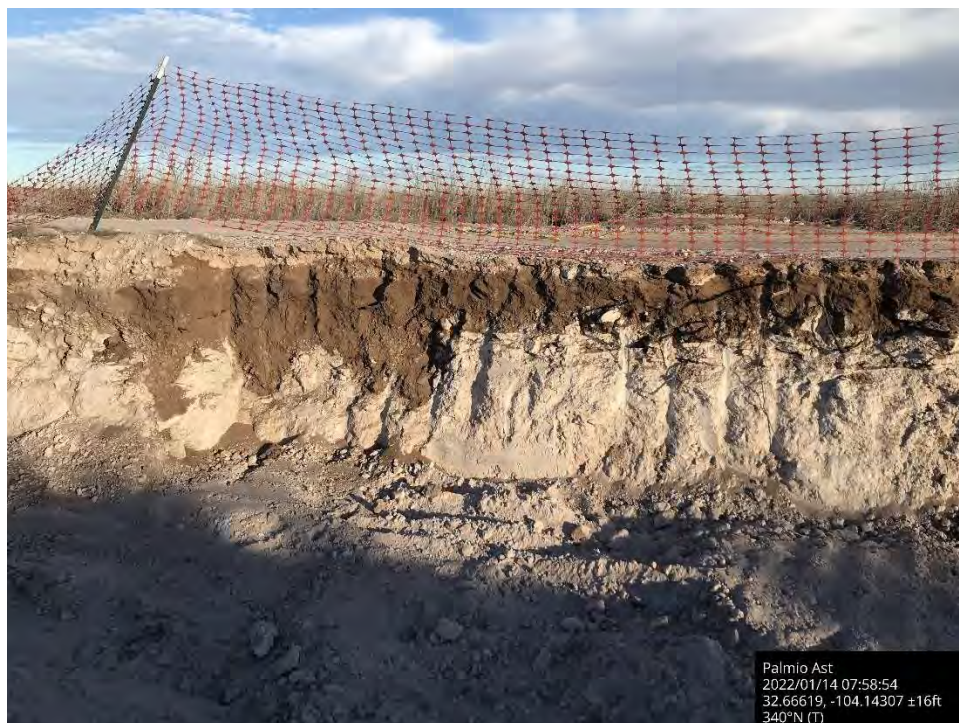
Further excavation of sidewall in pasture, Spill Area B, viewing to the north.
