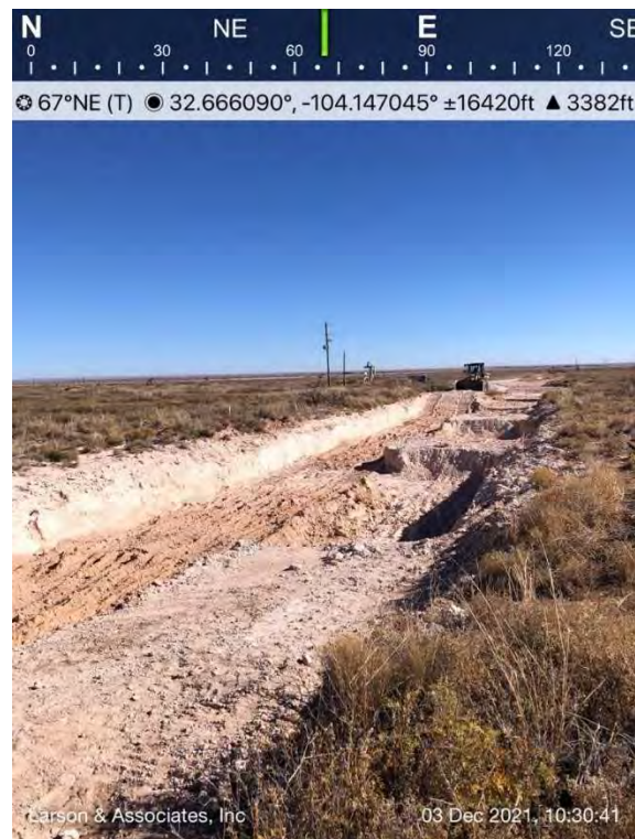
Further excavation on lease road, Spill Area C, viewing to the northeast.
