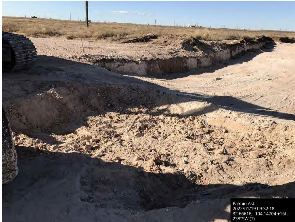
Further excavation on lease road, Spill Area C, viewing to the southwest.
