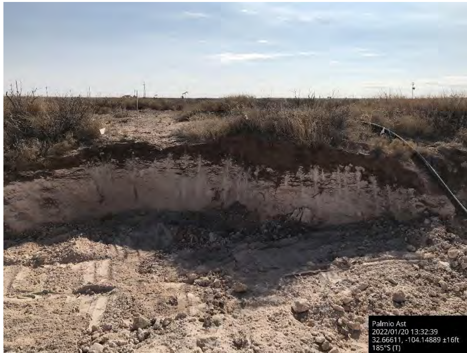
Further excavation of sidewall on lease road, Spill Area C, viewing to the south.
