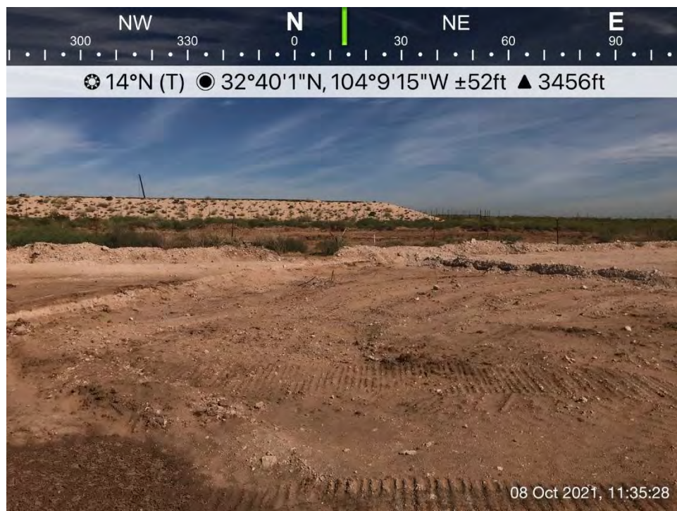
Excavated area on pad, Spill Area D, viewing to the north.
