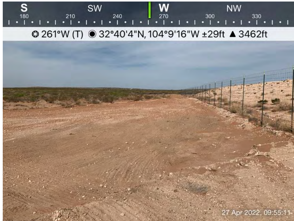
Backfilled and seeded excavation in pasture, Spill Area E, viewing to the west.
