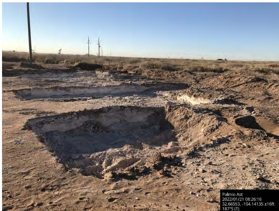
Further excavation in pasture, Spill Area A, viewing to the south.
