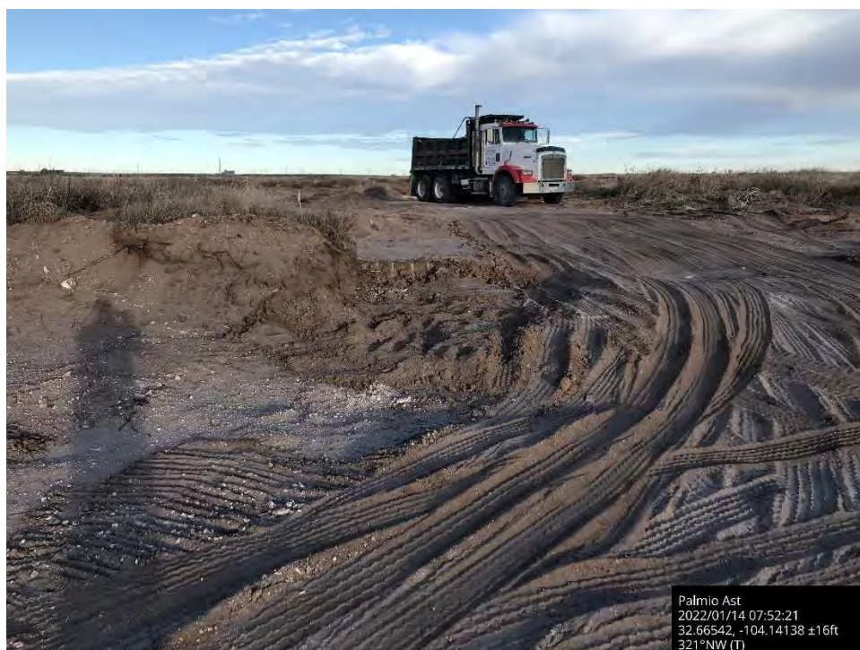
Further excavation in pasture, Spill Area A, viewing to the northwest.
