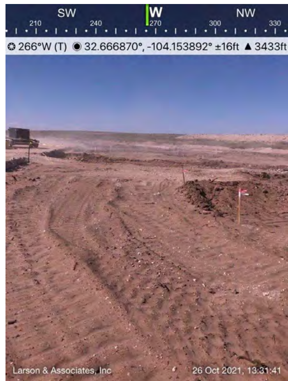
Further excavation on pad south of frac pond, Spill Area D, viewing to the west.
