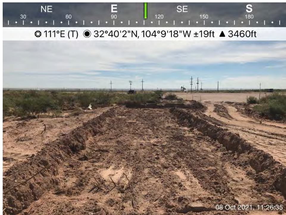
Excavated area south of the frac pond, Spill Area E, viewing to the east.
