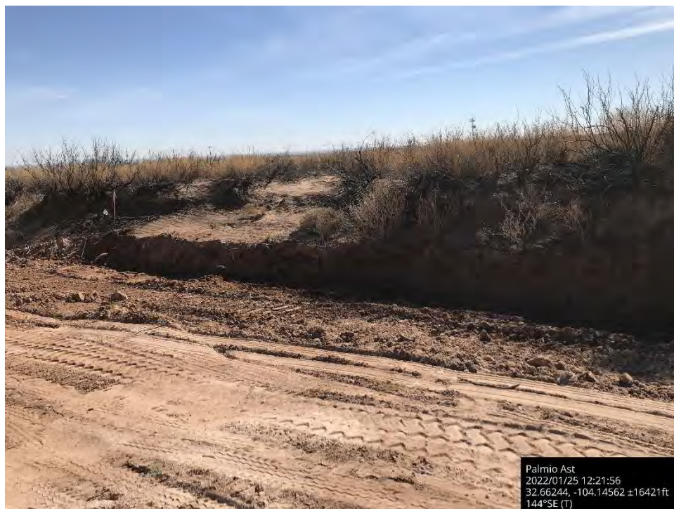
Further excavation of sidewall on lease road, Spill Area D, viewing to the southeast.
