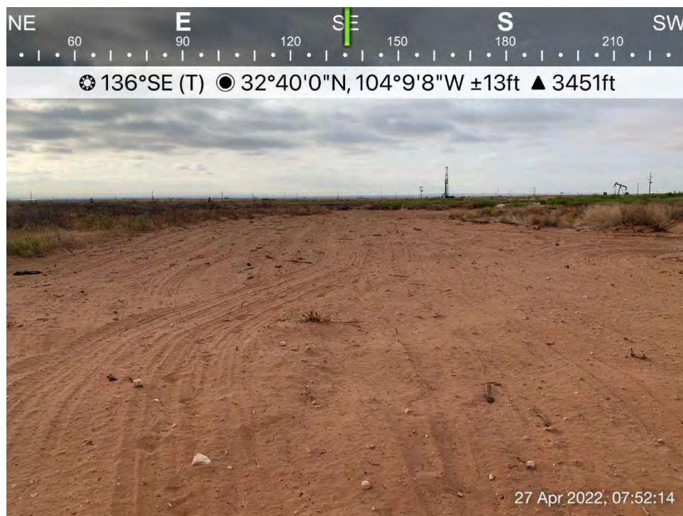
Backfilled and seeded excavation in pasture, Spill Area D, viewing to the southeast.
