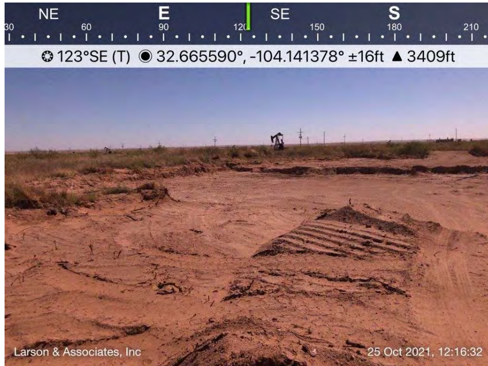
Excavated area in pasture, Spill Area A, viewing to the southeast.
