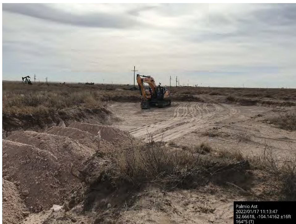
Backing pasture with caliche, Spill Area A, viewing to the south.
