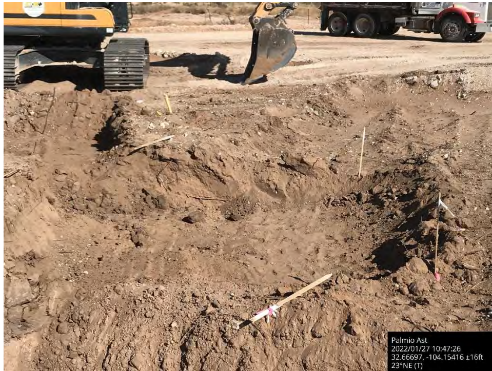
Further Excavation on pad, Spill Area D, viewing to the northeast.
