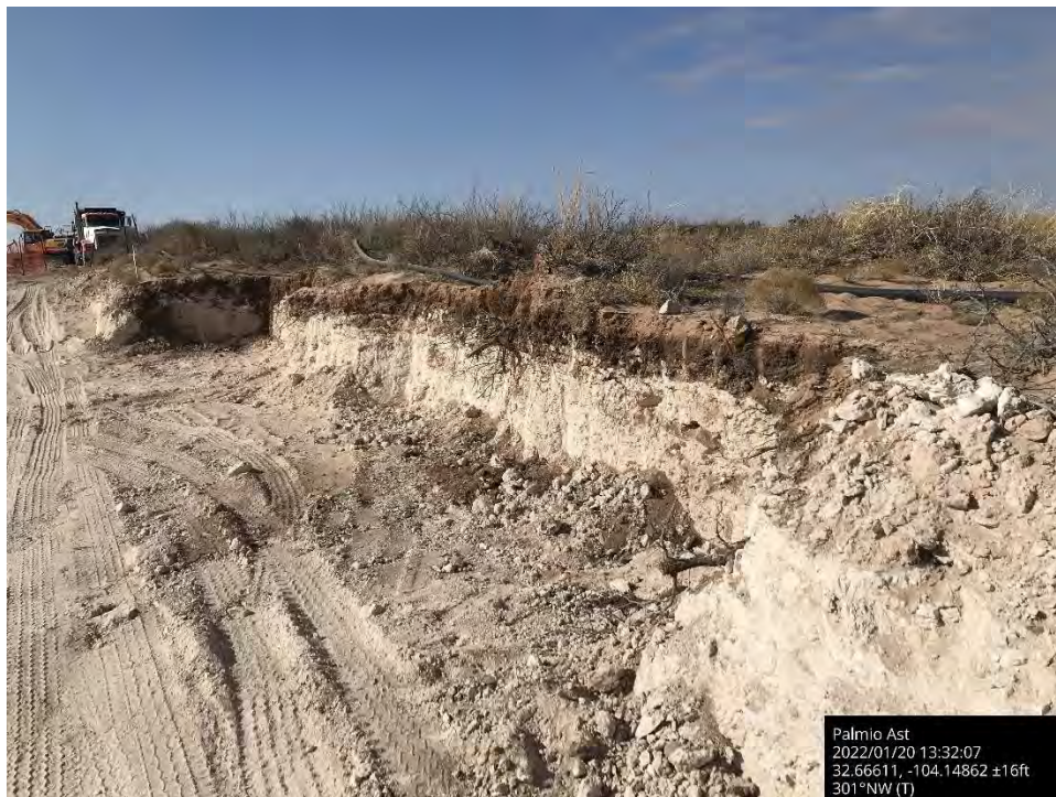
Further Excavation of sidewall on lease road, Spill Area C, viewing to the northwest.
