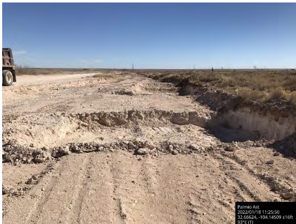
Further excavation on lease road, Spill Area C, viewing to the east.
