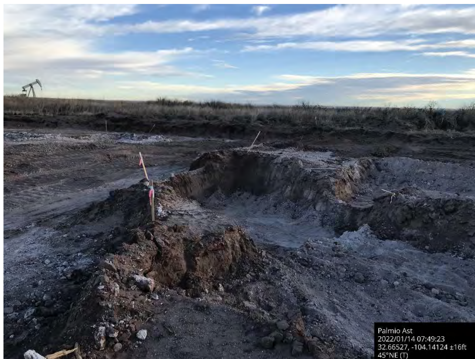
Further excavation in pasture, Spill Area A, viewing to the northeast.
