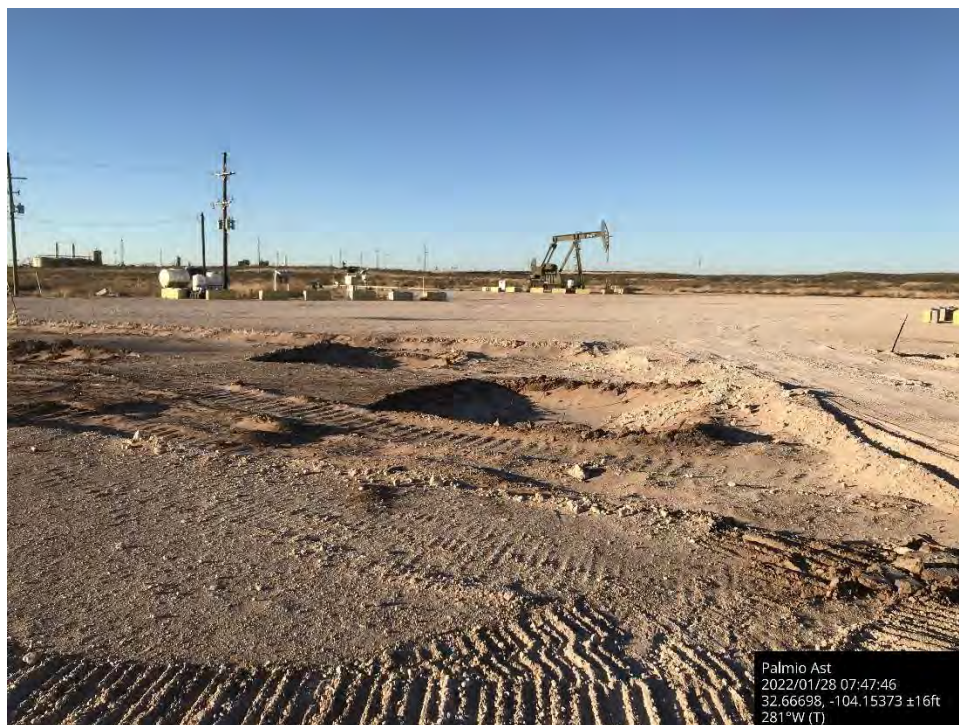
Further excavation on pad, Spill Area D, viewing to the west.
