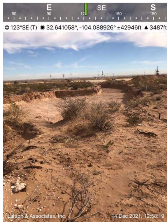
Excavated area south of the frac pond, Spill Area E, viewing to the southeast.
