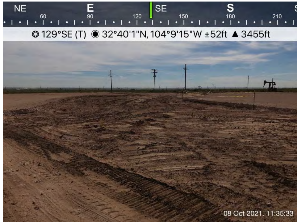
Excavated area on pad, Spill Area D, viewing to the southeast.
