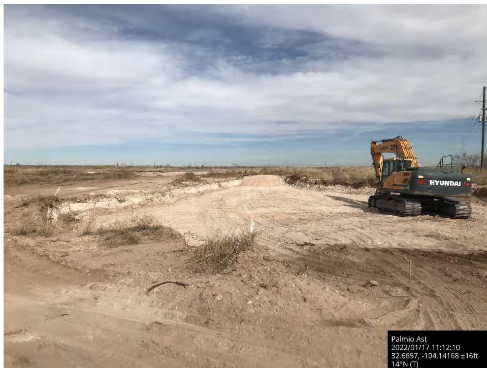
Backfilling pasture with caliche, Spill Area A, viewing to the north.
