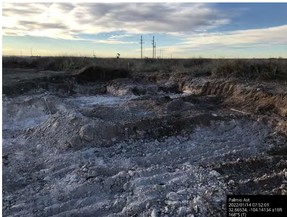
Further exaction in pasture, Spill Area A, viewing to the south.
