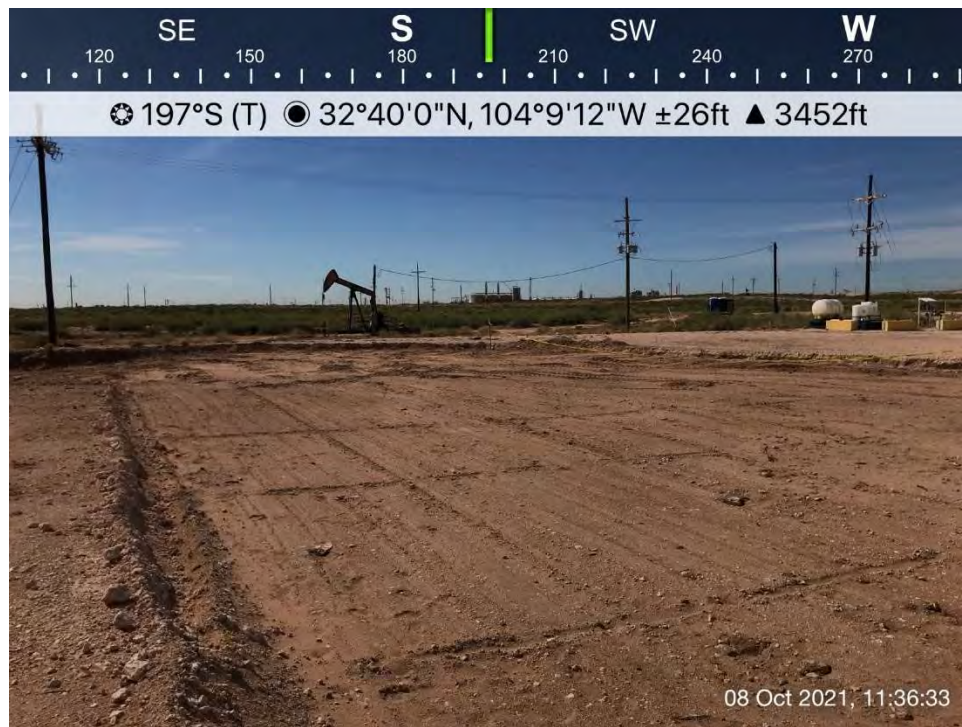
Excavated area on pad, Spill Area D, viewing to the south.
