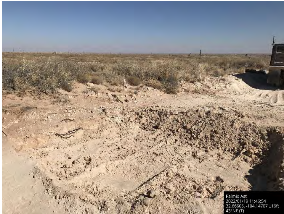
Further Excavation on lease road, Spill Area C, viewing to the northeast.
