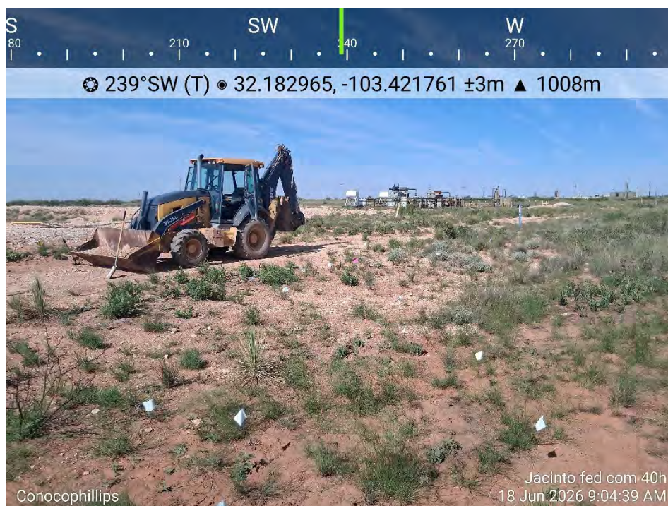
Photo 12: View of rake and shovel work in progress. Backhoe bucket used for soil transport.
