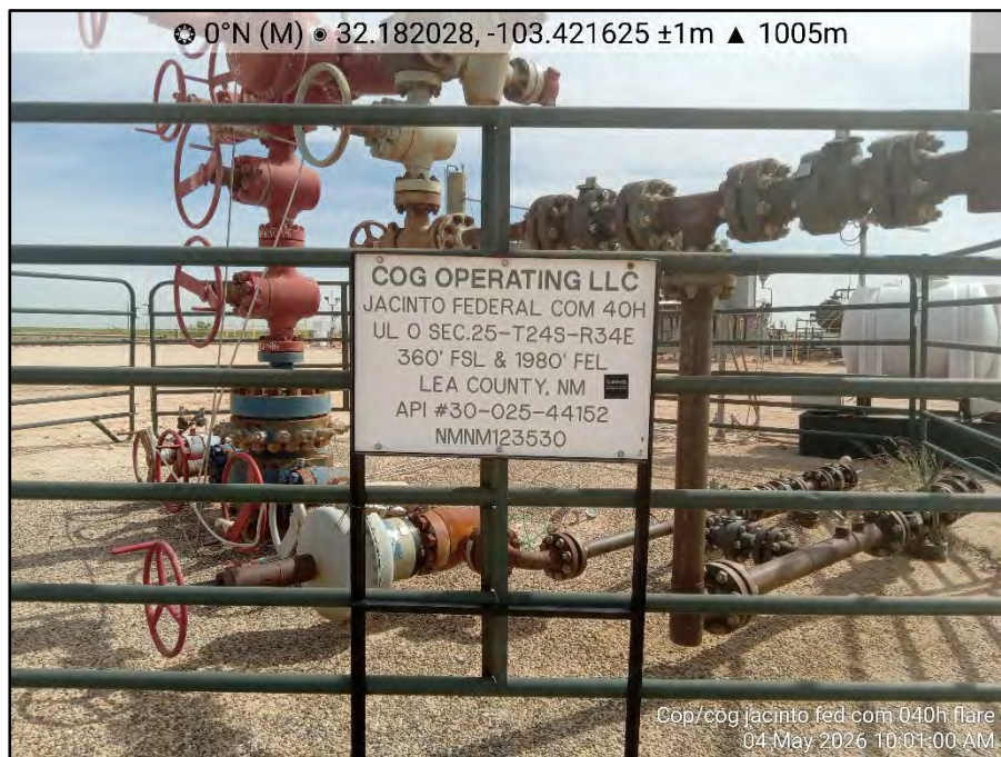
Photo 1: View of the well site signage.
