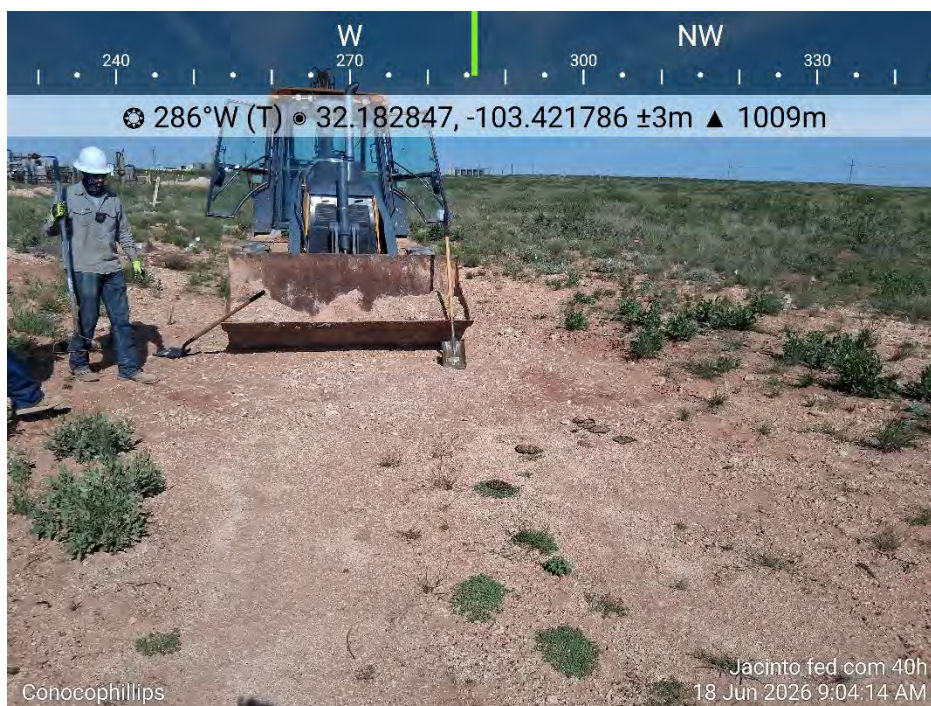
Photo 11: View of rake and shovel work in progress. Backhoe bucket used for soil transport.
