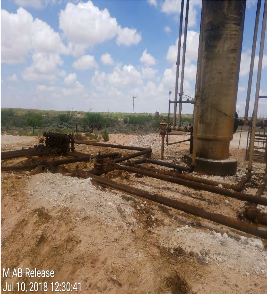
View Northeast– Origin of spill. Release caused by failed gasket on a heater treater.
