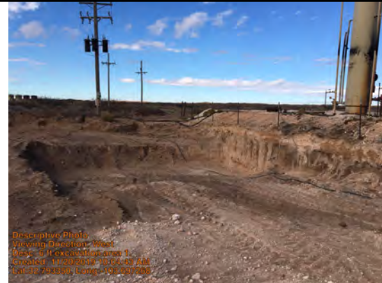
6 ft excavation area 1.
