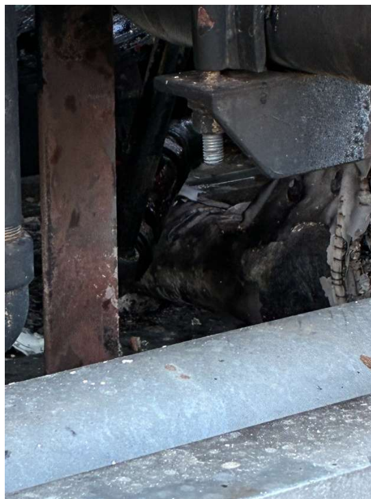
Photo 3 Close-up view of affected area confirming no staining or other indications of a release of fluids.
