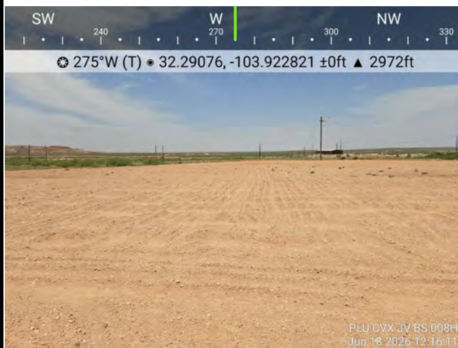
Photograph: 3 Date: 6/18/2026 Description: Backfilled Excavation Area View: West
