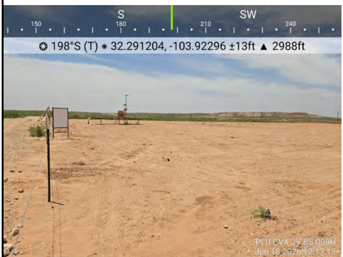
Photograph: 4 Date: 6/18/2026 Description: Backfilled Excavation Area View: South/Southwest
