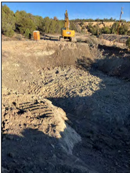
Photograph: 5 Description: Final excavation extent
