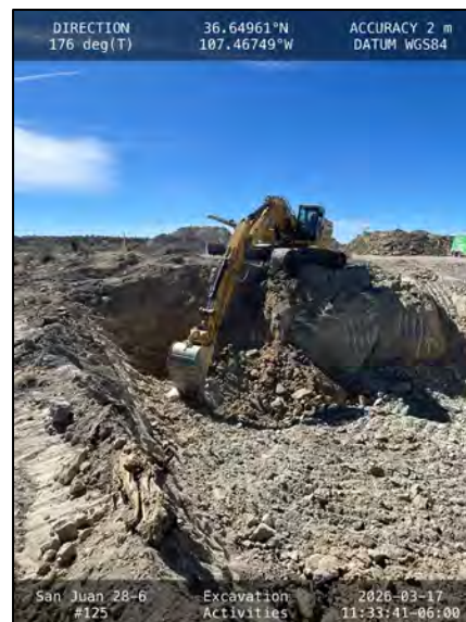
Photograph: 2 Description: Excavation activities
