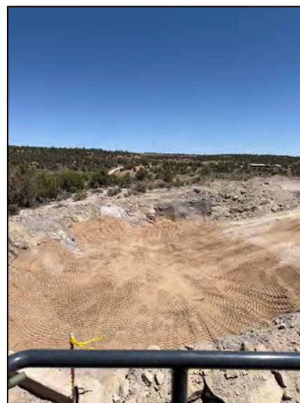
Photograph: 8 Description: Final liner installation
