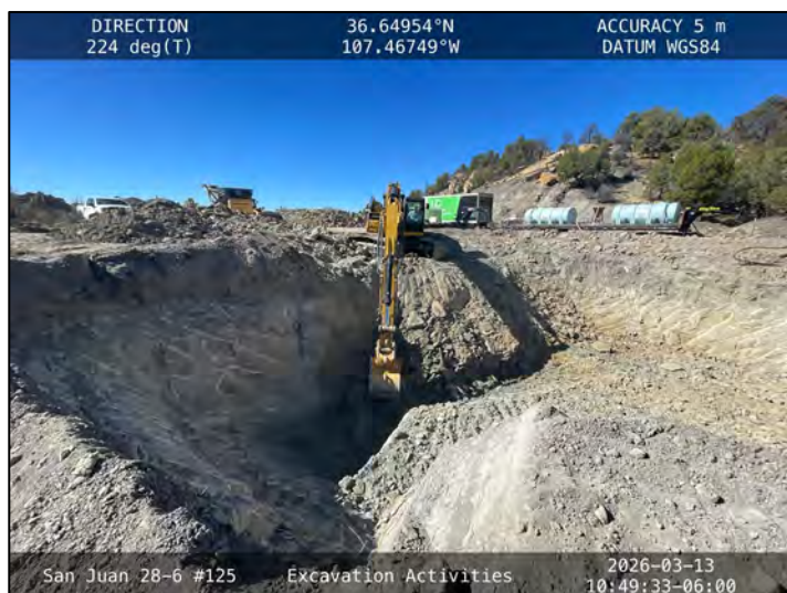
Photograph: 1 Description: Excavation activities
