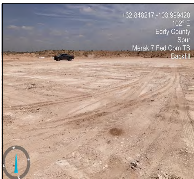
Photo taken post backfill facing east.
