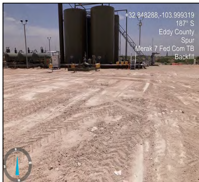
Photo taken post backfill facing south.
