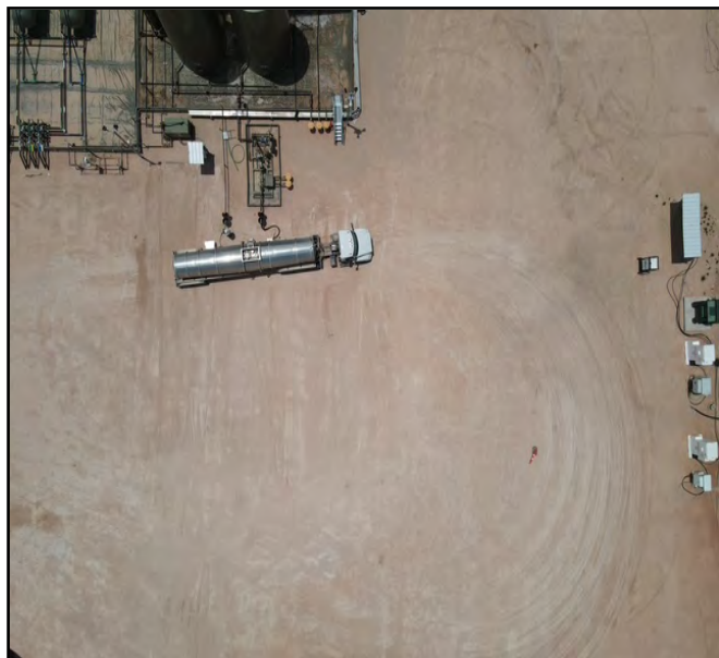
Aerial photo taken post backfill
