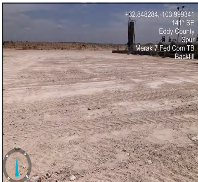
Photo taken post backfill facing southeast.
