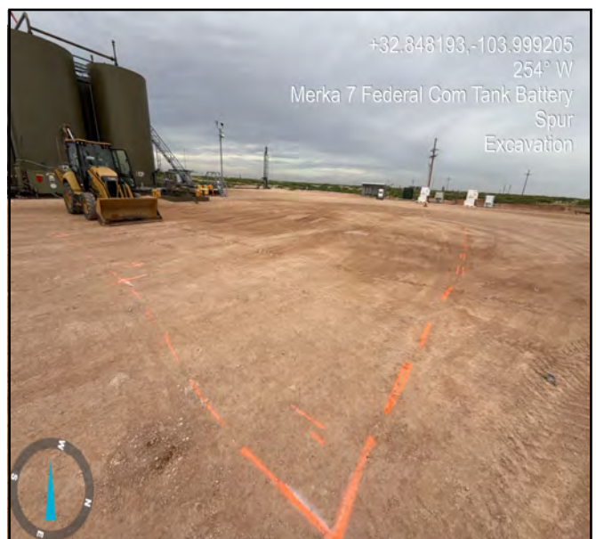
Photo taken pre- excavation process facing west.
