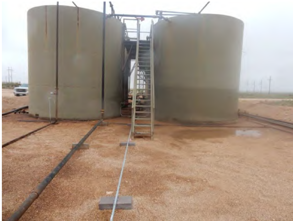
Site Prior to Remediation Viewing South, September 28, 2017
