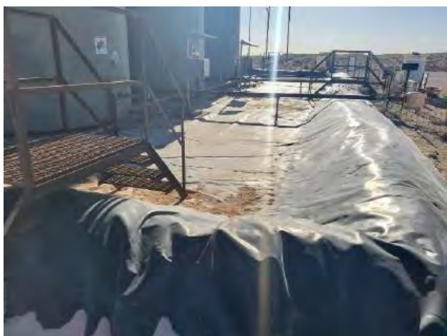
Photograph 3: View of liner corner and base
