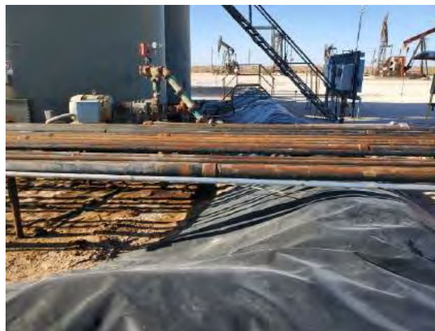
Photograph 4: View of liner with piping
