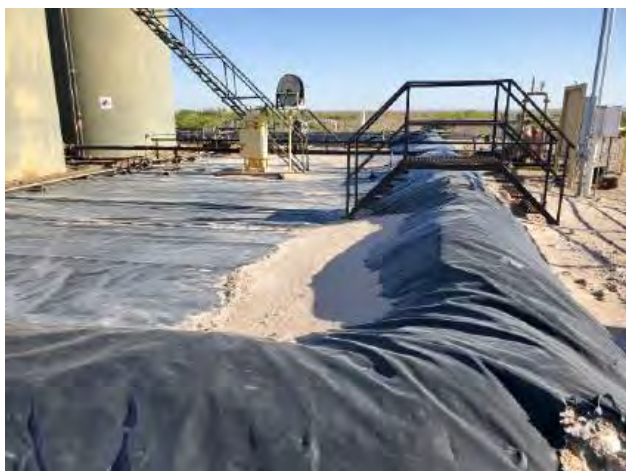
Photograph 2: View of liner corner and base
