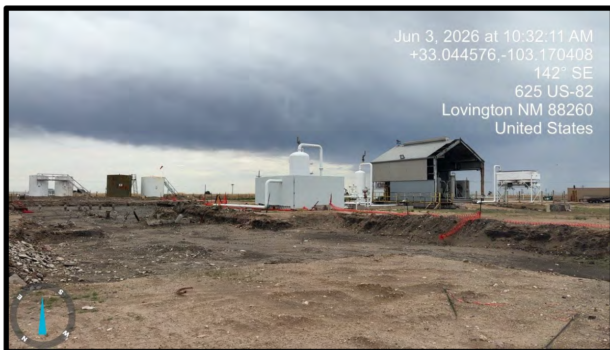
PHOTOGRAPH NO. 8 – An additional view of the anticipated area to be included in the deferral of the remediation request. The area is along the southern extent of the current excavation area.
