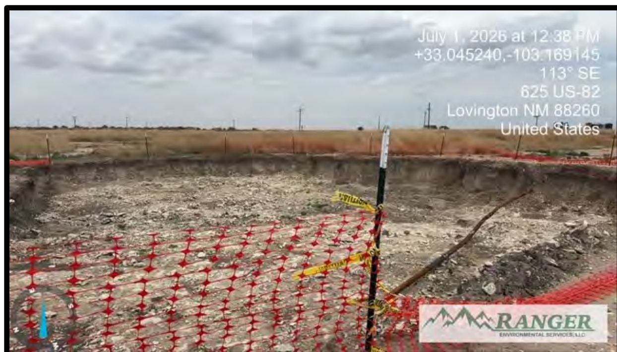
PHOTOGRAPH NO. 9 – A view of the elevated chloride concentration excavation area upon completion of the removal operations in the area.
