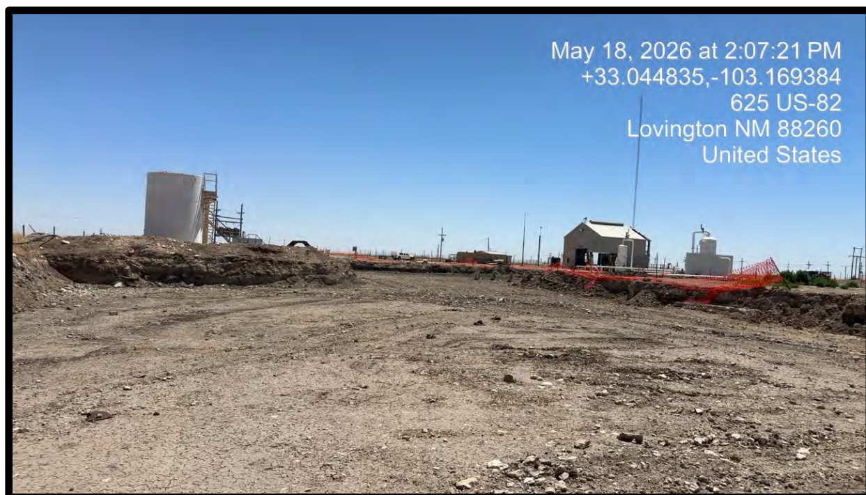
PHOTOGRAPH NO. 7 – An additional view of the remediation area. The view is towards the south.
