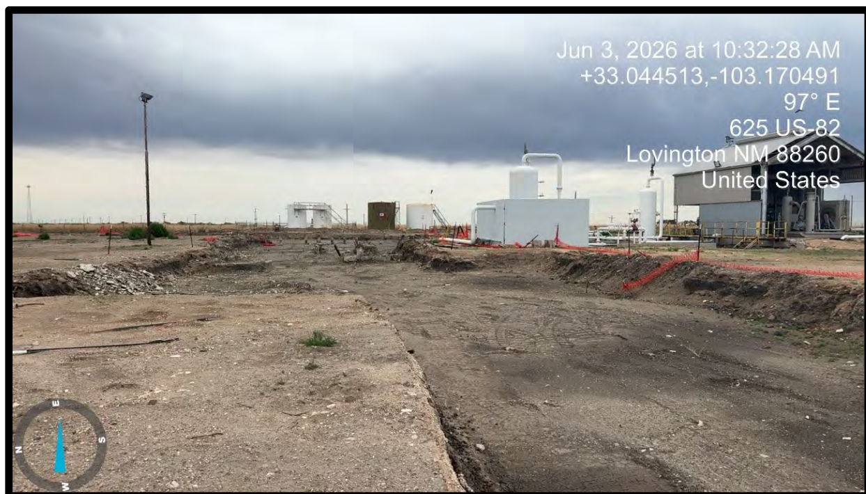
PHOTOGRAPH NO. 2 – A view of the southern portion of the excavation area. The anticipated area of deferral request can be seen on the right-hand side of the photograph.
