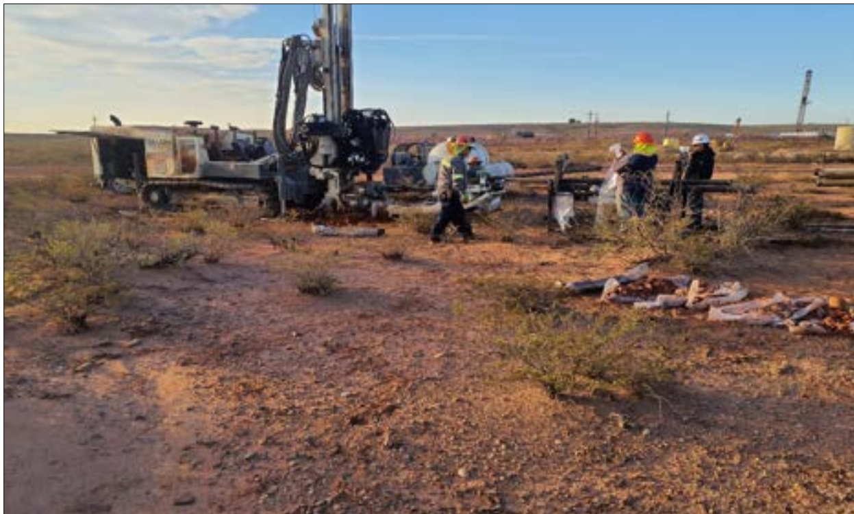
Figure 4-9. Overview of boring progress, approximately 63 m south of LA 194774, facing south (Frame 7354).
