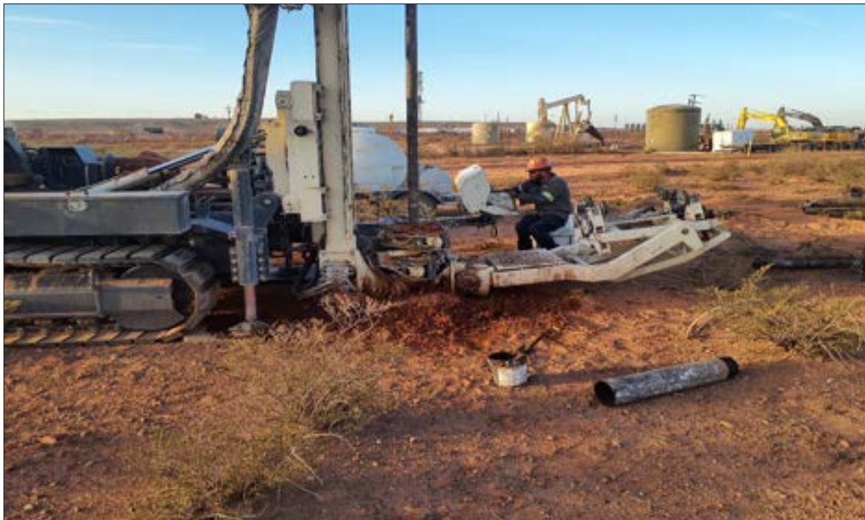
Figure 4-11. Overview of boring in progress, approximately 63 m south of LA 194774, facing southwest (Frame 7601).
