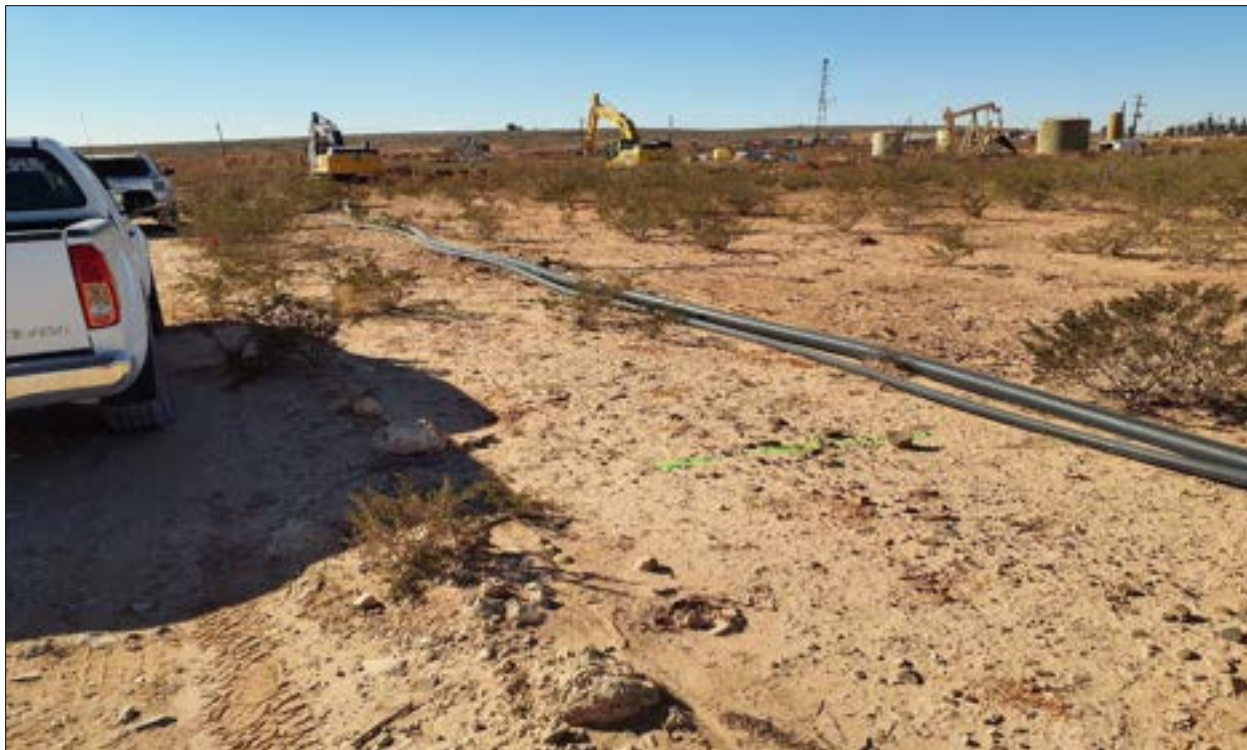
Figure 4-7. Overview of proposed access to drilling locations south of LA 194774, facing southwest (Frame 3302).
