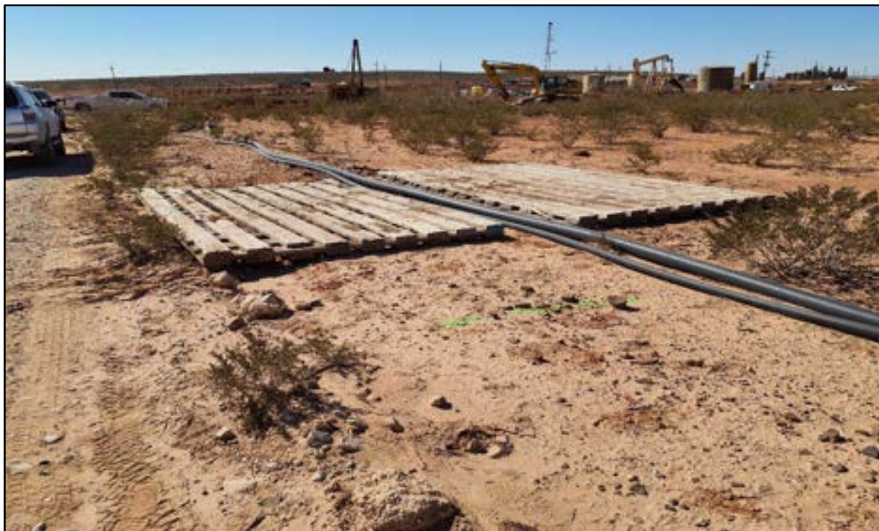
Figure 1-5. Overview of southern access to bore hole locations, avoiding LA 194774, facing southwest (Frame 7766).
