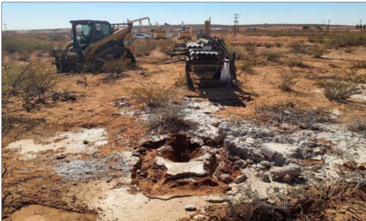
Figure 4-8. Overview of finished bore hole, located approximately 58 m southwest of LA 194774, facing south (Frame 2943).
