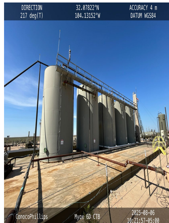
Photo 2 View of containment facing southwest.
