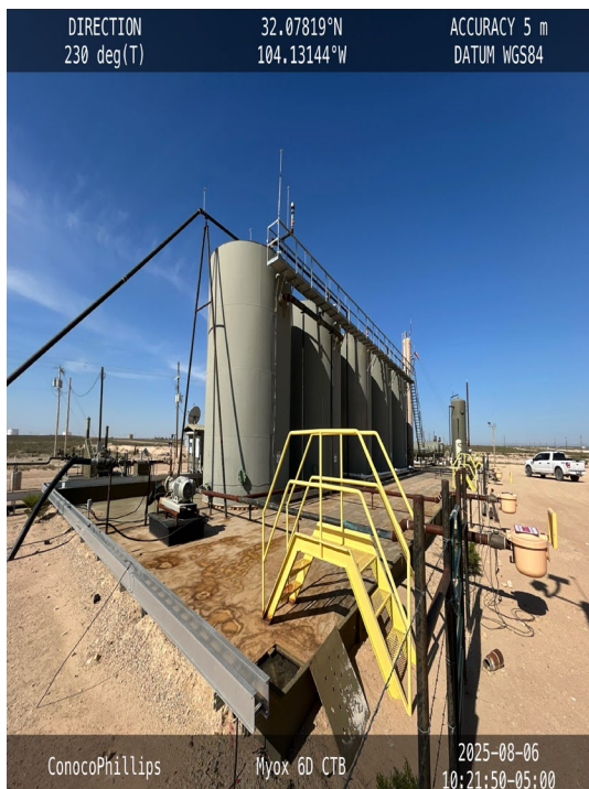
Photo 1 View of containment facing southwest.
