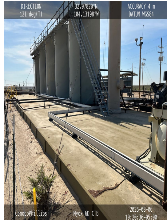
Photo 2 View of containment facing southeast.
