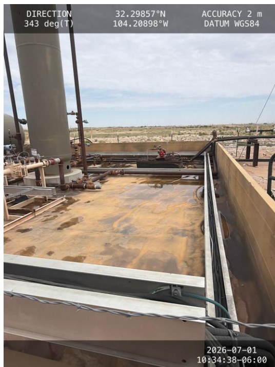
Photo 1 View of the liner corner of the containment area facing north northwest. Residual water from rainfall event.
