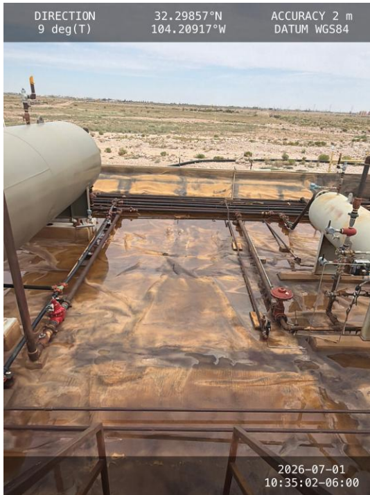
Photo 5 View of the liner in containment area facing north. Residual water from rainfall event.
