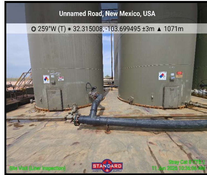
View of Secondary Containment
