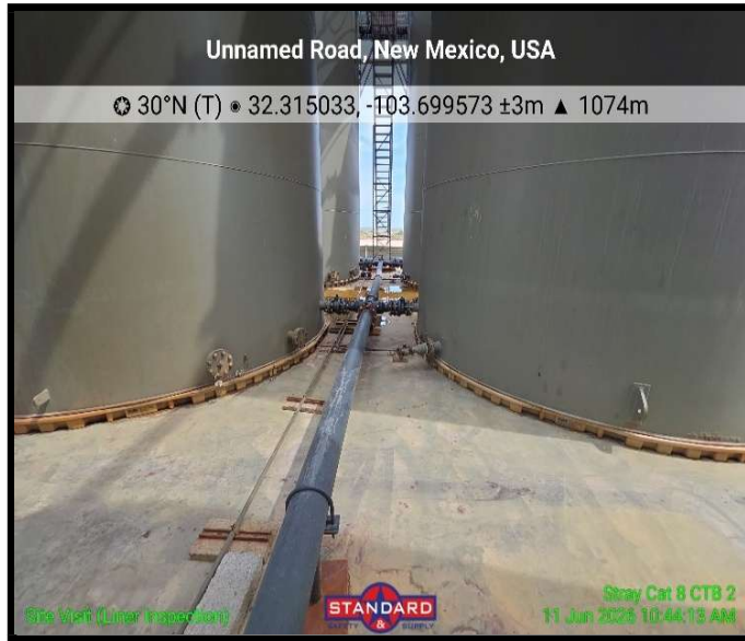
View of Secondary Containment
