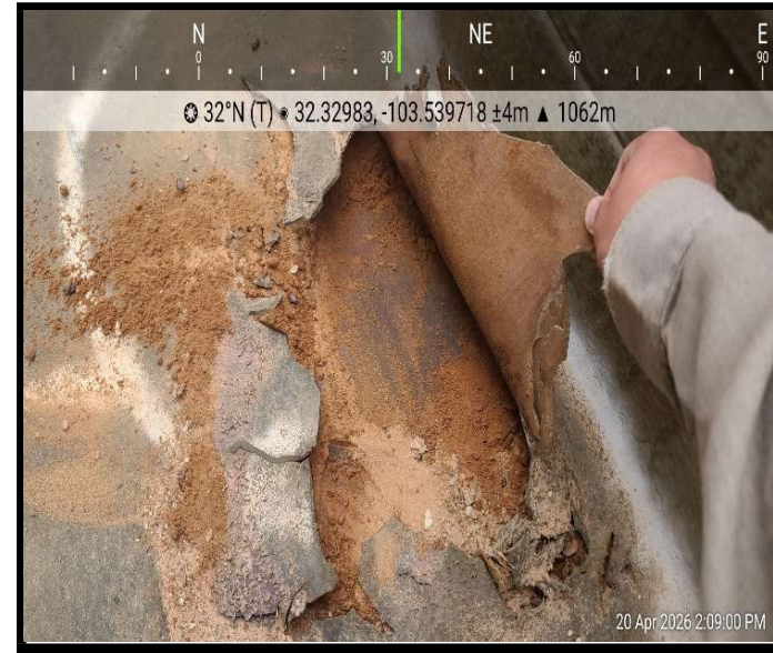
View of secondary liner under primary liner
