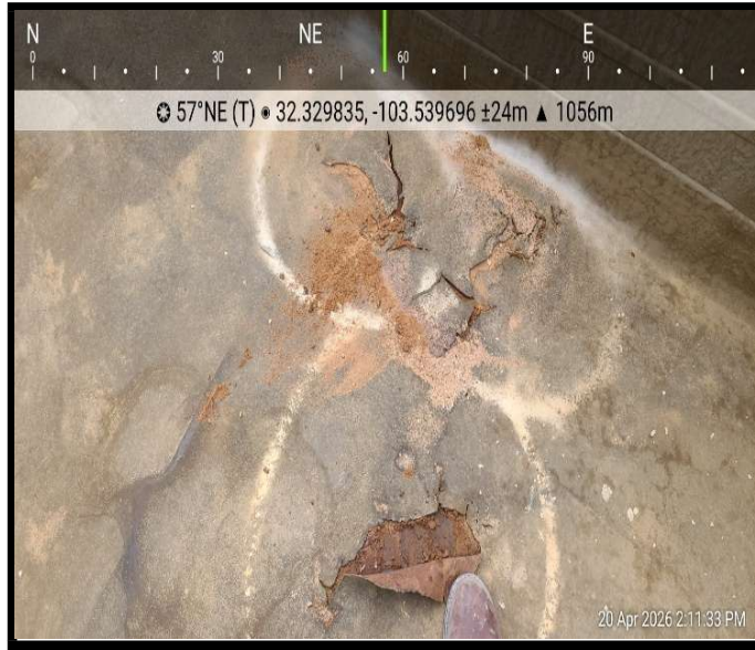
View of secondary liner under primary liner
