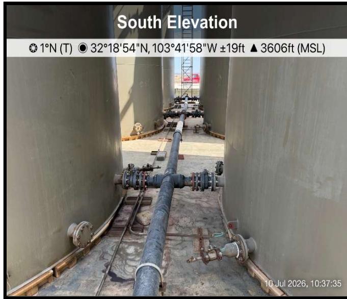
View of Secondary Containment
