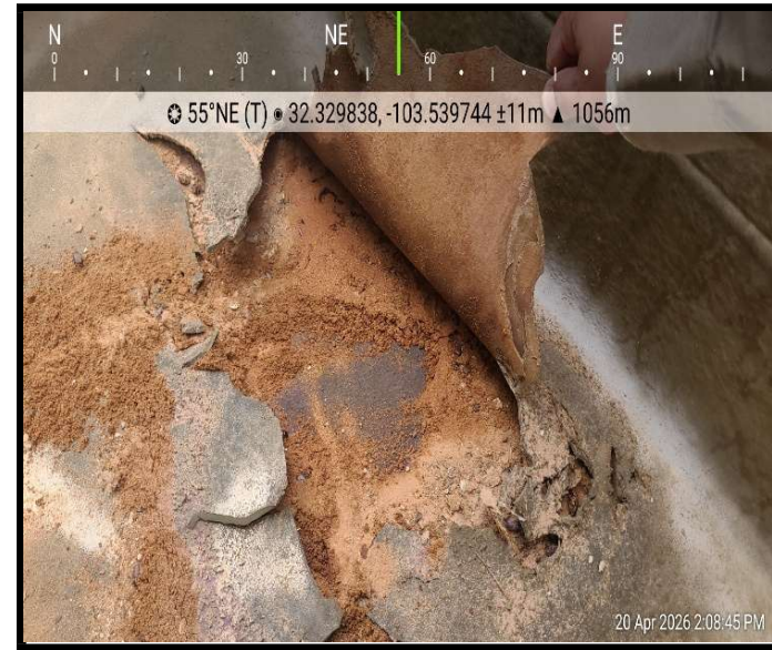
View of secondary liner under primary liner
