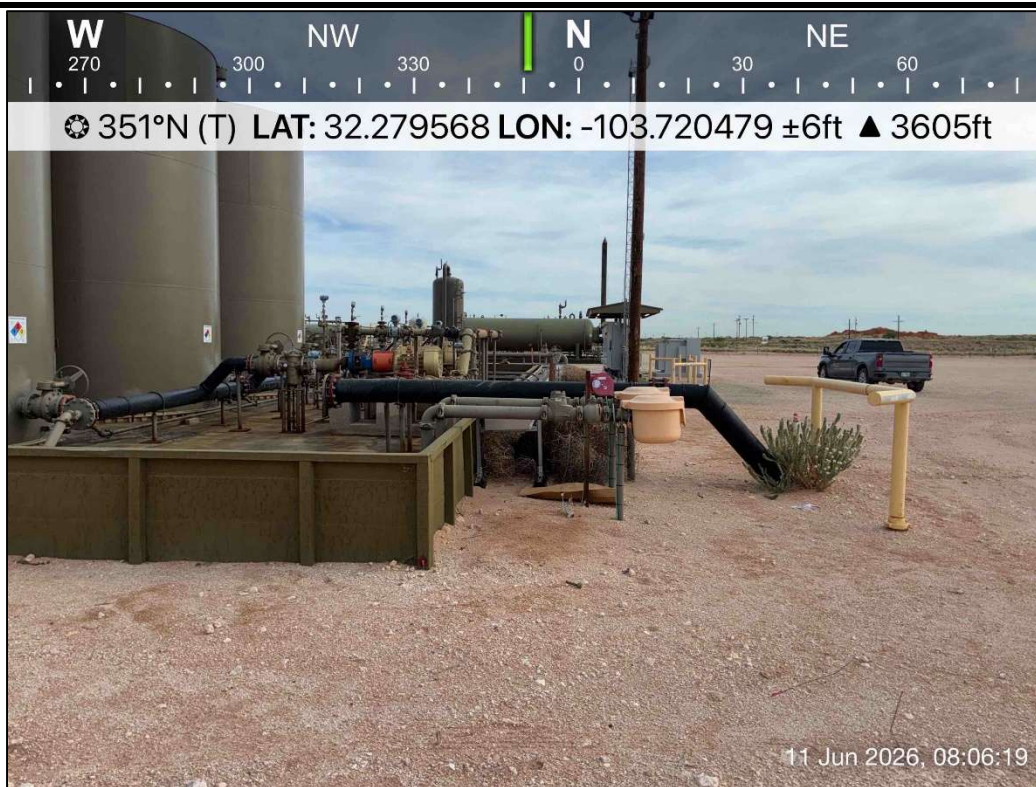
PHOTO 5: Northern view outside of containment during liner inspection activities. 6/11/2026
