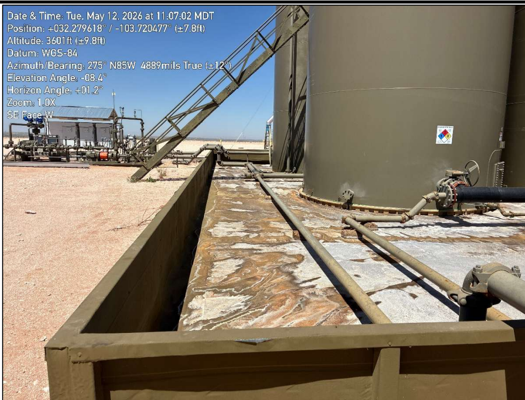
PHOTO 2: Northwestern view during initial site assessment. 5/12/2026
