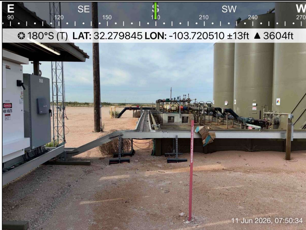
PHOTO 3: Southern view outside of containment during liner inspection activities. 6/11/2026
