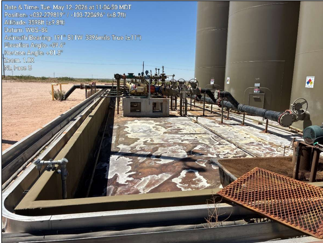
PHOTO 1: Southwestern view during initial site assessment. 5/12/2026
