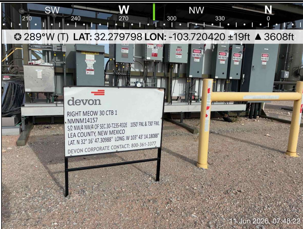
PHOTO 22: Western view of location sign. 6/11/2026
