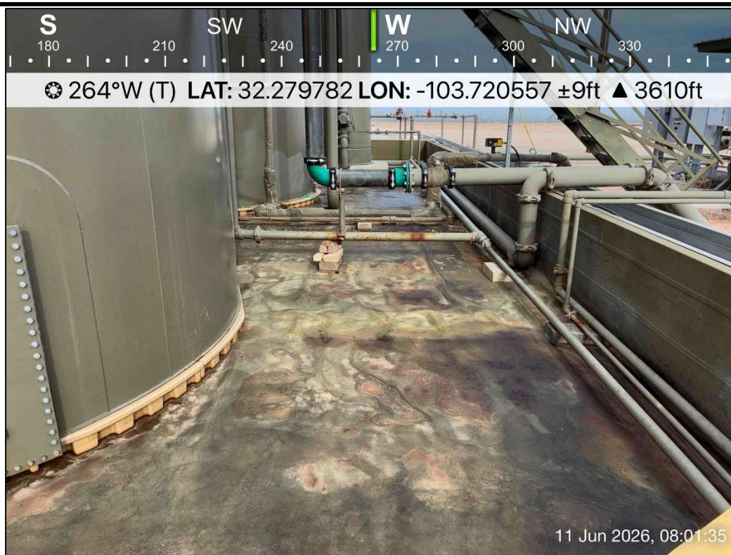
PHOTO 10: Western view during liner inspection activities. 6/11/2026
