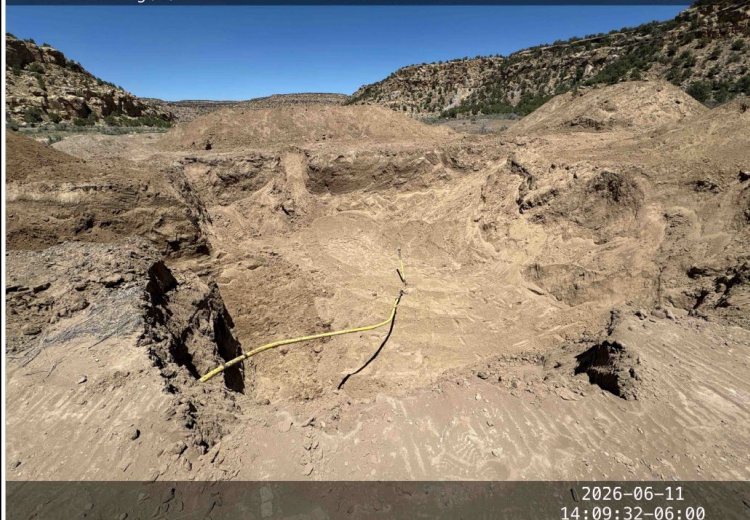
Photograph: 5 Date: 6/11/2026 Description: Northeast view of excavation View: Northeast
