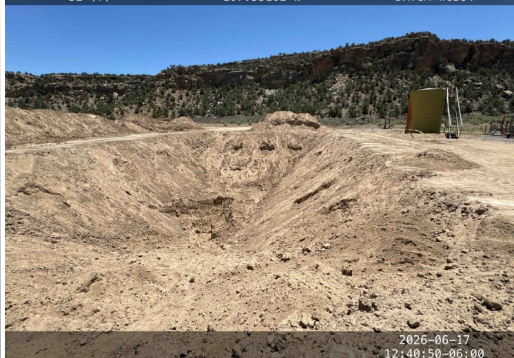
Photograph: 6 Date: 09/29/2025 Description: Southeast view of excavation View: Southeast
