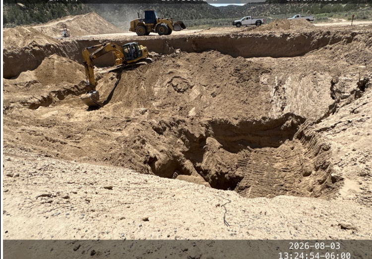
Photograph: 7 Date: 8/03/2026 Description: Excavation activities View: Southwest
