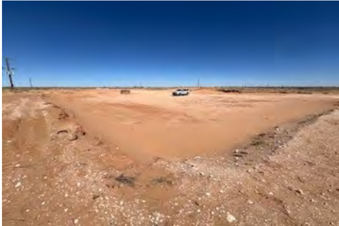
View to NE of excavation (3/13/26).
