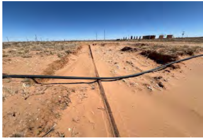
View to SE of excavation (3/13/26).
