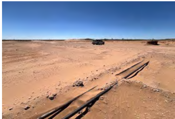
View to SW of excavation (3/13/26).
