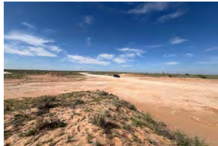
View to SW of excavation (6/24/26).
