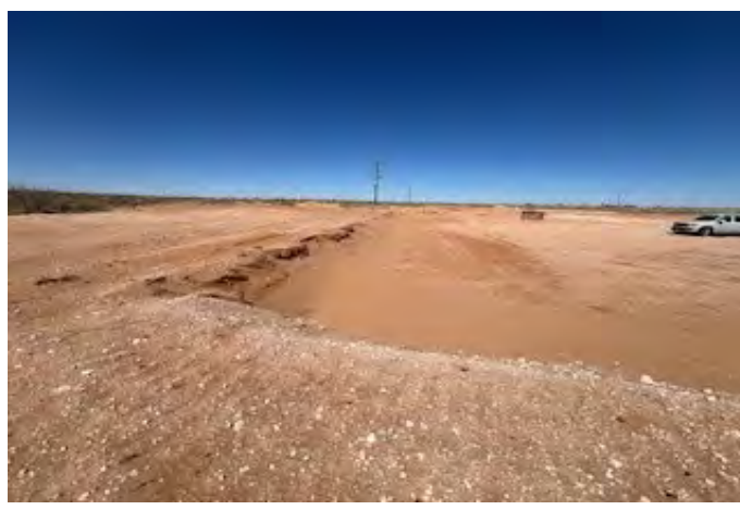
View to N of excavation (3/13/26).
