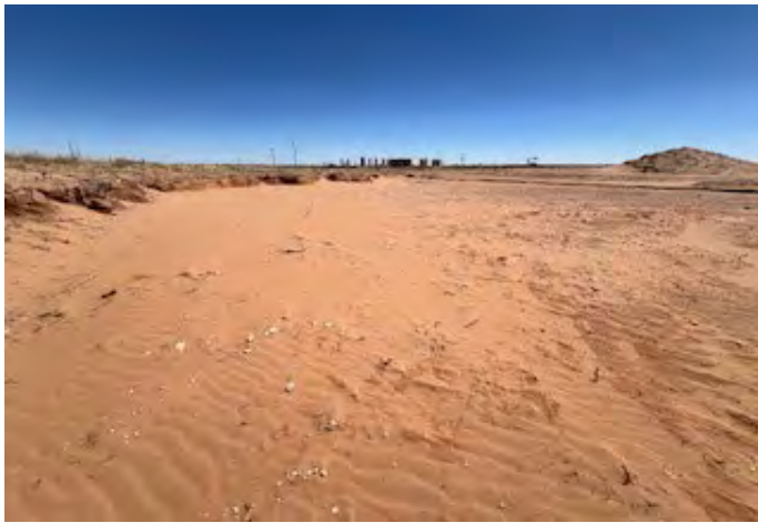
View to SE of excavation (3/13/26).
