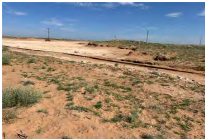
View to NW of excavation (6/24/26).
