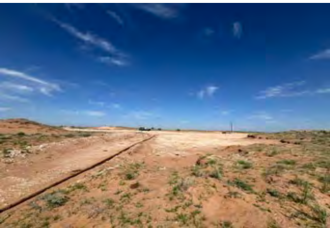
View to W of excavation (6/24/26).
