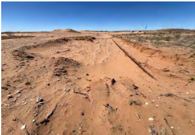
View to NW of excavation (3/13/26).
