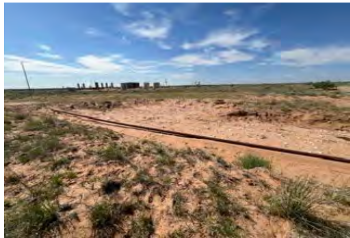
View to SE of excavation (6/24/26).
