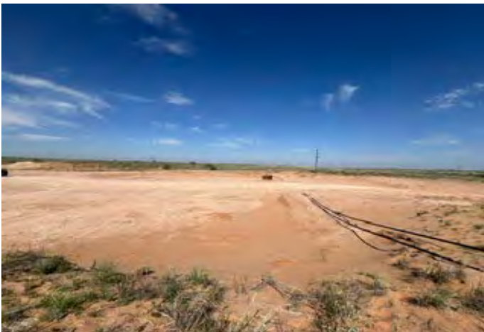
View to W of excavation (6/24/26).
