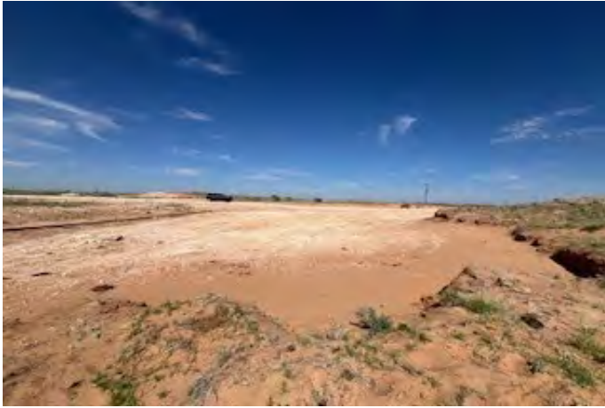
View to W of excavation (6/24/26).
