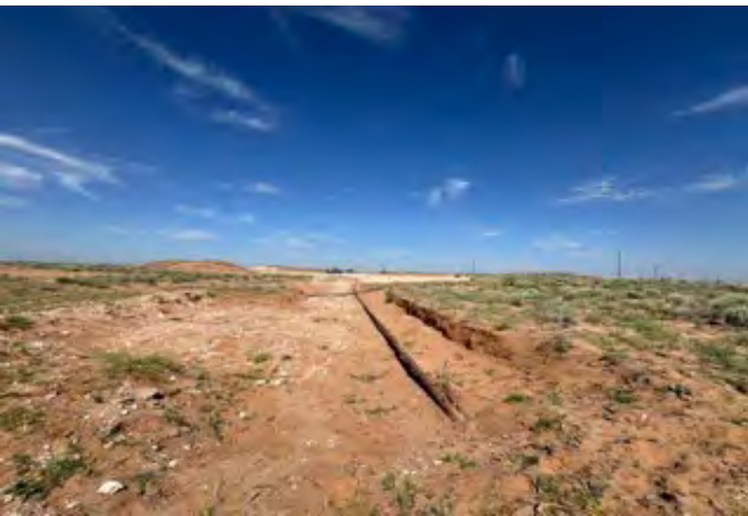
View to W of excavation (6/24/26).
