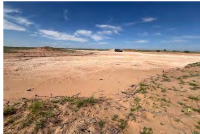
View to SW of excavation (6/24/26).
