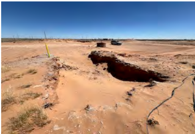
View to E of excavation (3/13/26).
