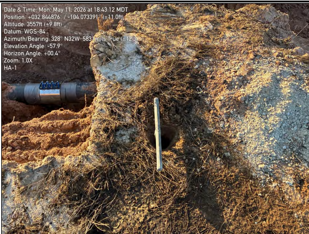
PHOTO 4: Northwestern view during delineation activities. 5/11/2026
