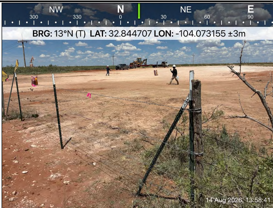
PHOTO 11: Northeastern view following restoration activities. 8/14/2026
