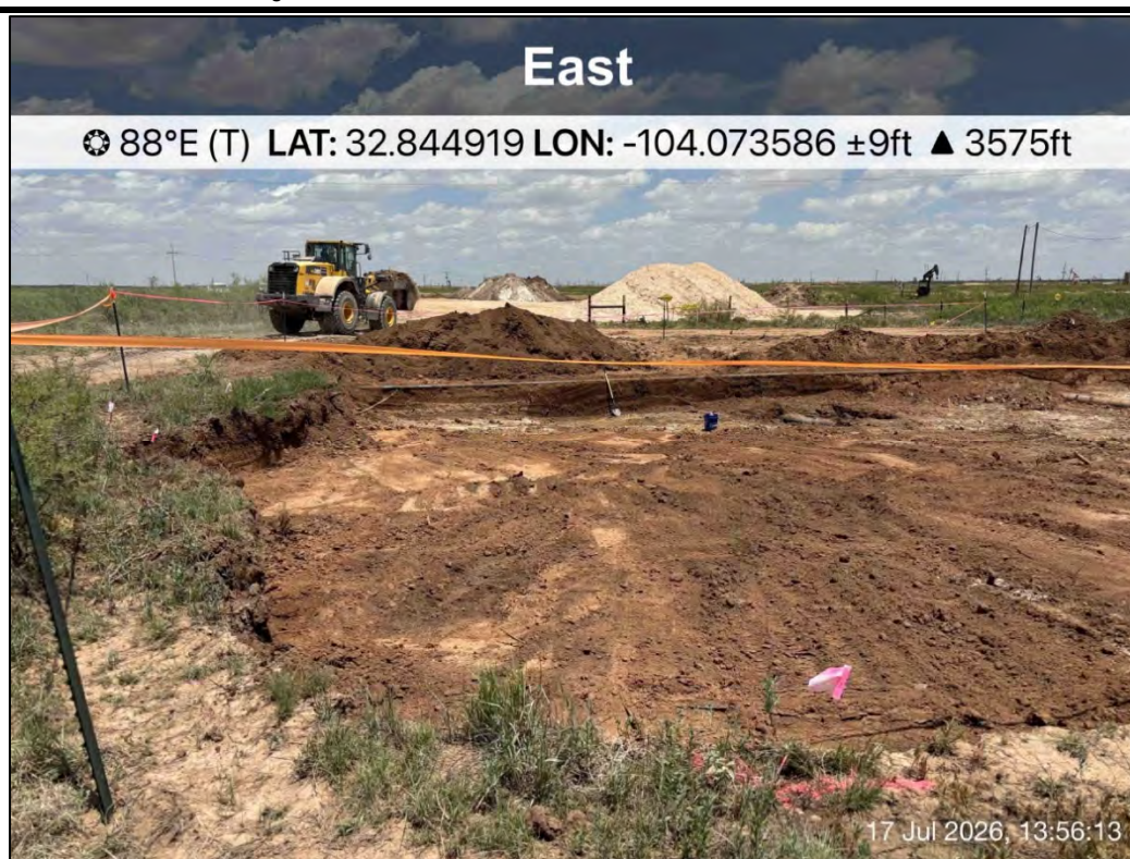
PHOTO 6: Eastern view of excavation extent. 7/17/2026
