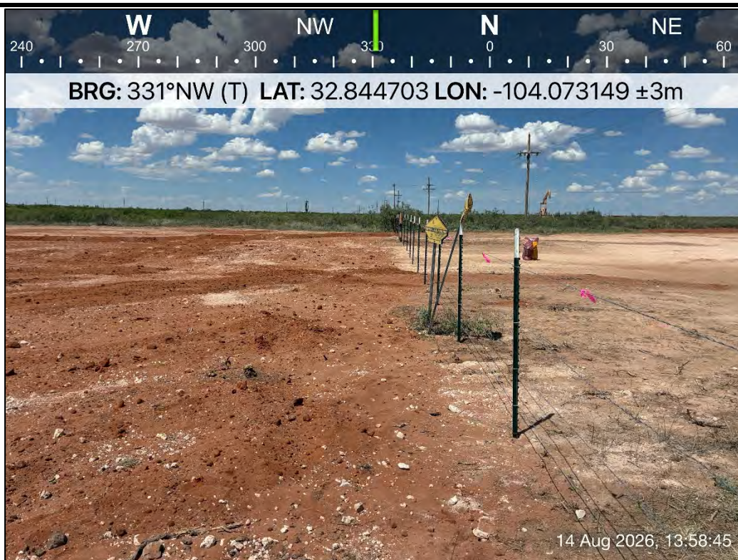
PHOTO 12: Northwestern view following restoration activities. 8/14/2026
