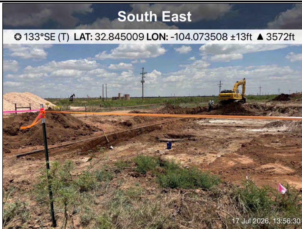
PHOTO 7: Southeastern view of excavation extent. 7/17/2026
