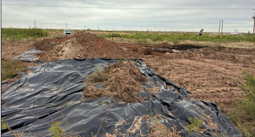
PHOTO 1: Northeastern view during initial site assessment activities. 5/5/2026
