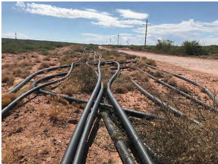
3 N point looking S on E side
