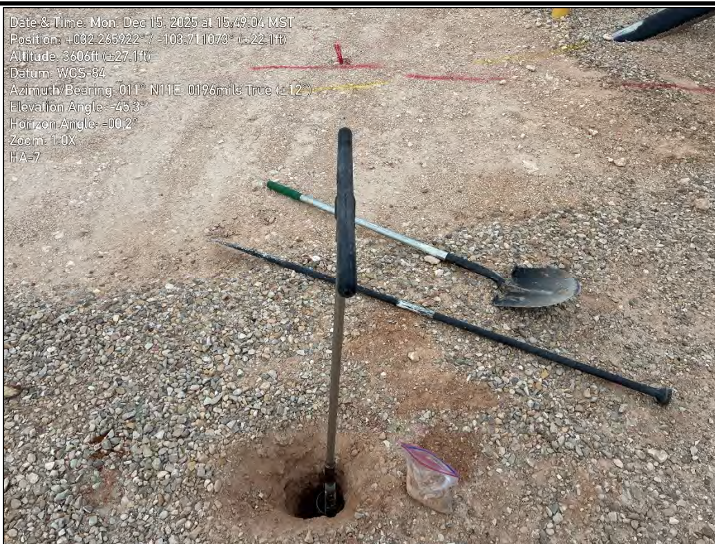
PHOTO 4: Northeastern view during delineation activities of nAPP2525125732. 12/15/2025
