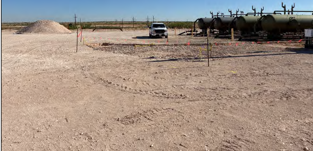
PHOTO 15: Northeastern view of excavation extent. 5/18/2026
