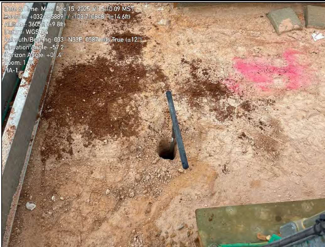
PHOTO 3: Northeastern view during delineation activities of nAPP2525125732. 12/15/2025
