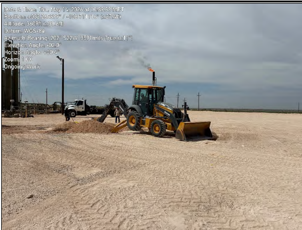
PHOTO 12: Southwestern view during excavation activities. 5/14/2026
