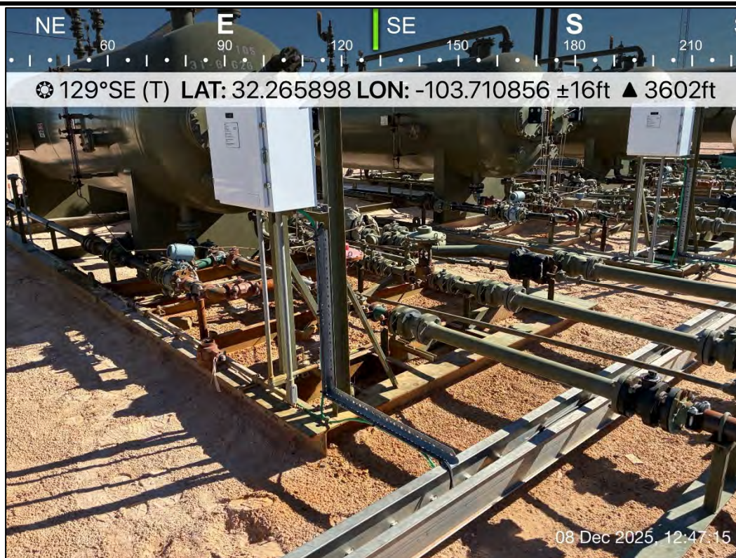
PHOTO 1: Southeastern view during site assessment activities for nAPP2525125732. 12/8/2025
