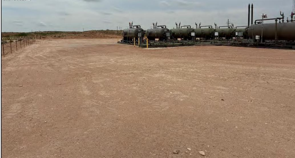
PHOTO 16: Southeastern view following restoration activities. 6/3/2026
