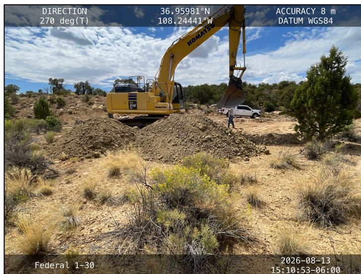
Photograph: 16 Date: 08/13/2026 Description: Clean imported backfill, sampled as SP01/
