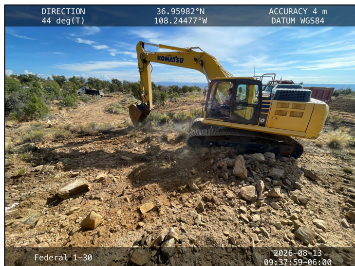
Photograph: 9 Date: 08/13/2026 Description: Excavation activities: removing stained soil and flora from release footprint. View: Northeast
