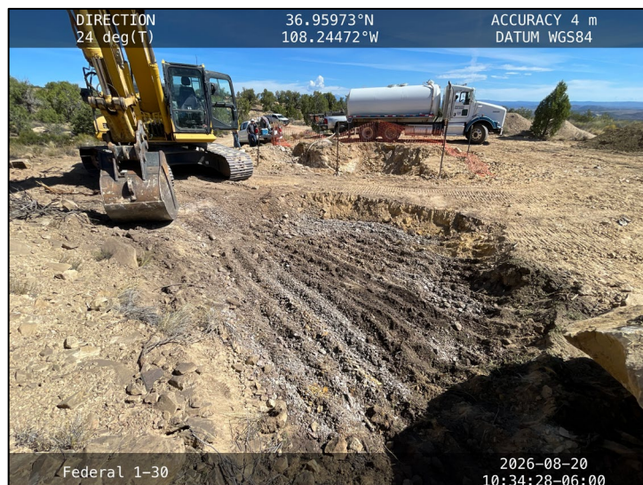
Photograph: 14 Date: 08/20/2026 Description: Removal of the exceeding sample FS08. Newly exposed sidewalls and floor sampled as FS08A.
