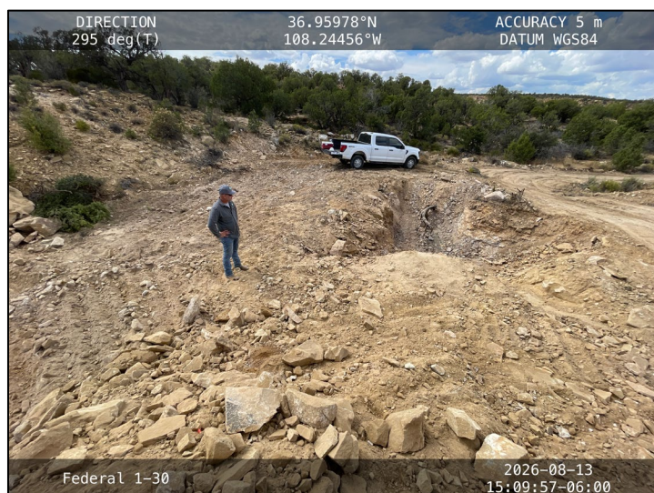
Photograph: 13 Date: 08/13/2026 Description: Excavation extent as of August 13 th , 2026.
