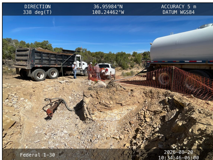
Photograph: 15 Date: 08/20/2026 Description: Pipeline cutting, pigging, and capping activities.
