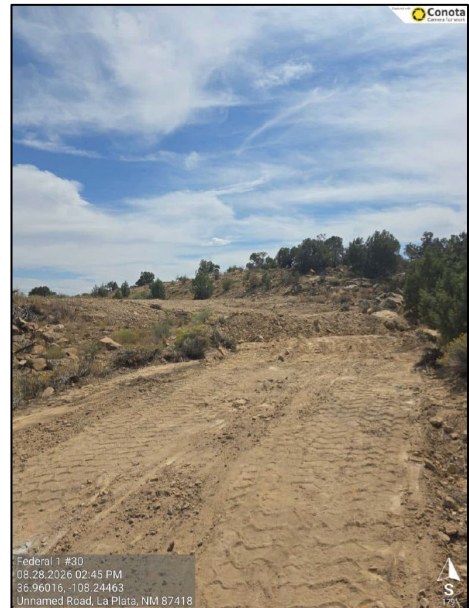
Photograph: 16 Date: 08/28/2026 Description: Reclamation and reseeding activities. View: West
