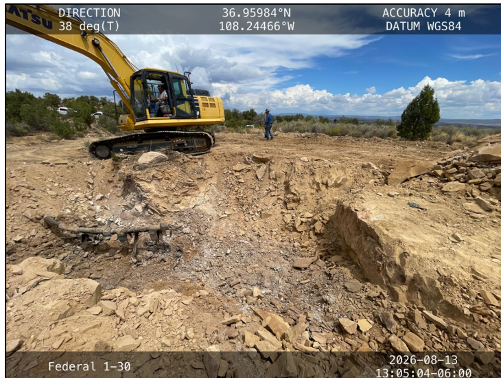
Photograph: 12 Date: 08/13/2026 Description: Excavation activities: exposing the pipeline for repair. Sampled as FS01, FS02, SW01, and SW02. View: Northeast
