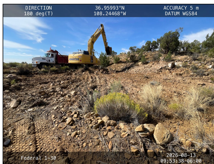
Photograph: 10 Date: 08/13/2026 Description: Excavation activities: removing stained soil and flora from release footprint. View: South
