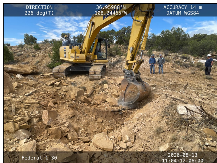
Photograph: 11 Date: 08/13/2026 Description: Excavation activities: exposing the pipeline for repair. View: Southwest
