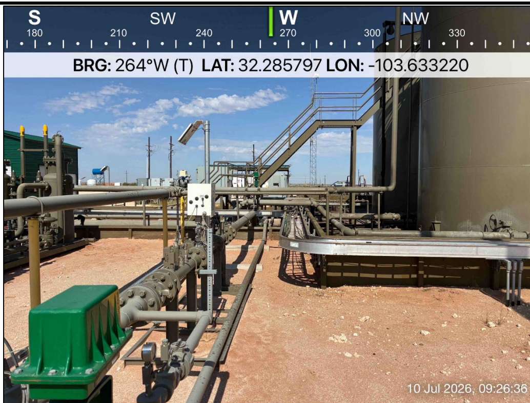
PHOTO 6: Western view outside of containment during liner inspection activities. 7/10/2026
