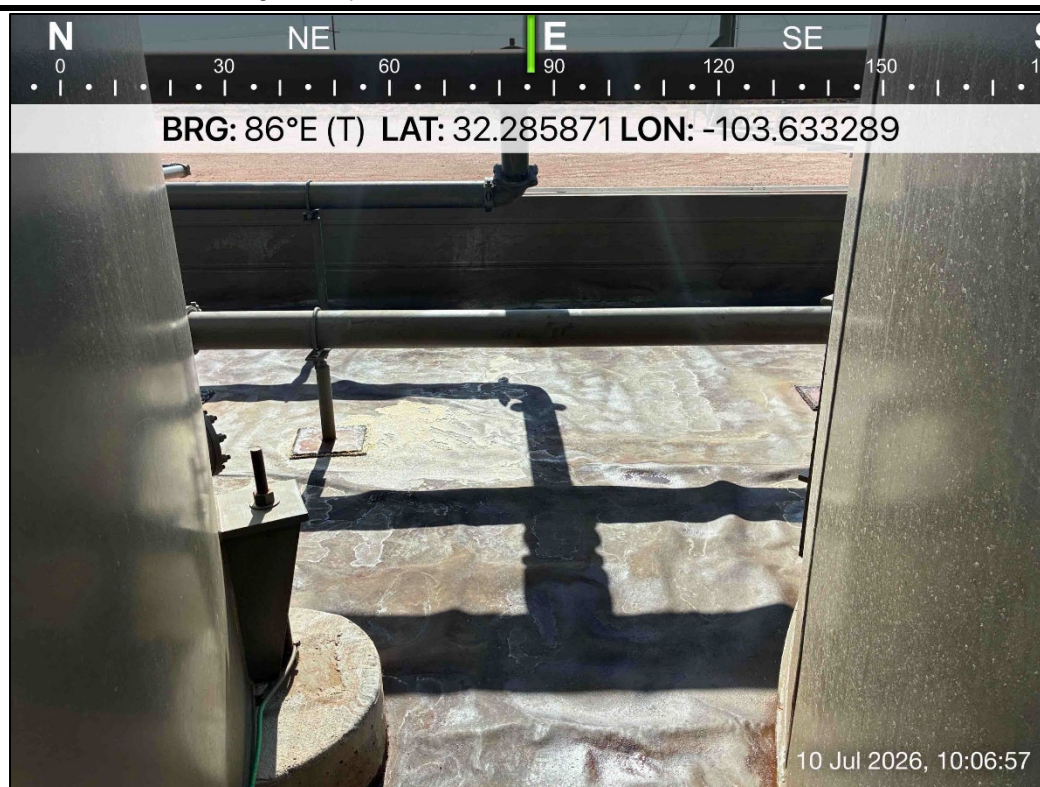
PHOTO 12: Eastern view during liner inspection activities. 7/10/2026
