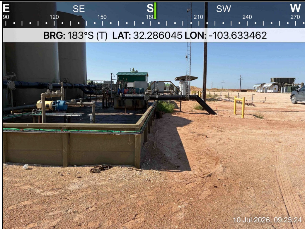
PHOTO 3: Southern view outside of containment during liner inspection activities. 7/10/2026
