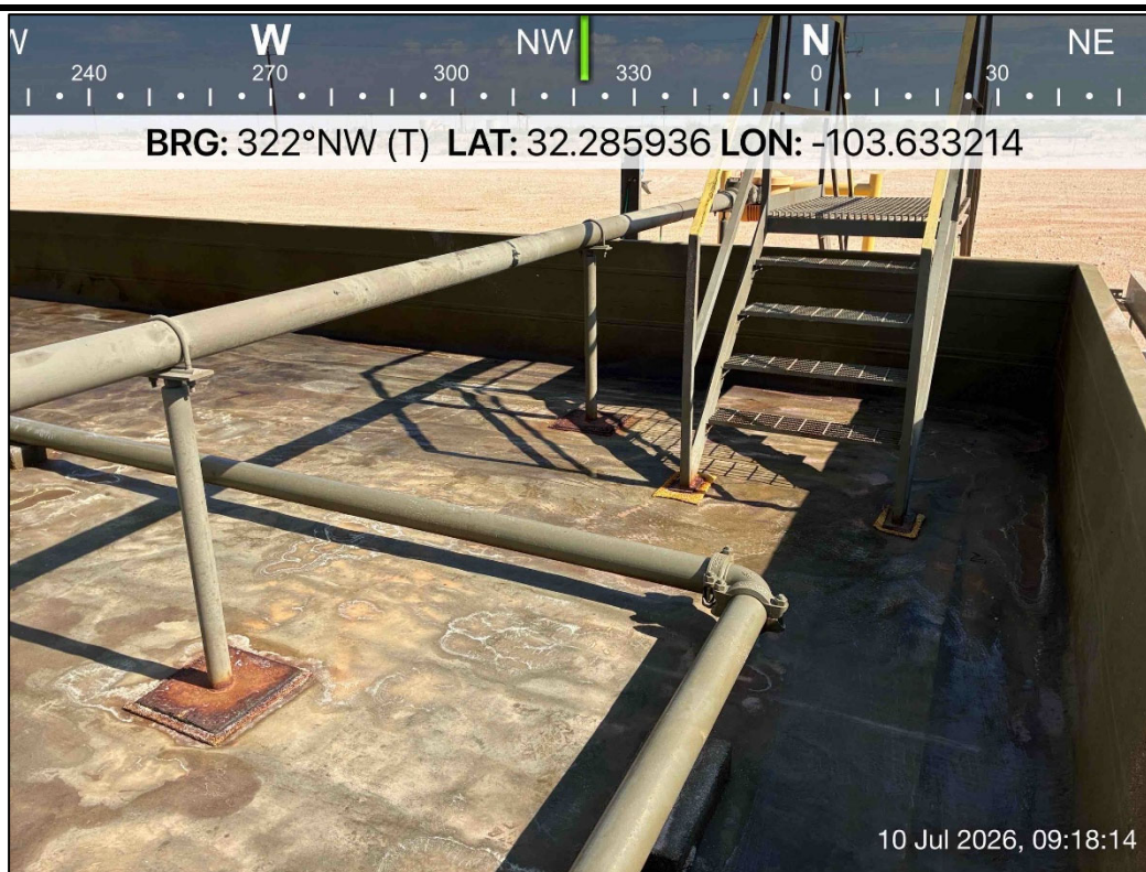
PHOTO 19: Northwestern view during liner inspection activities. 7/10/2026
