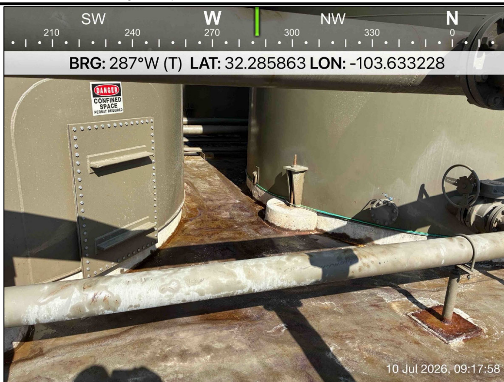
PHOTO 18: Western view during liner inspection activities. 7/10/2026
