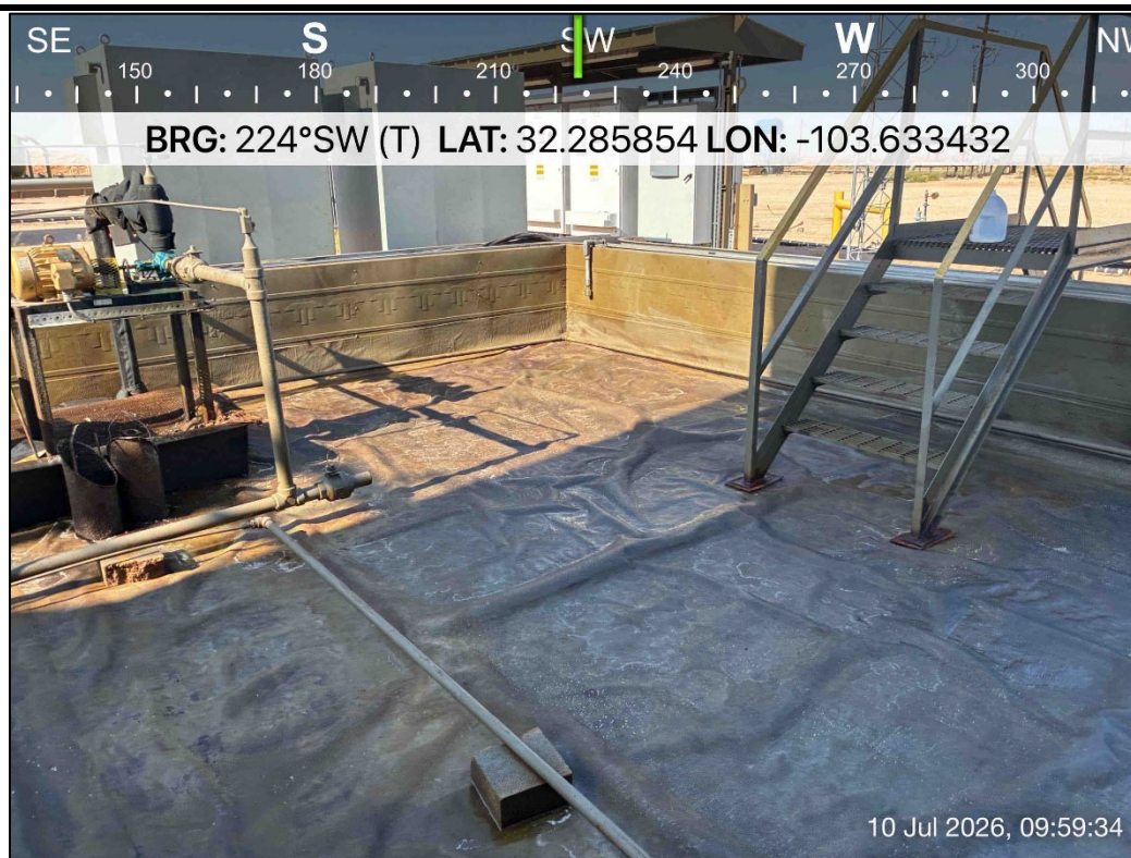
PHOTO 8: Southwestern during liner inspection activities. 7/10/2026
