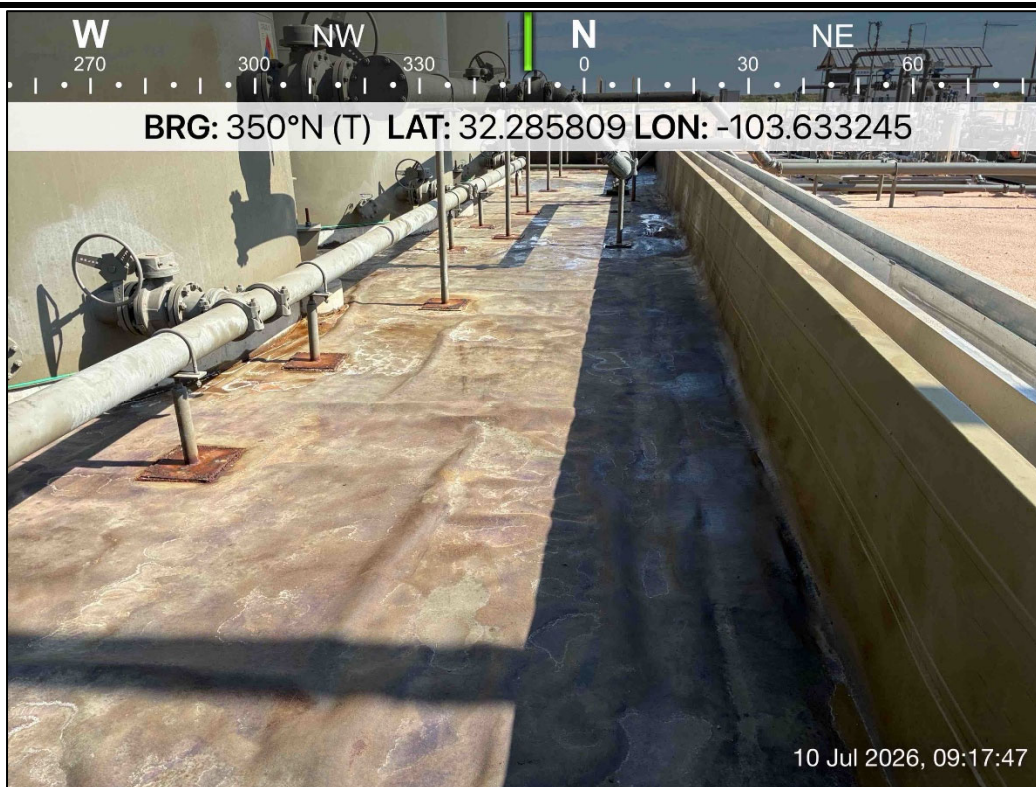
PHOTO 17: Northwestern view during liner inspection activities. 7/10/2026
