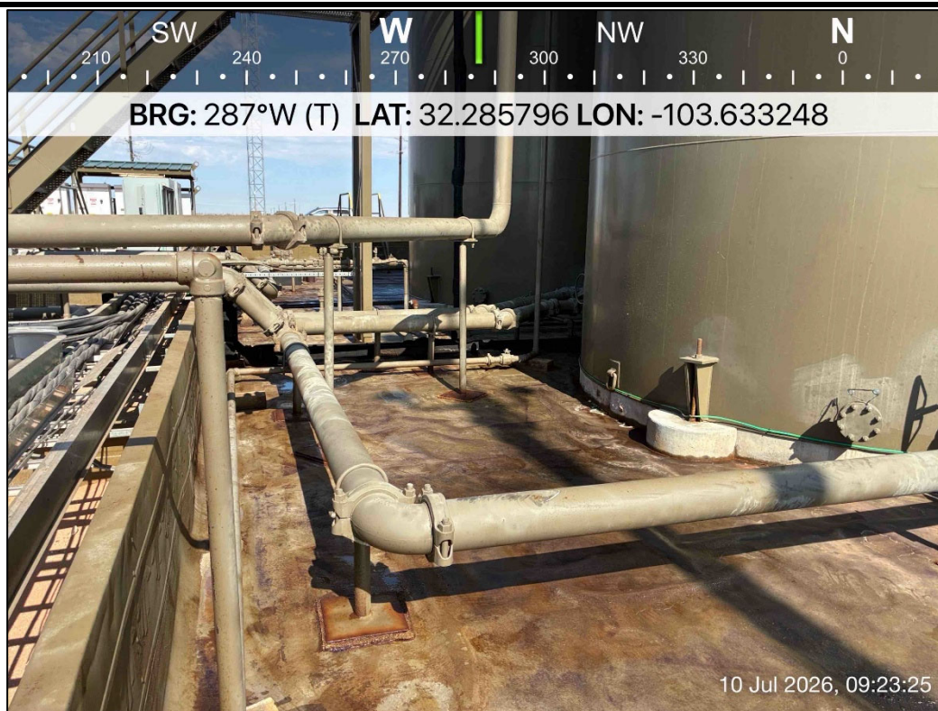
PHOTO 21: Northwestern view during liner inspection activities. 7/10/2026
