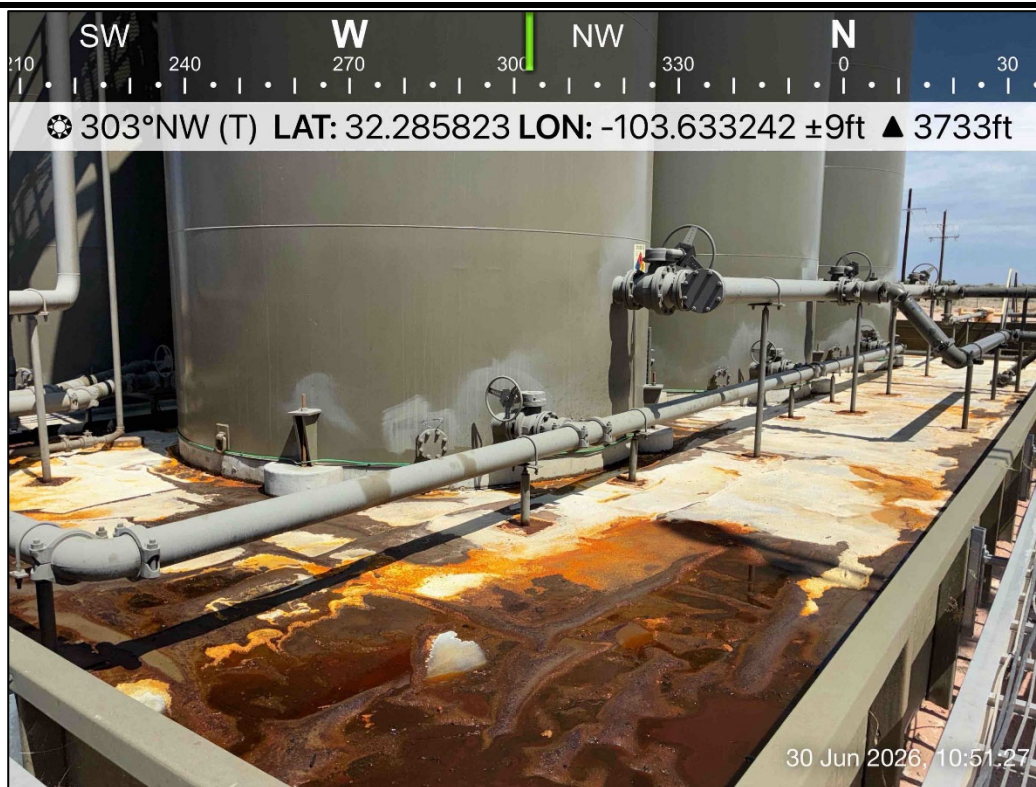
PHOTO 1: Northwestern view during initial site assessment. 6/30/2026
