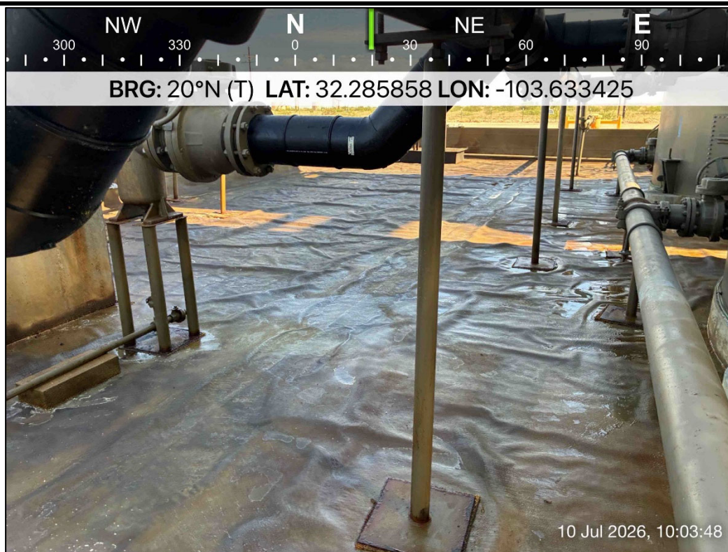
PHOTO 11: Northeastern view during liner inspection activities. 7/10/2026
