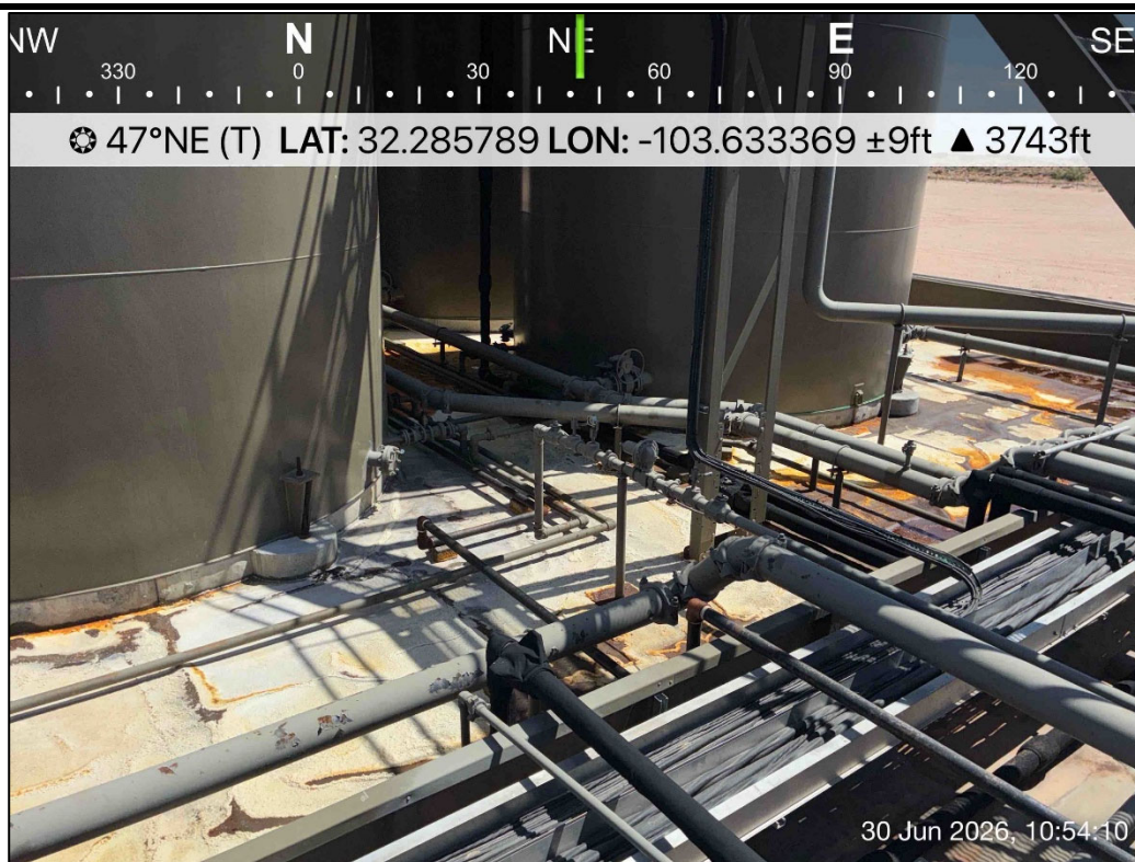
PHOTO 2: Northeastern view during initial site assessment. 6/30/2026
