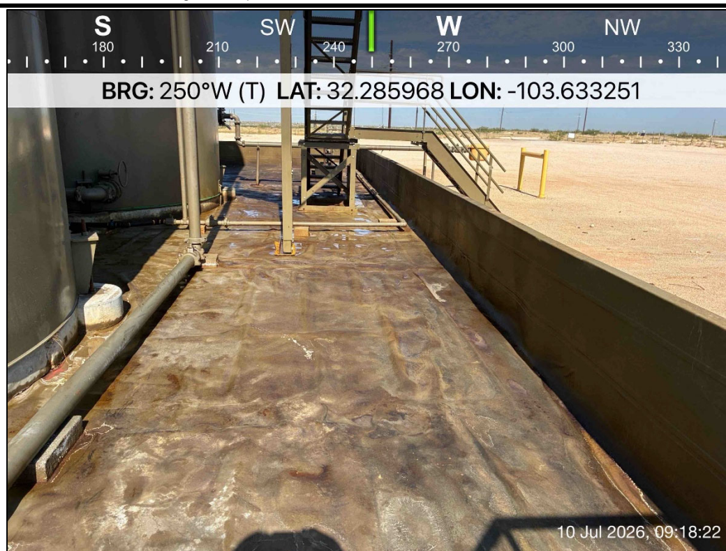
PHOTO 20: Southwestern view during liner inspection activities. 7/10/2026
