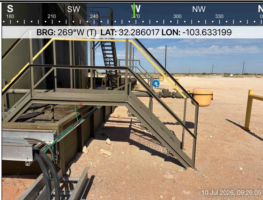
PHOTO 5: Western view outside of containment during liner inspection activities. 7/10/2026
