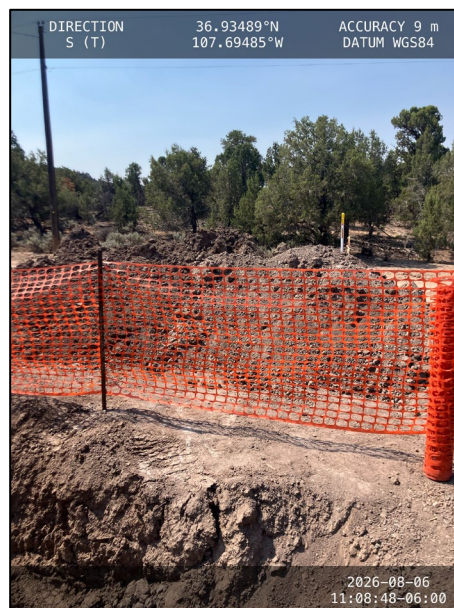
Photograph: 8 Date: 08/06/2026 Description: Removed impacted soil.
