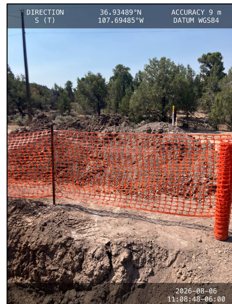
Photograph: 8 Date: 08/06/2026 Description: Removed impacted soil.
