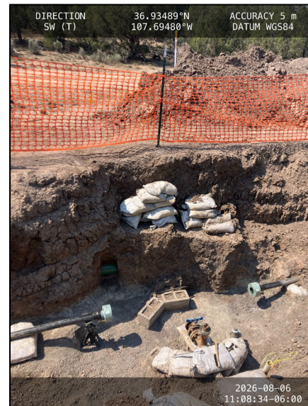
Photograph: 6 Date: 08/06/2026 Description: Excavation and exposed pipelines.
