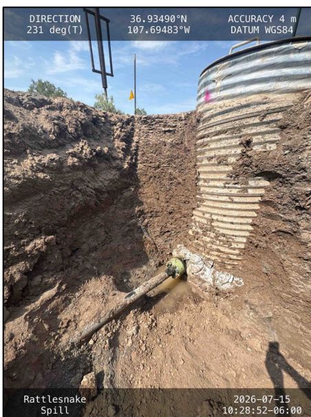
Photograph: 3 Date: 07/15/2026 Description: Excavation extent, exposed and repaired pipeline.
