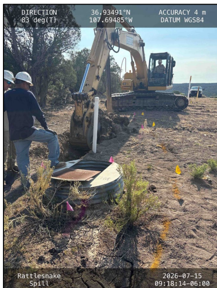
Photograph: 1 Date: 07/15/2026 Description: Excavation activities to repair pipeline.
