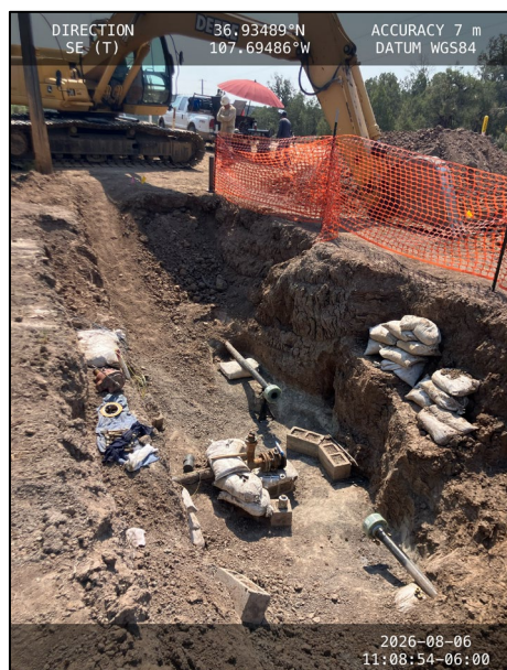
Photograph: 7 Date: 08/06/2026 Description: Final excavation extent.
