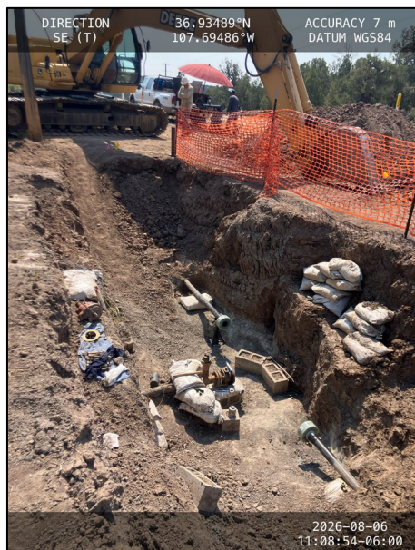
Photograph: 7 Date: 08/06/2026 Description: Final excavation extent.
