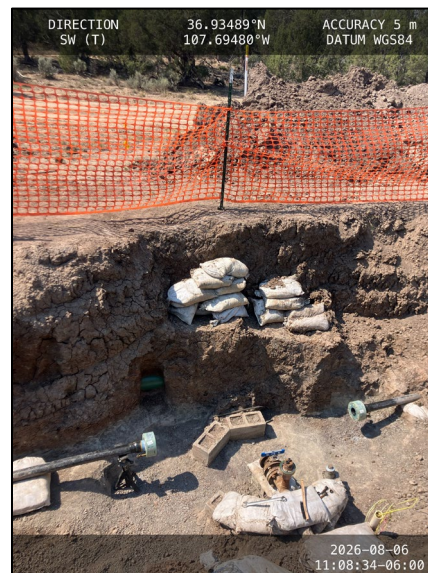
Photograph: 6 Date: 08/06/2026 Description: Excavation and exposed pipelines.
