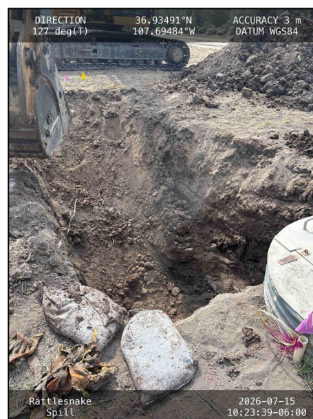
Photograph: 4 Date: 07/15/2026 Description: Excavation extent.
