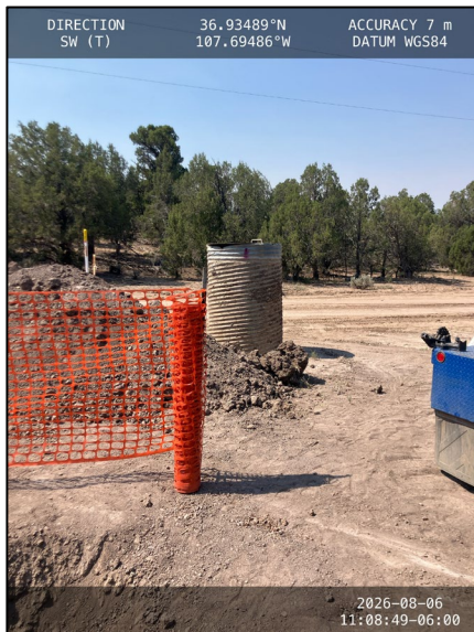
Photograph: 5 Date: 08/06/2026 Description: Underground pipeline access cellar removal.
