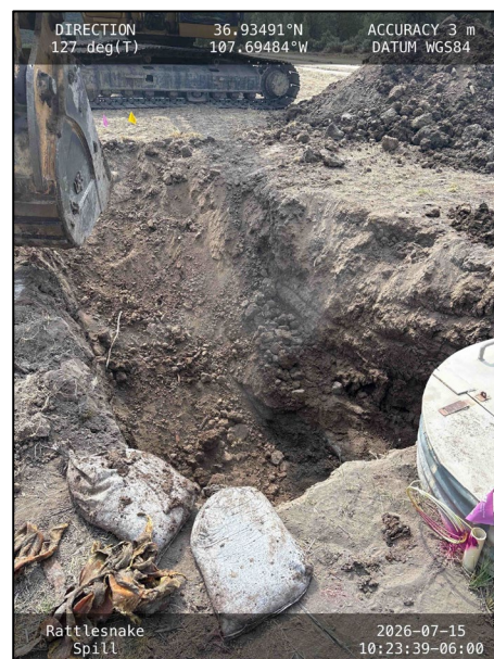
Photograph: 4 Date: 07/15/2026 Description: Excavation extent.
