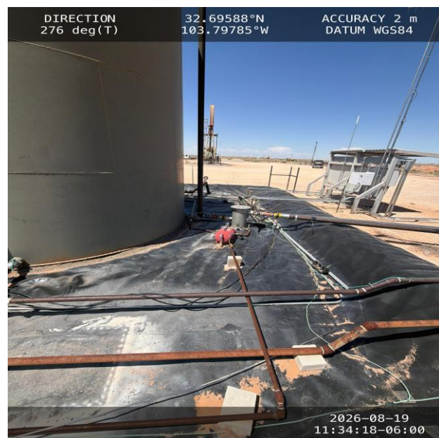
Photo 8 View of the liner corner in secondary containment area facing west.
