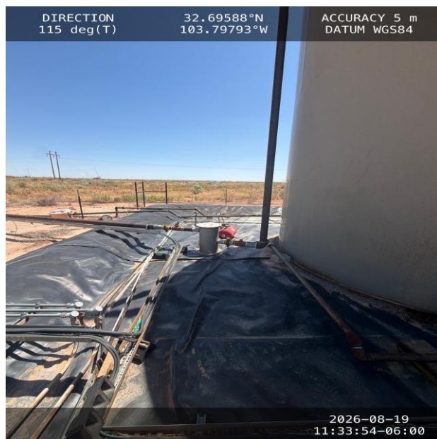
Photo 1 View of the liner corner of the containment area facing east-southeast.
