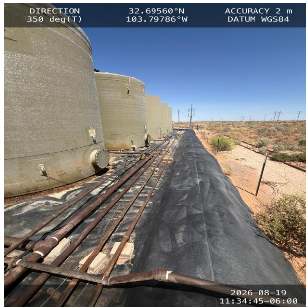
Photo 9 View of the liner along the perimeter of the tank battery secondary containment area facing north.
