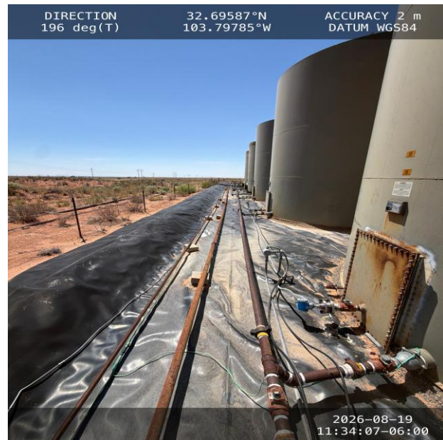
Photo 6 View of the liner along the tank battery in the secondary containment area facing south-southwest.
