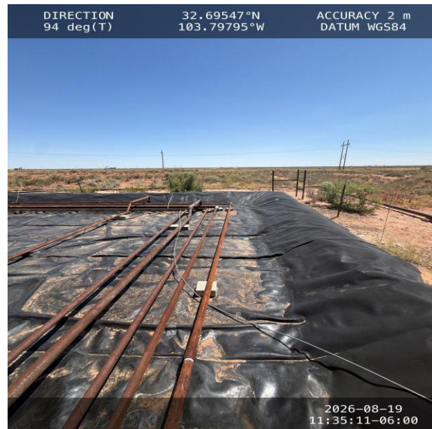
Photo 10 View of the liner with multiple aboveground pipes crossing the containment area facing east.
