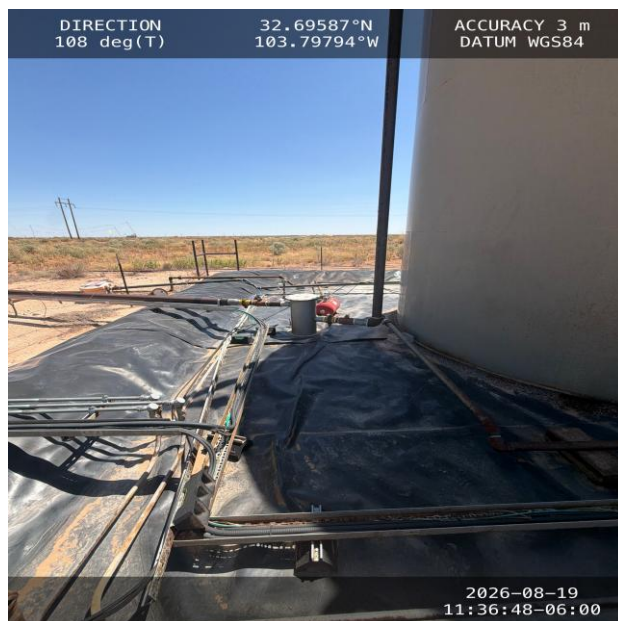
Photo 11 View of the liner in secondary containment area adjacent to a storage tank facing east-southeast.
