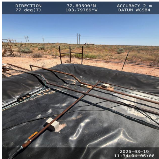
Photo 5 View of the corner of the secondary containment liner with associated piping and electrical conduits crossing the area, facing east-northeast.
