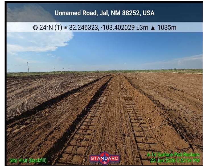
View of reclamation
