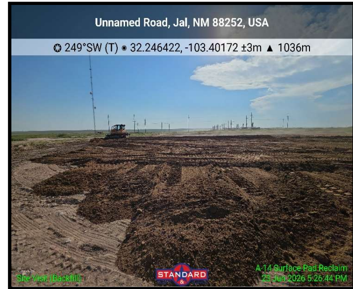
View of reclamation
