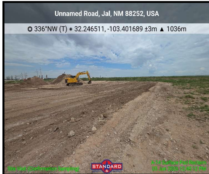
View of excavation
