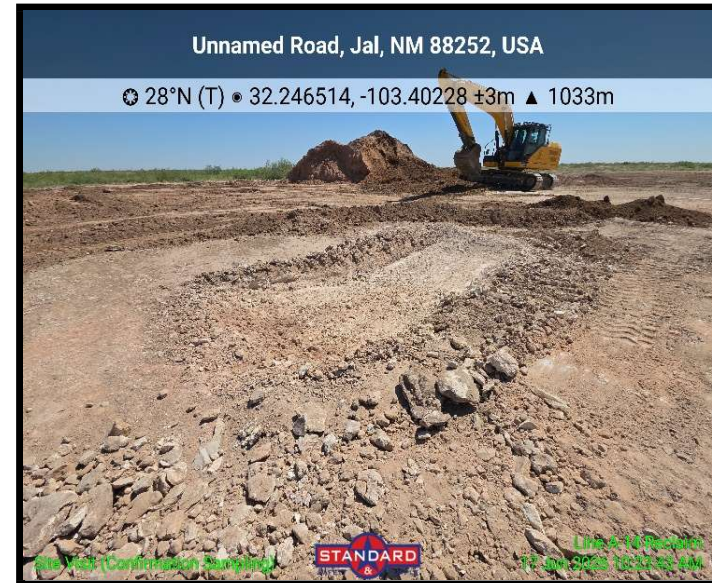
View of excavation
