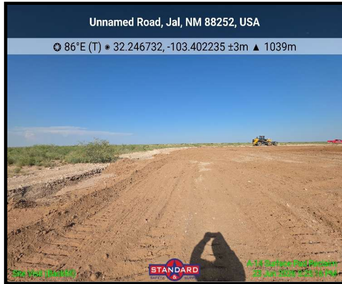
View of reclamation
