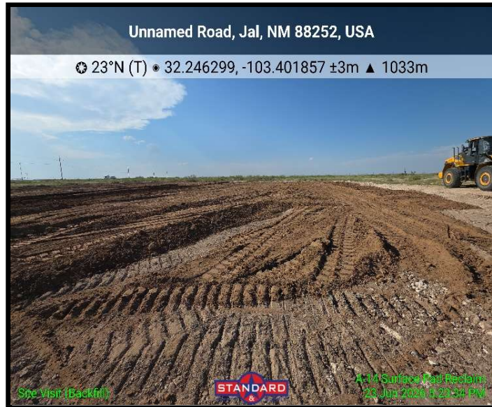
View of reclamation
