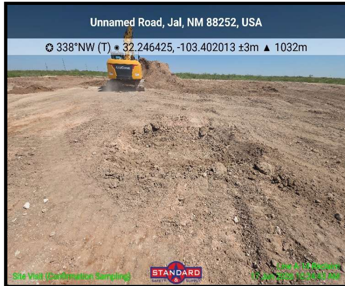
View of excavation
