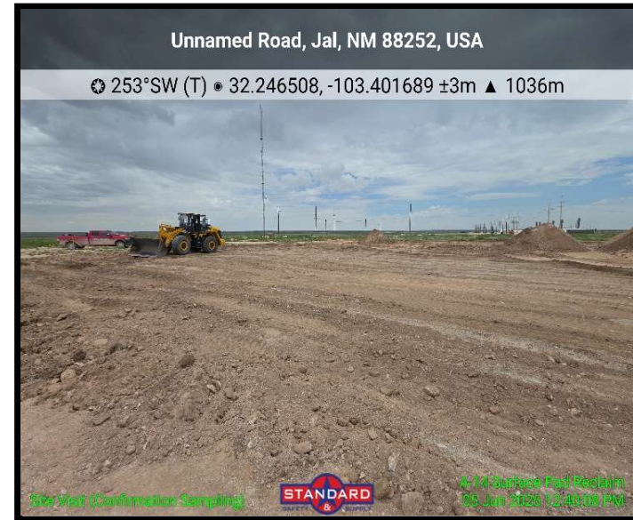
View of excavation
