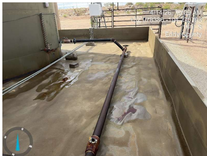
Photograph: 15 Date: 4/14/2026 Description: Liner inspection activities
