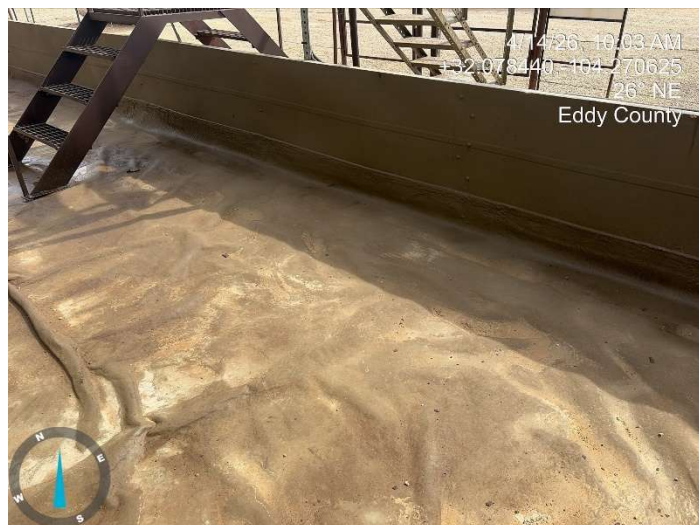
Photograph: 13 Date: 4/14/2026 Description: Liner inspection activities
