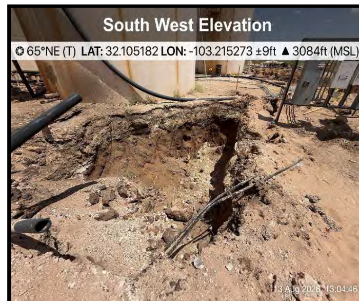
View of Excavation
