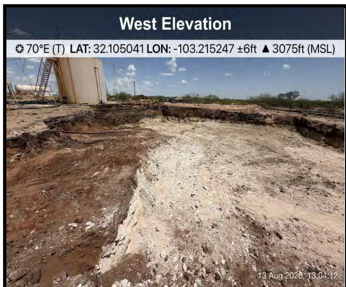
View of Excavation
