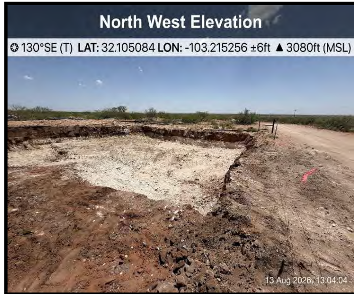
View of Excavation
