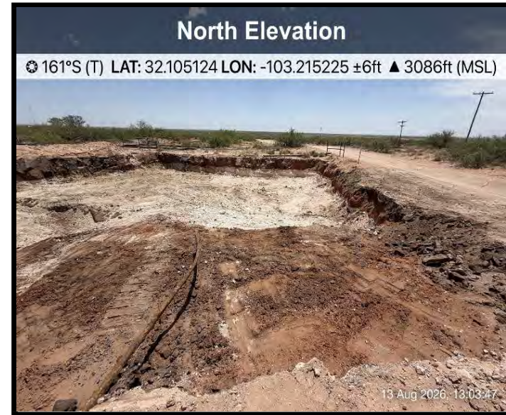
View of Excavation
